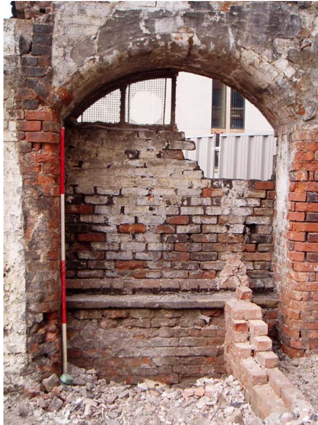
Plate 12: Blocking of window in north elevation, Bay 13
