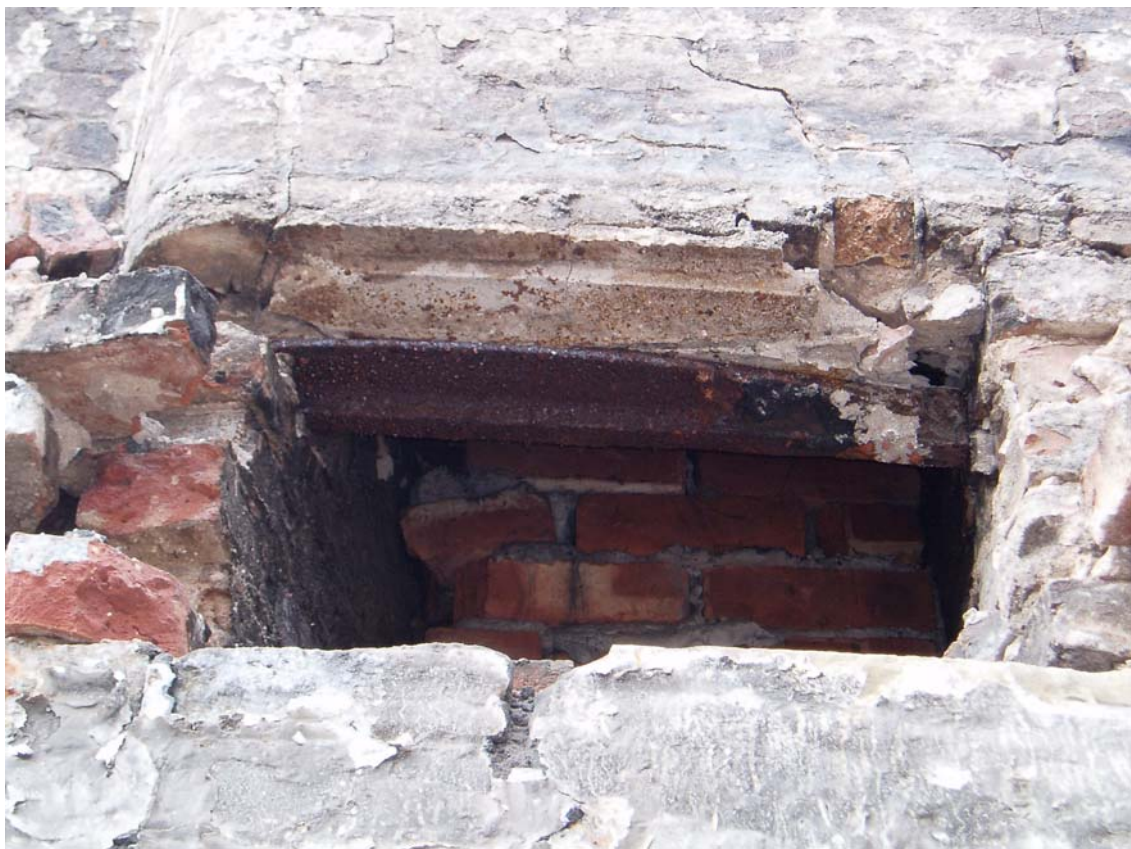
Plate 16: Detail of fish-bellied flue lintel
