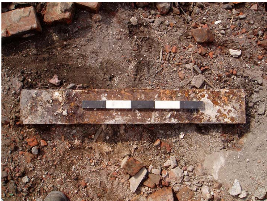
Plate 15: Detail of rectangular-section flue lintel
