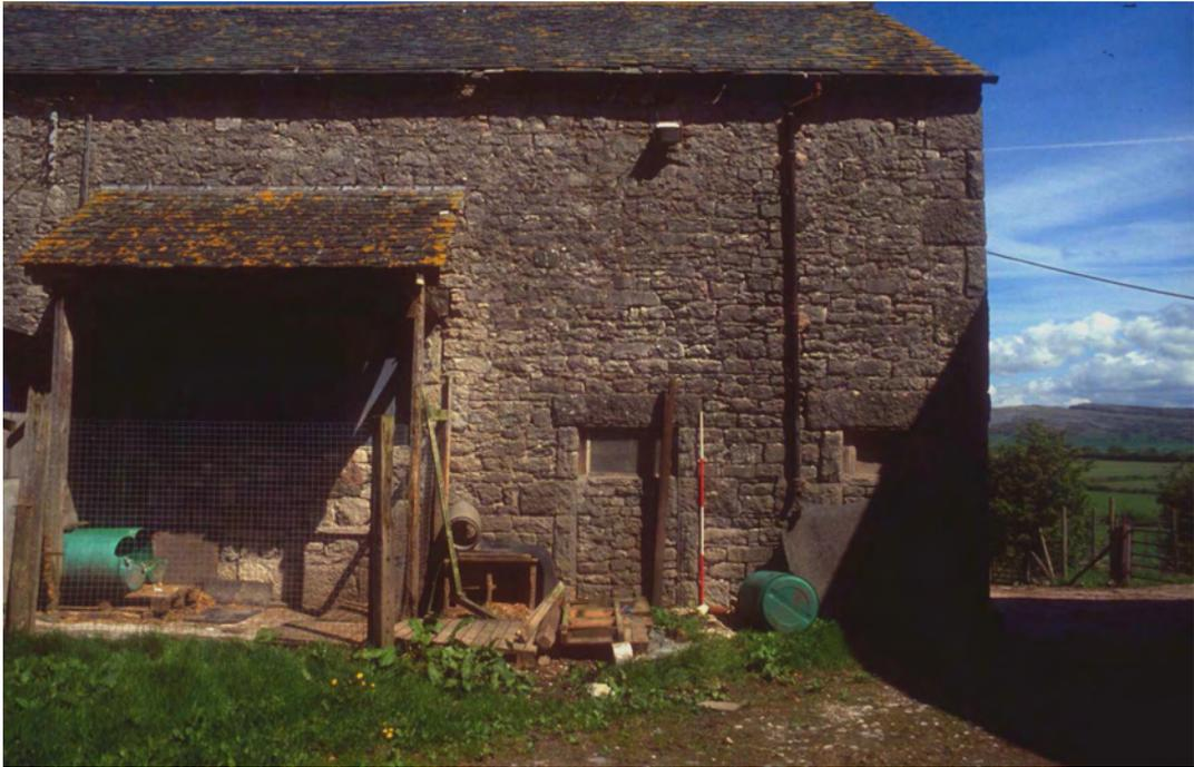
Plate 3: Detail of the porch and blocked doors at the south end of the west elevation.
