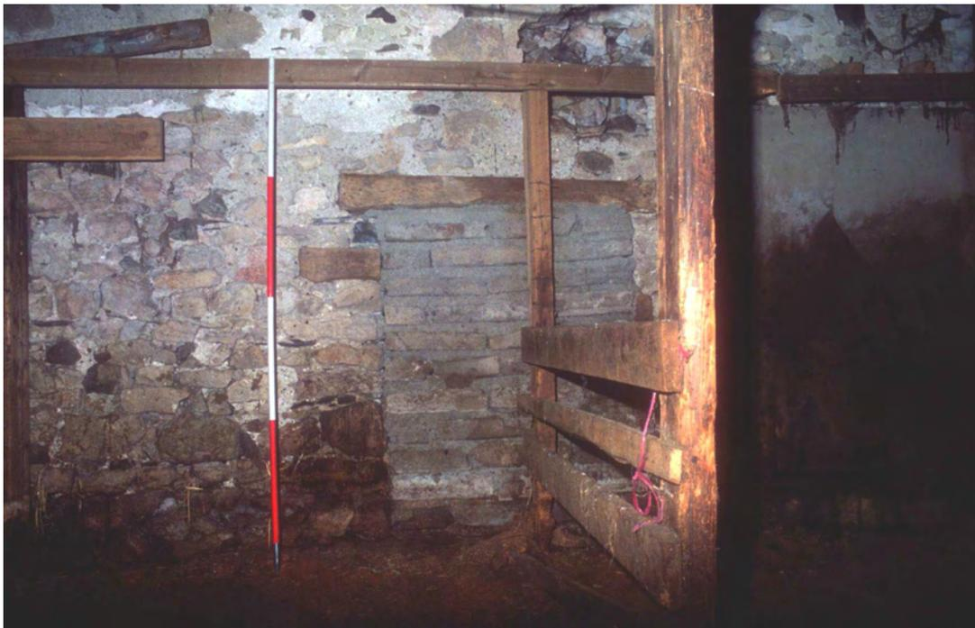
Plate 4: Detail of the stalls and one of the blocked doors on the east elevation.
