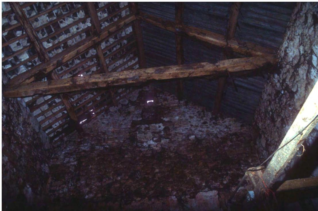
Plate 2: Detail of the most northerly truss within the barn.
