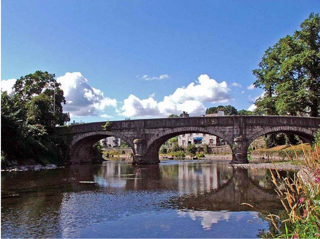
Plate 1: General view of the north side of Miller Bridge
