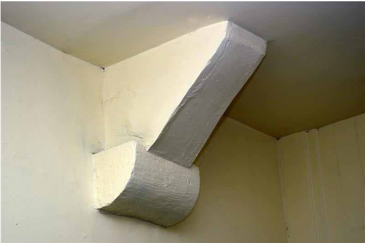
Plate 84: Corbel and base of truss in Room U102 of the Sound Archive
