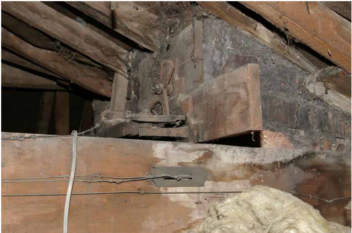
Plate 62: Communication pulleys
