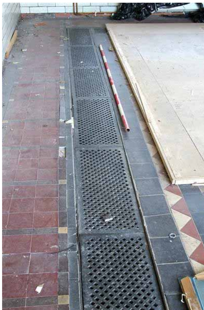
Plate 92: Heating grille in the floor of Room U107 of the Court House
