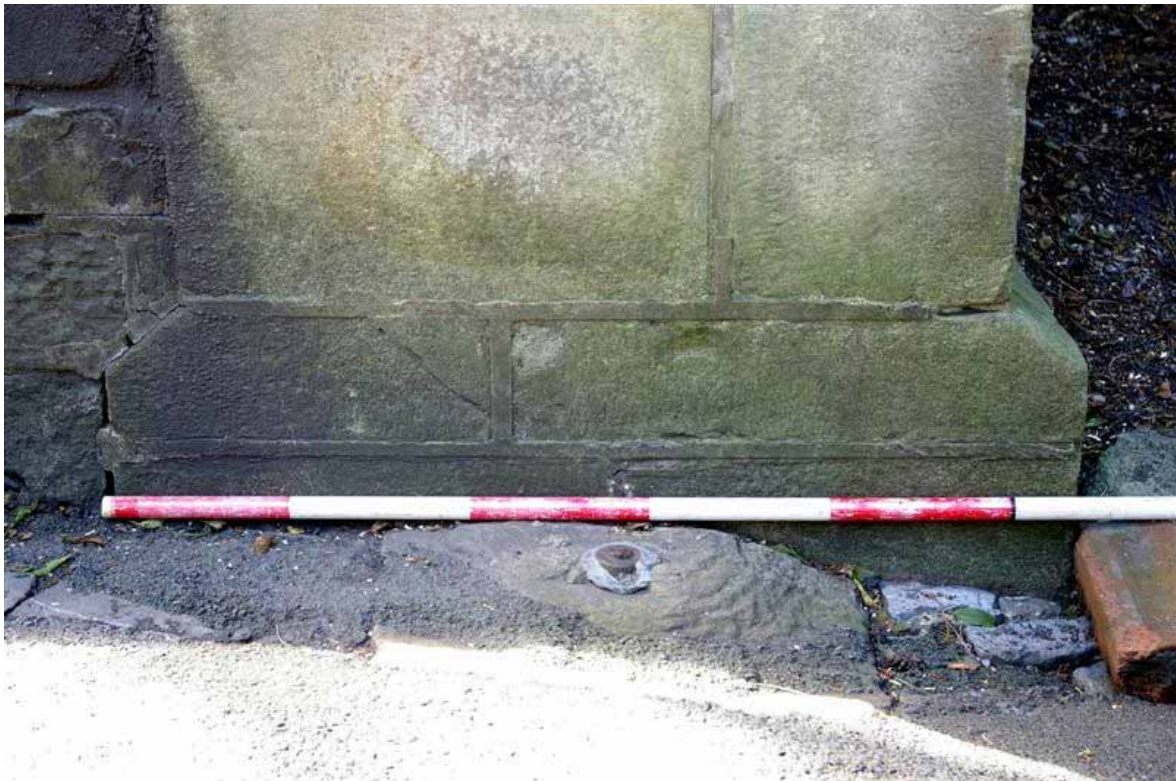
Plate 100: Example of the plinth at the base of the post, together with remnant of the gate hinges
