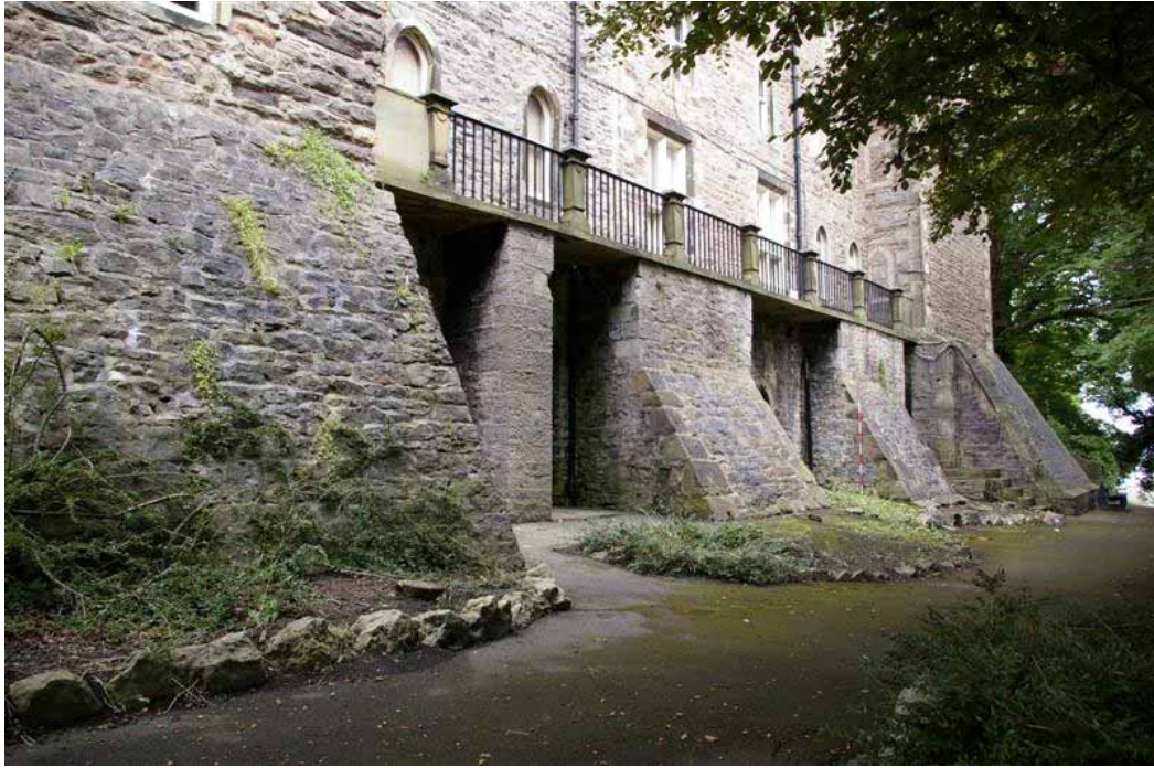
Plate 7: Buttresses and balcony at the base of the south-east elevation of the Museum
