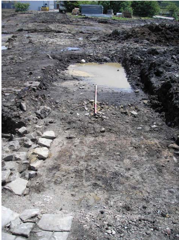
Plate 7: Wall 105 in Trench 4, looking south-east
