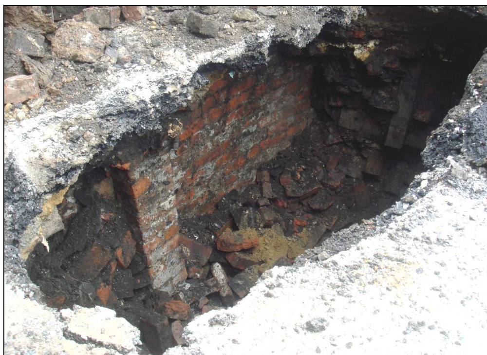
Plate 8: historic fabric revealed in the north-east-facing section of Trial Pit 1
