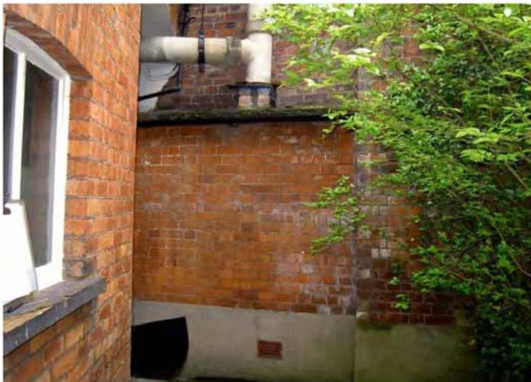
Plate 11: Junction of the main house (Phase 3) and earlier walling (Phase 2). The blocked arched aperture in the north return of the south-facing elevation is just visible below the pipe
