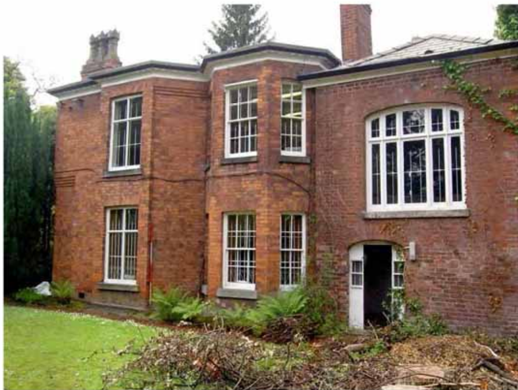
Plate 8: East-facing external elevation, showing the bay windows and raised height of the north-east end
