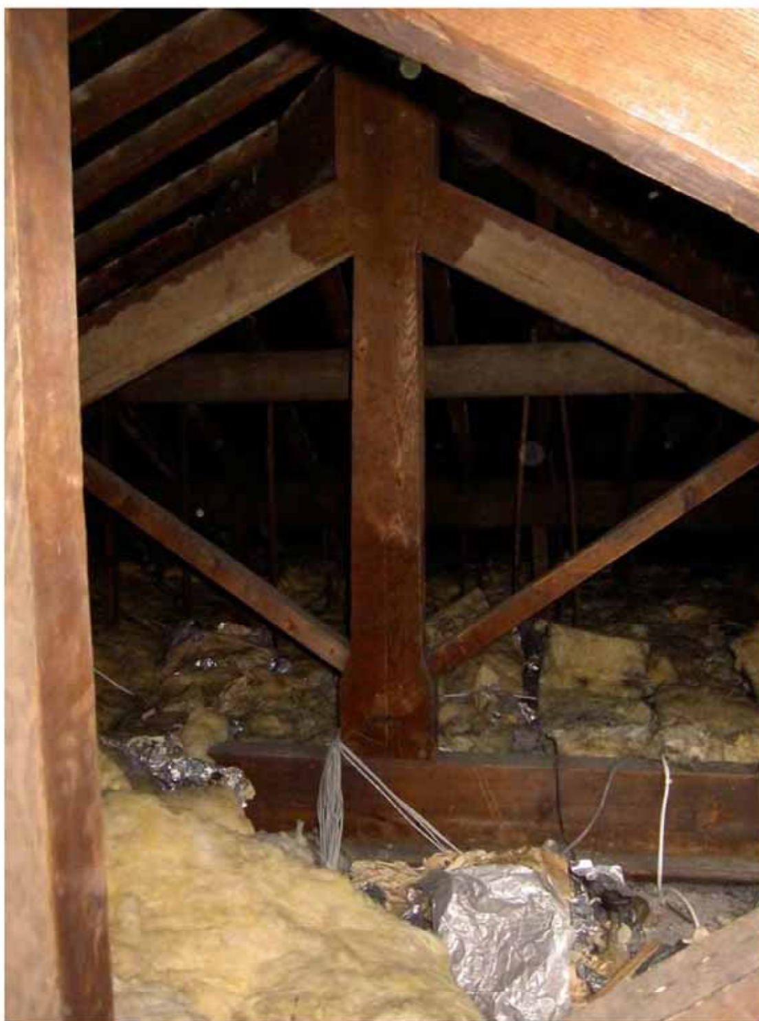
Plate 31: King-post truss in the roof space above Rooms F1-F5
