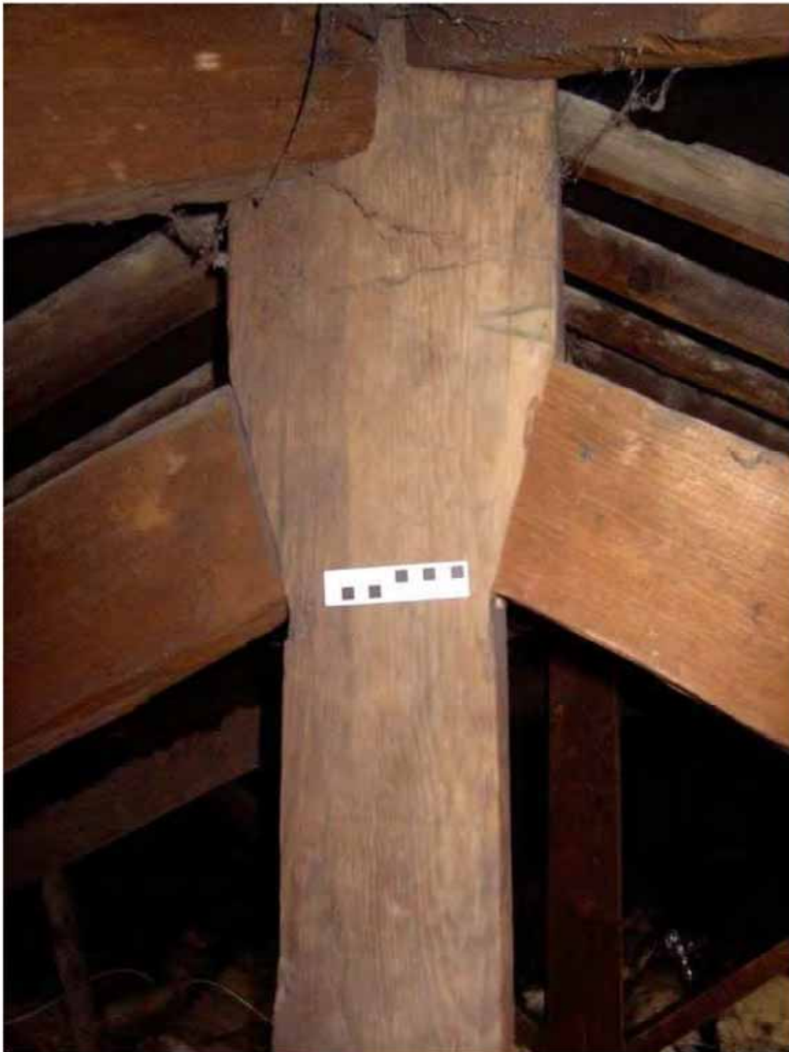
Plate 32: Baltic timber marks on one of the king post trusses
