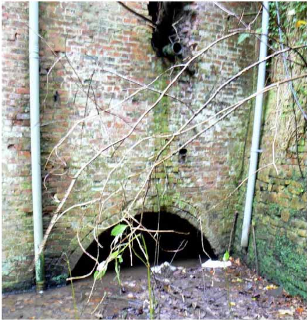
Plate 6: Brick-arched aperture at foot of north-facing elevation
