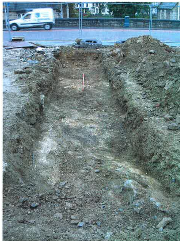
Plate 4: Post-excavation shot of Trench 1, looking east
