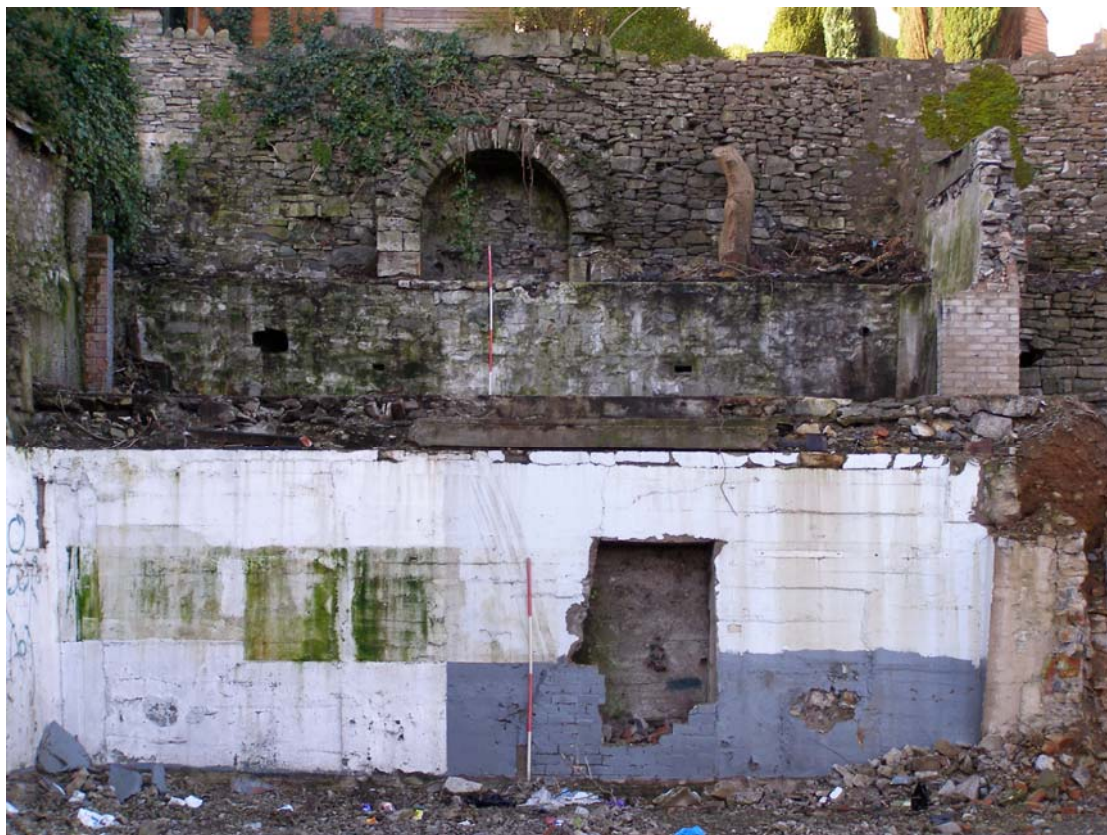
Plate 10: East-facing elevation of boundary wall, southern end
