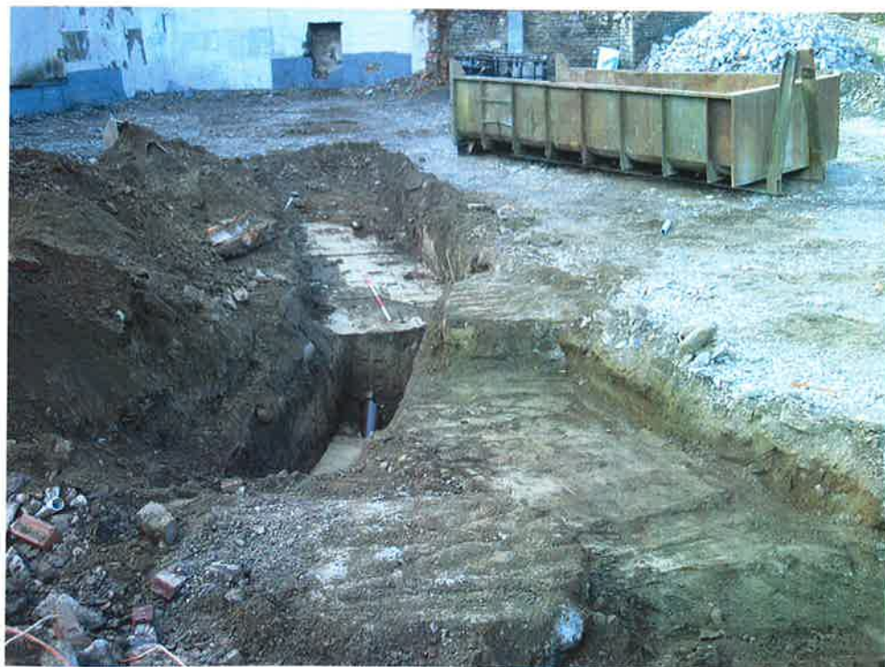
Plate 8: post-excavation shot of Trench 4, looking west
