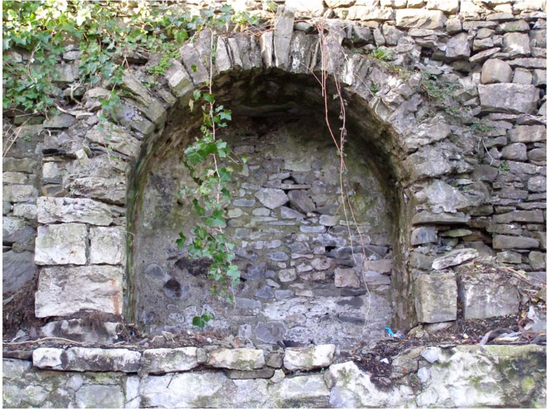
Plate 15: Detail of southern arch, east-facing elevation
