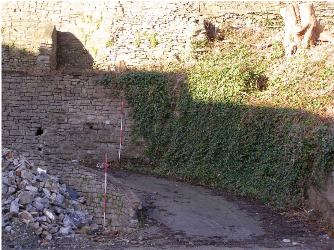
Plate 12: East-facing elevation of boundary wall, northern end
