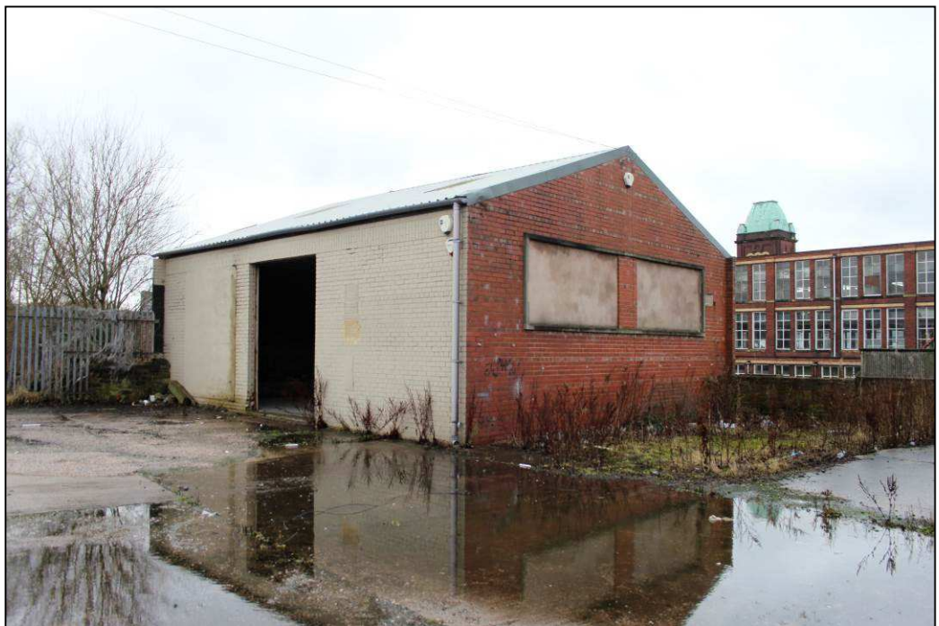
Plate 21: Late brick shed above original power plant
