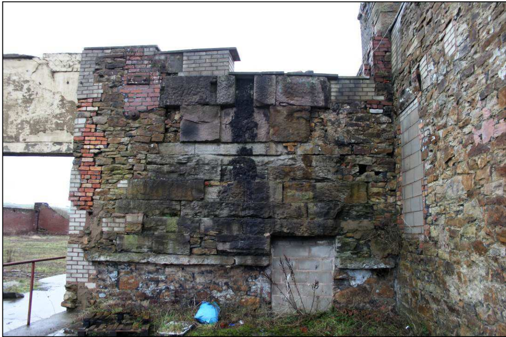
Plate 16: East wall of 1869 engine house with dressed sandstone blockwork
