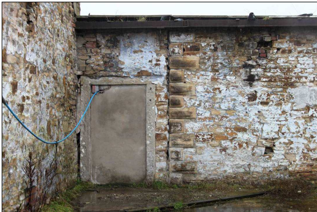
Plate 15: Quoined return of 1869 engine house with doorway in later Unit 4 extension
