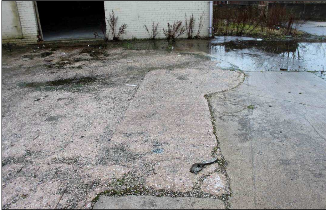
Plate 18: Joints in concrete slab denoting possible position of chimney and flue
