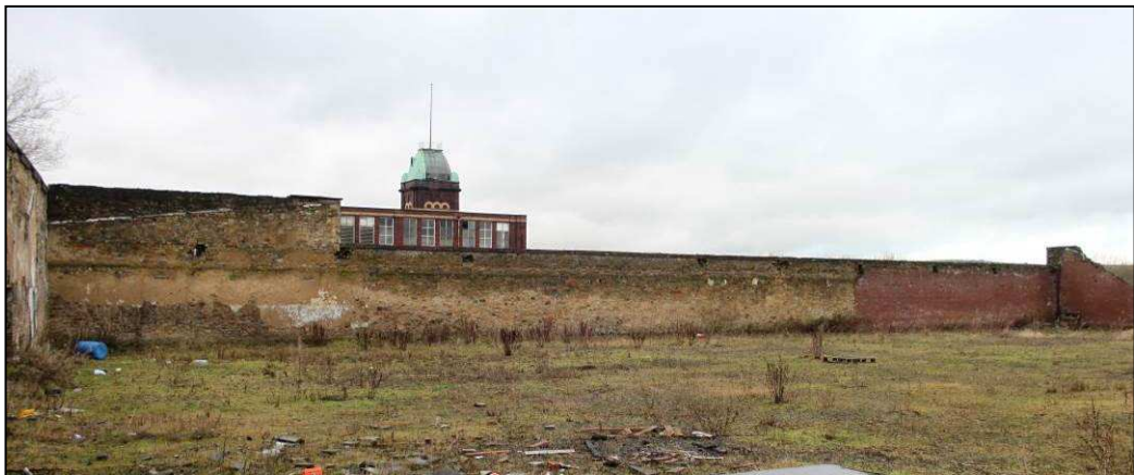
Plate 28: North internal wall of weaving shed, with extension in brick
