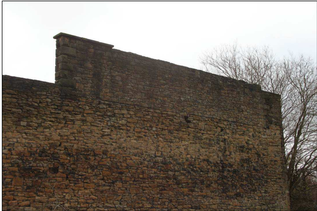
Plate 26: Rebuild at top of external north wall of weaving shed
