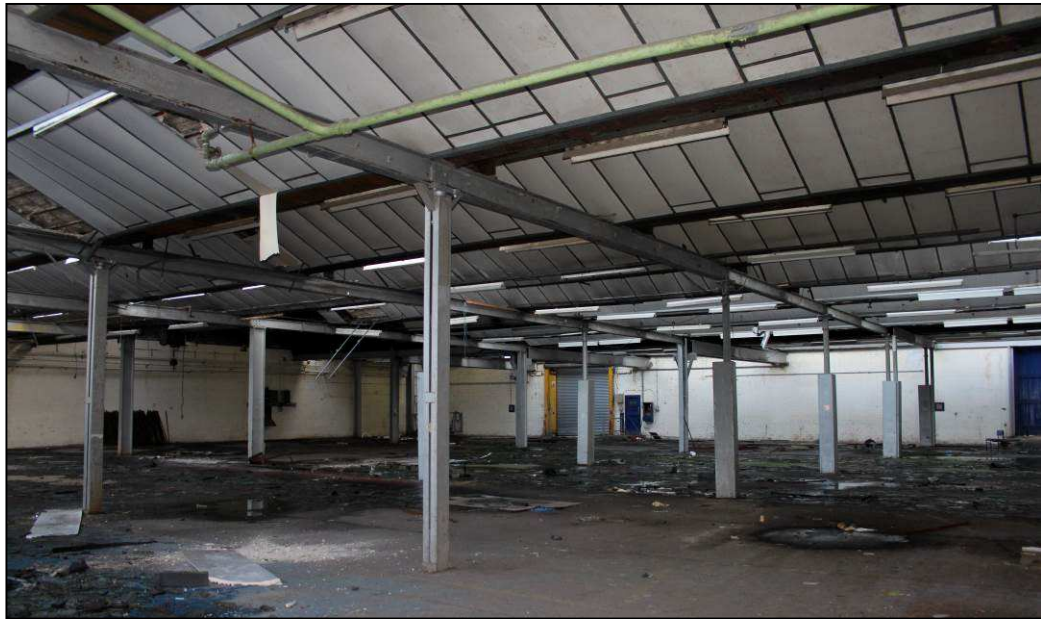
Plate 56: General view of warehouse looking south-east
