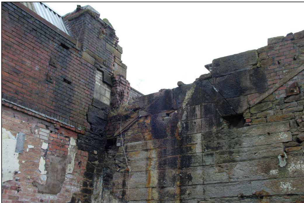
Plate 17: Upper east external elevation of 1869 engine house with bearing box position into weaving shed to left
