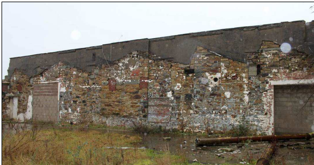
Plate 10: West external façade of spinning block with blocked tall ground-floor windows and sills for first-floor apertures
