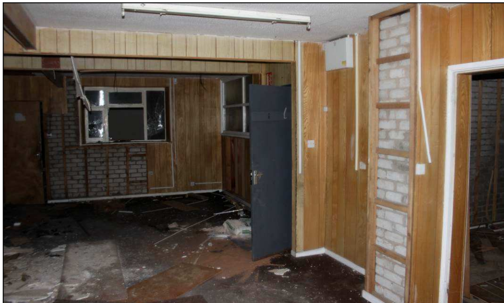
Plate 45: Remodelled interior of south-west preparation block
