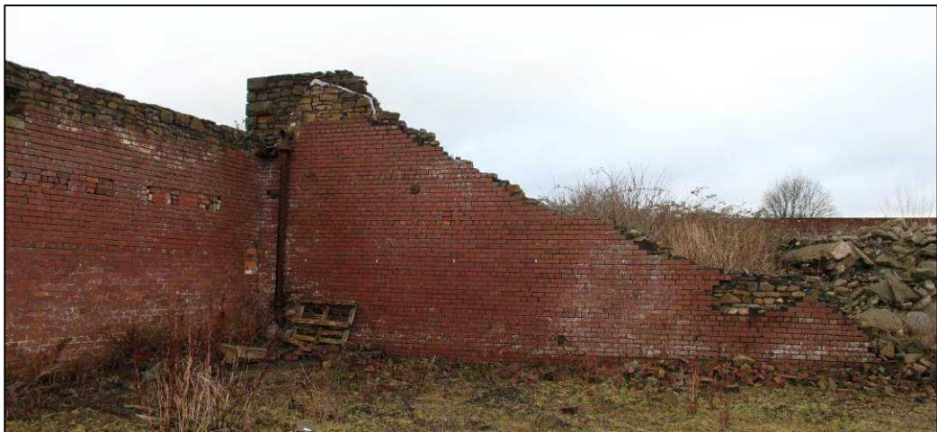
Plate 29: Brick internal facing of extension to weaving shed
