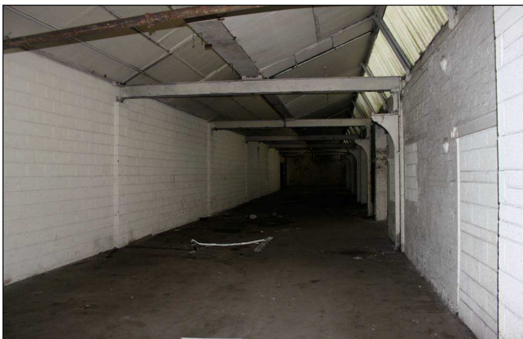
Plate 46: Northern part of Unit 9, looking west, with dividing brick wall on right and late concrete block internal partition to left
