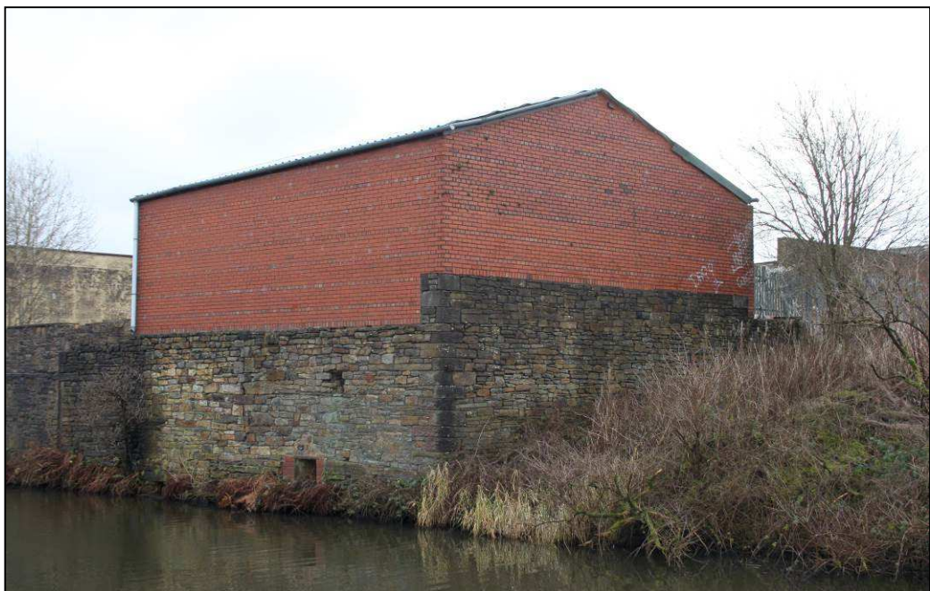
Plate 19: Boundary wall of north-west corner, with late brick shed above
