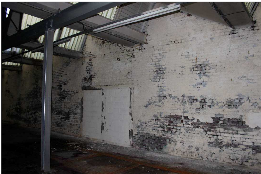
Plate 51: East wall of central warehouse with blocked double doorway
