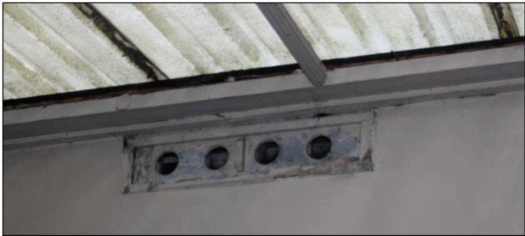
Plate 32: Timber vent in northern-light roof
