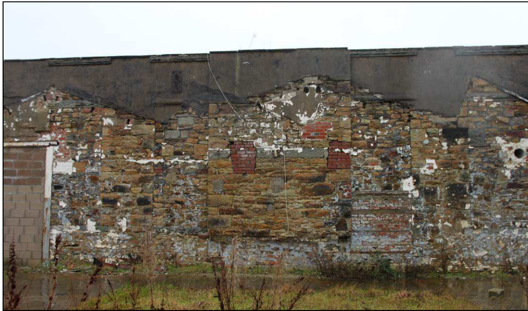
Plate 9: Projecting pilaster in centre of west external façade of original spinning block
