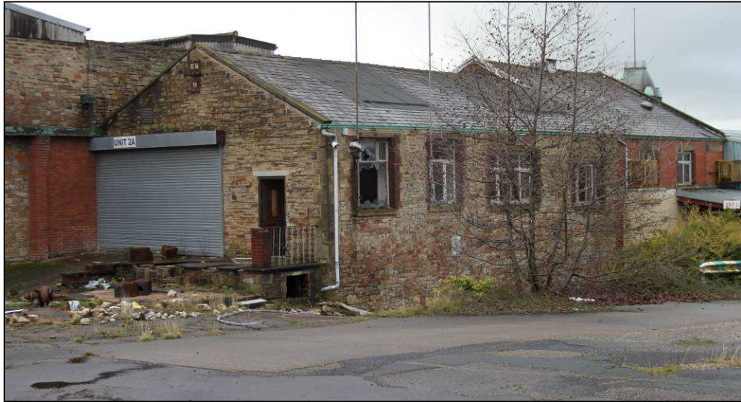
Plate 63: Loading bay, looking north-west
