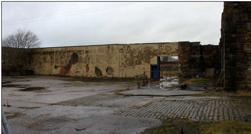
Plate 13: Concrete base denoting position of 1869 engine house with weaving shed wall to left
