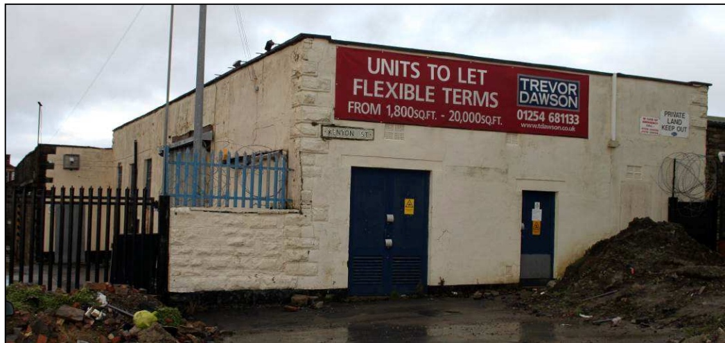
Plate 42: Kenyon Street façade of south-west preparation block
