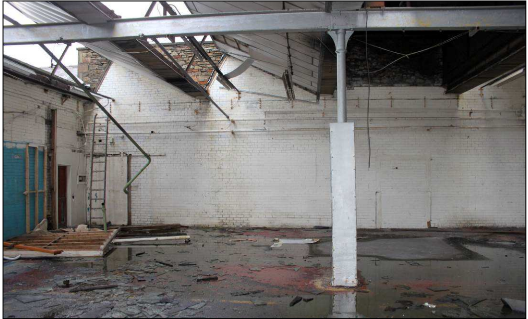
Plate 54: White-glazed brick wall of warehouse, with column detail and ceiling beam
