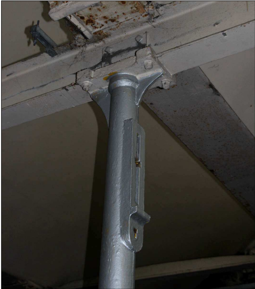
Plate 34: Column within Unit 5, looking west
