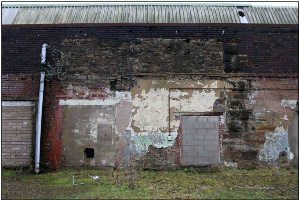
Plate 12: Quoined return of spinning block, with wall scar for first weaving shed to left
