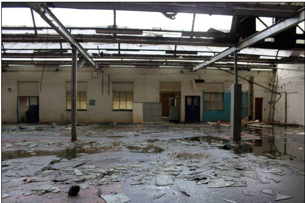
Plate 58: Windows in north elevation of warehouse
