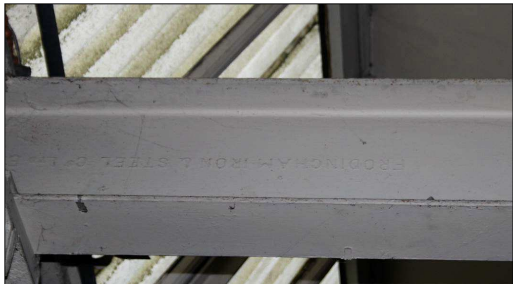
Plate 33: Rolling stamp on I-section ceiling beam
