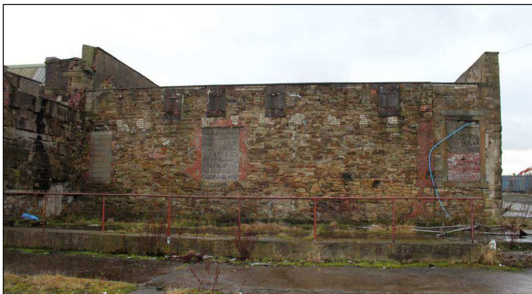
Plate 14: Raised concrete base of 1869 engine house and extant reduced south wall
