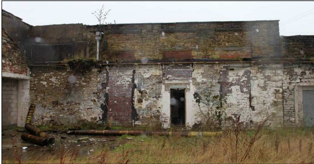
Plate 44: North wall of south-west preparation block, with first-floor window apertures at wall head
