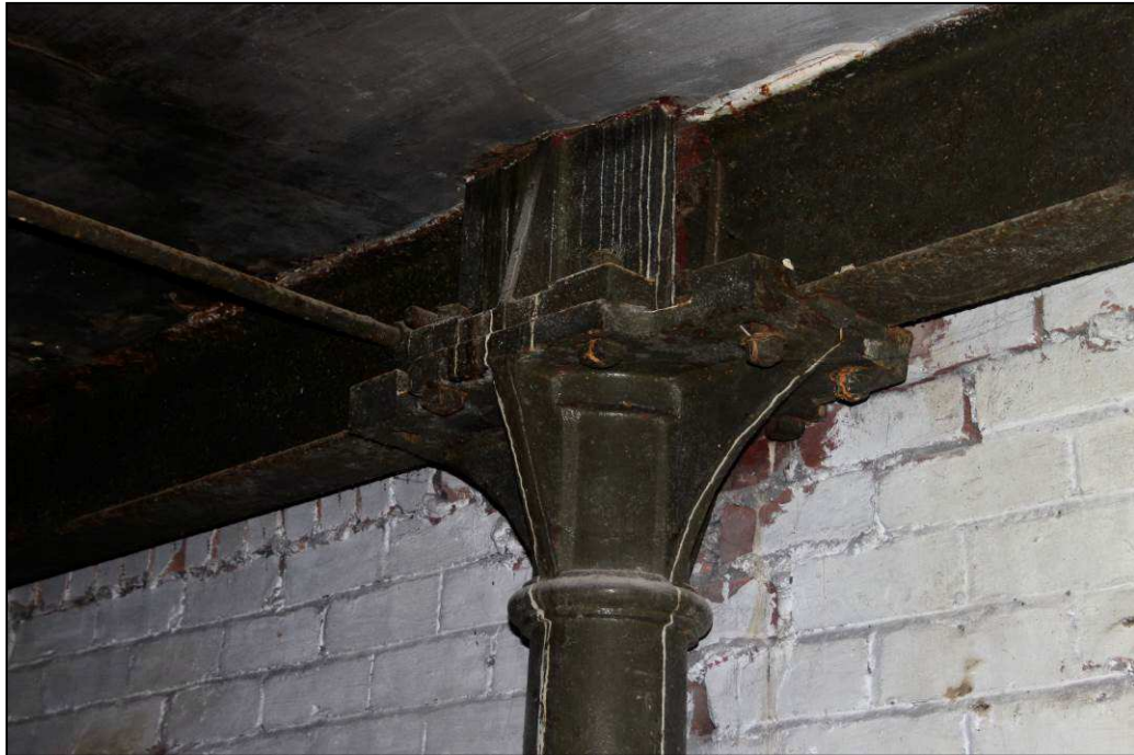
Plate 73: Detail of column capital and crush box in basement
