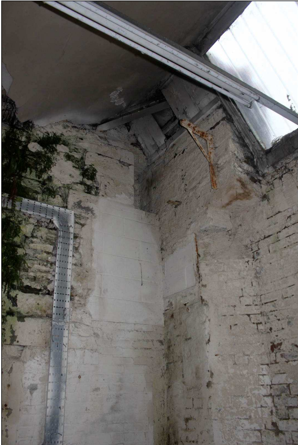
Plate 37: Angled brick pier with blocked bearing boxes, north-west corner of Unit 5
