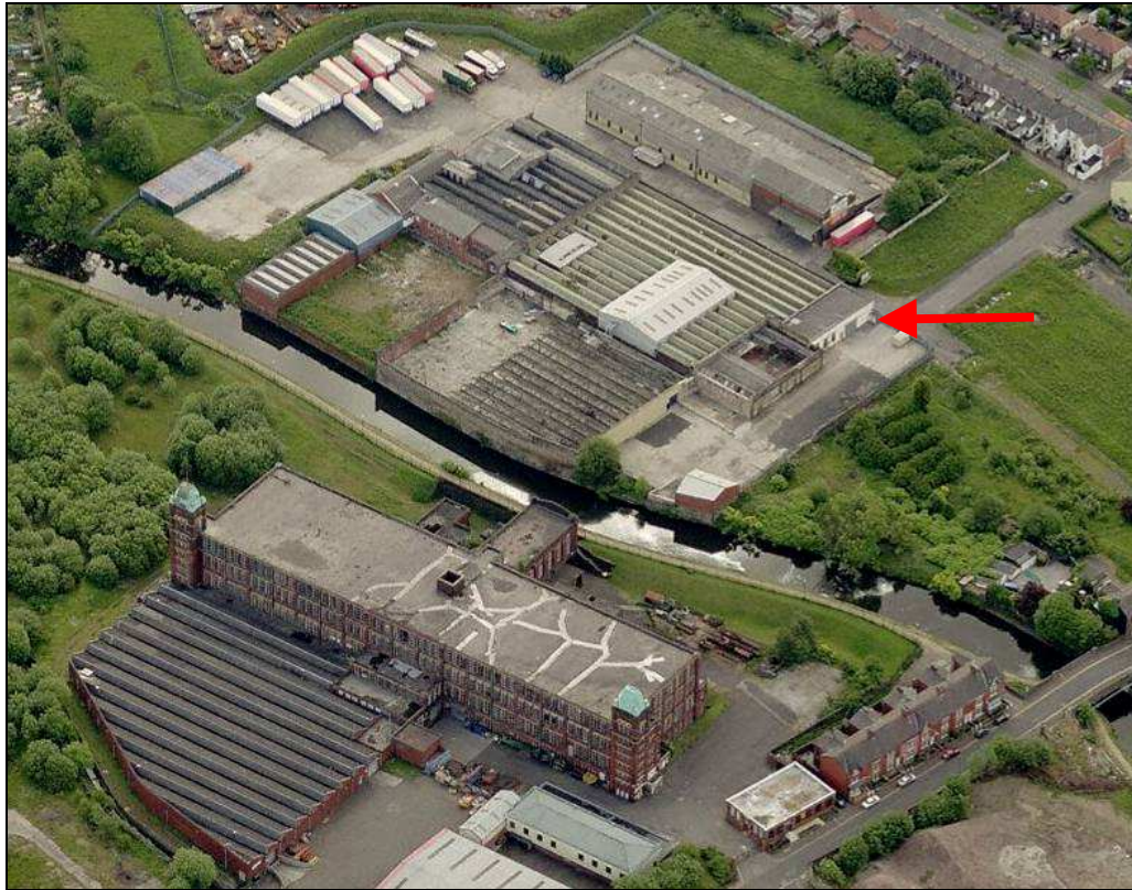
Plate 1: Recent aerial view across Hole House Mill, the canal and Imperial Mill, looking west
