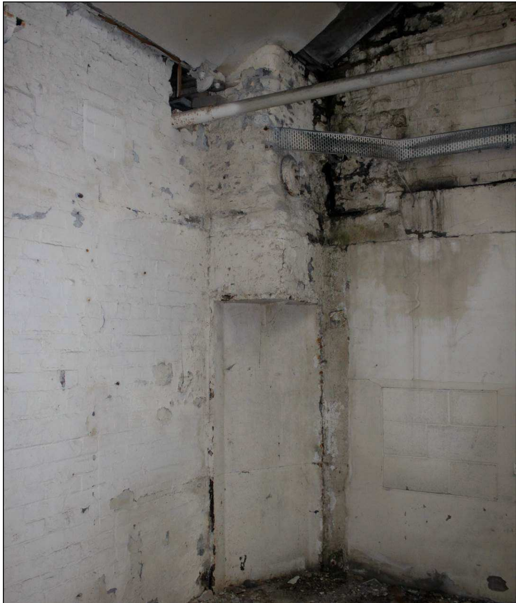
Plate 36: Cut-away angled pier in south-west corner of Unit 5
