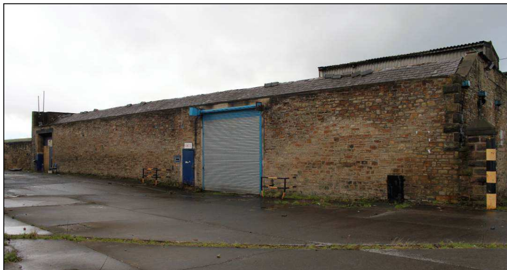
Plate 52: South elevation of Unit 3, with inserted loading door in foreground
