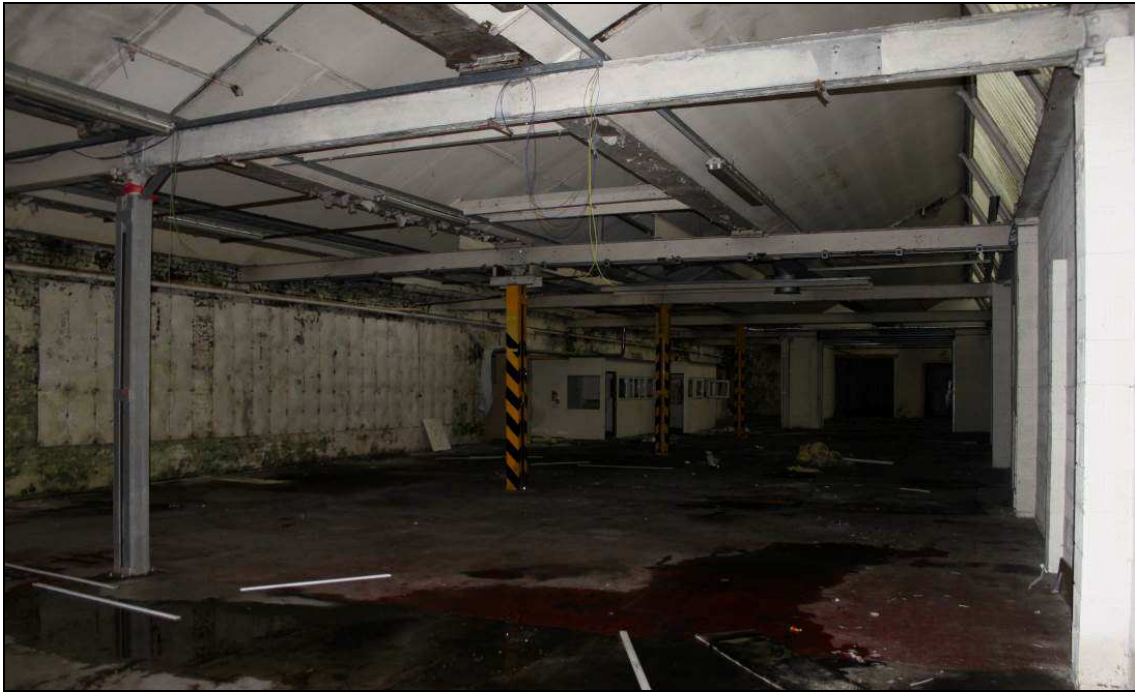
Plate 47: Southern part of preparation block, looking west
