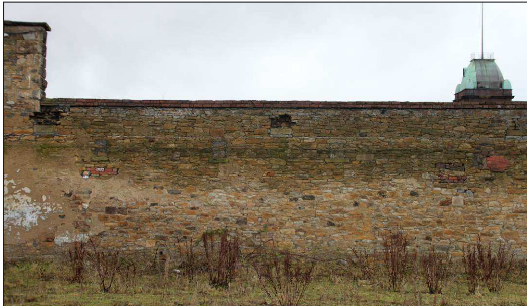
Plate 24: Detail of blocked end bearing sockets in north wall
