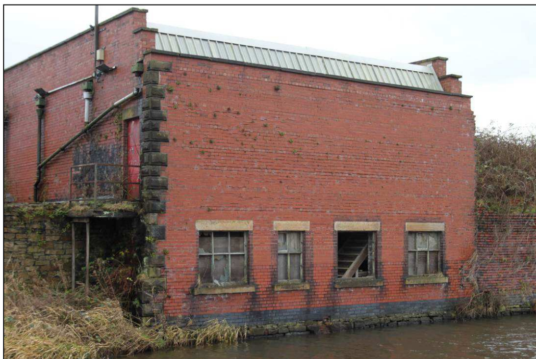
Plate 70: View of warehouse across the Leeds and Liverpool Canal, with stone-built fuse room to left
