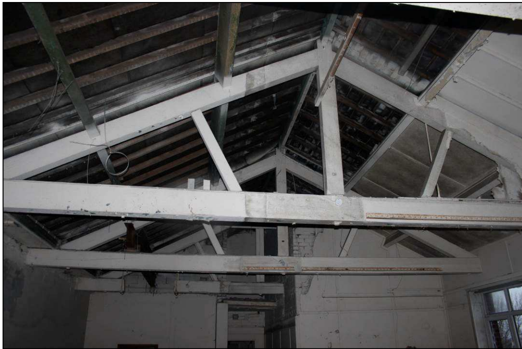
Plate 64: Trusses within loading bay
