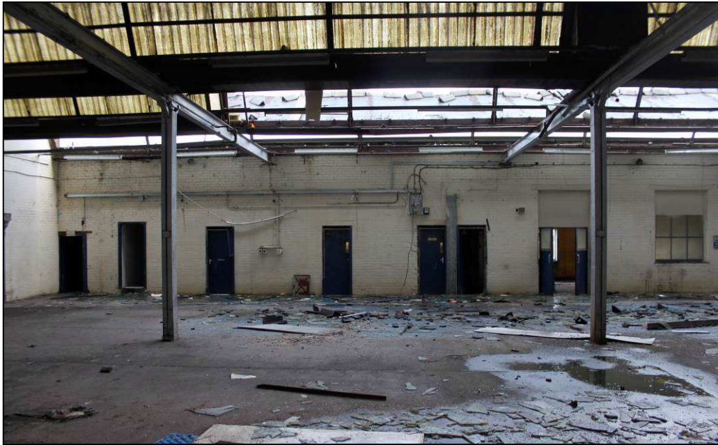
Plate 59: Privy block inserted at west side of north wall
