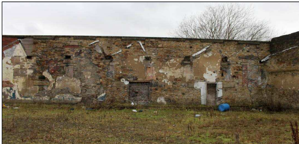
Plate 25: First floor window sills and valley gutter sockets, west wall
