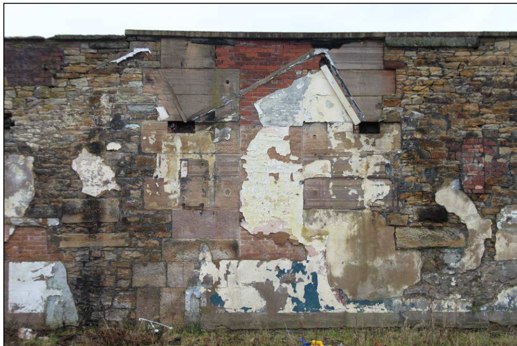
Plate 22: Ashlar blockwork of bearing for rope drum, with bolt holes and infilled wheel pit
