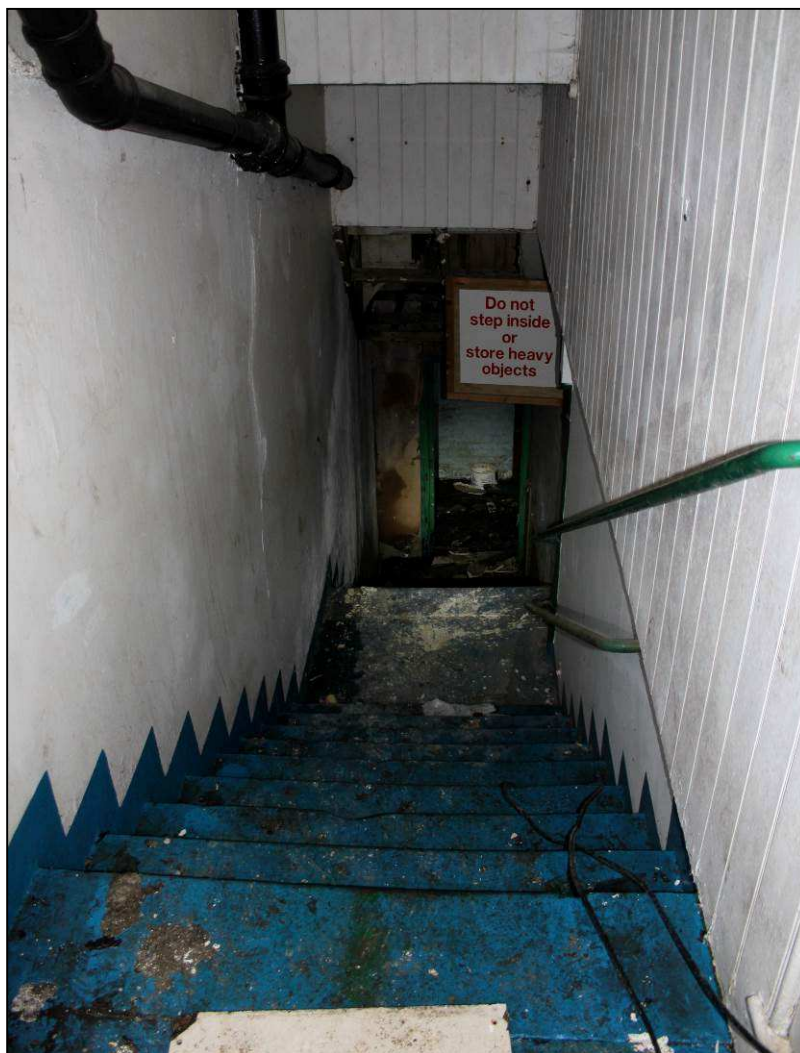
Plate 60: Stairs to open yard to north from warehouse, and to basement of Unit 8
