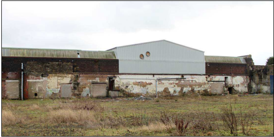
Plate 11: External stone north face of spinning block, with red brick of later weaving shed above
