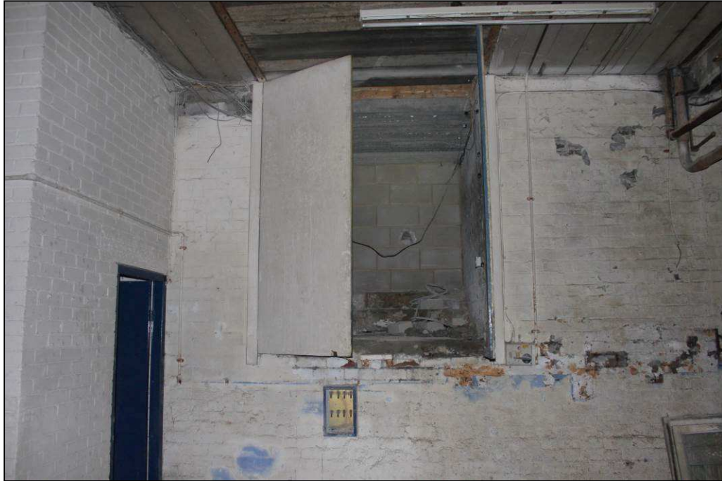
Plate 65: Hoist in north wall of loading bay
