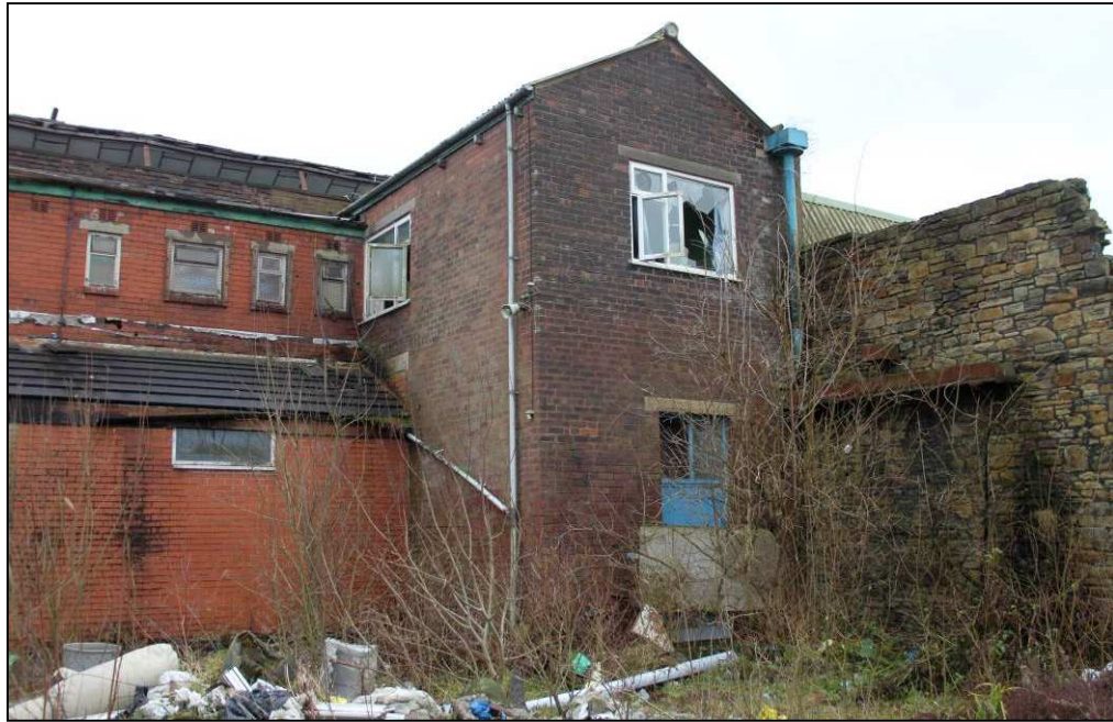
Plate 30: Two-storey tower and external gutter of weaving shed to right
