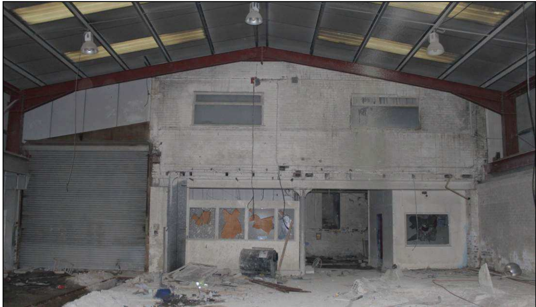
Plate 68: North wall of office block and replacement steel roof of north-east warehouse
