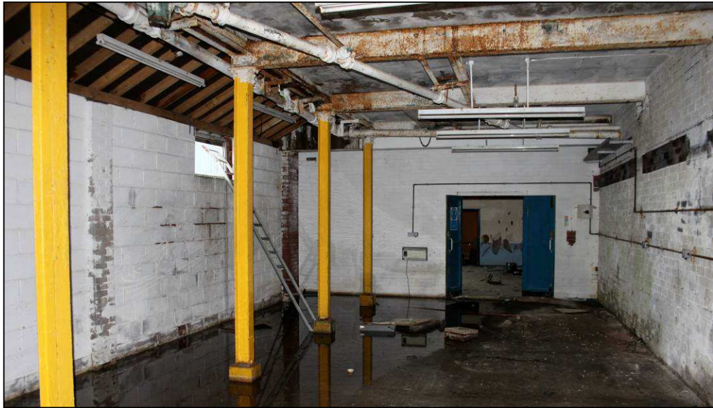
Plate 61: Extension to north of warehouse
