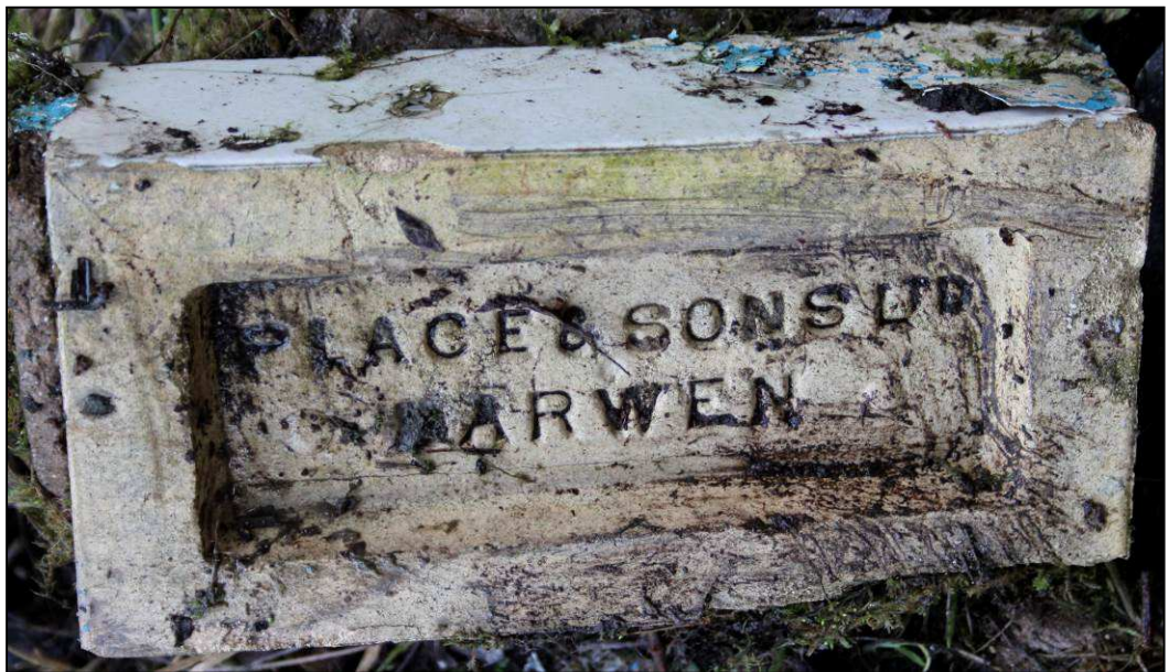
Plate 55: Frogged and stamped brick from warehouse
