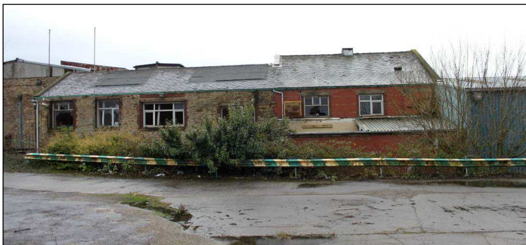
Plate 62: General view of warehouse loading bay and brick office block
