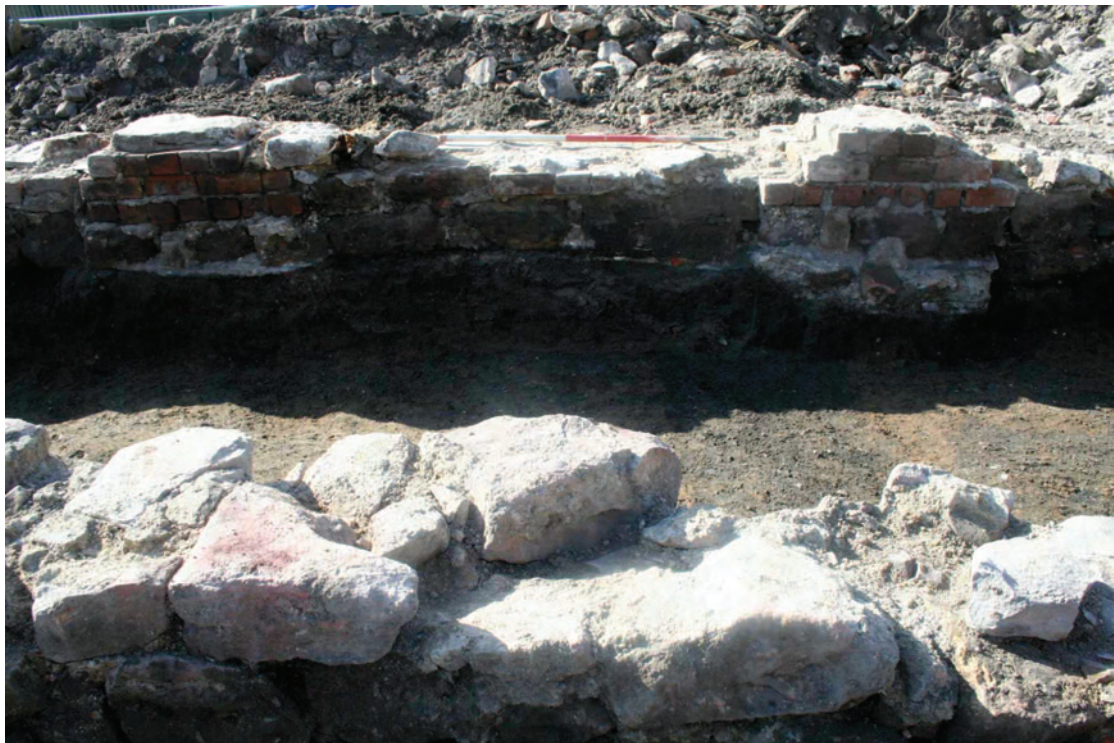
Plate 41: North-facing elevation of wall 1020 showing inserted brick column bases 1023 and 1024
