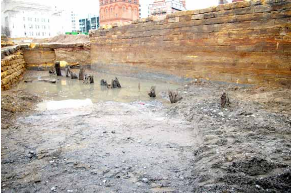
Plate 2: Sea wall 5707 , west-facing elevation, also showing timbers 7736 ; Area A
