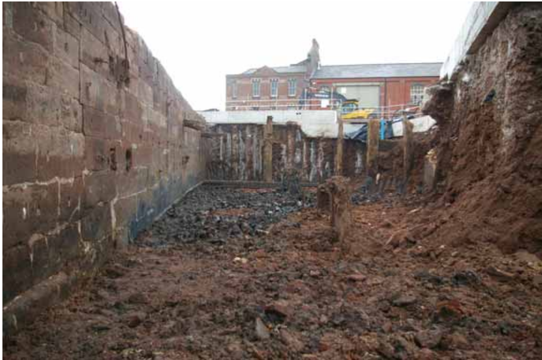
Plate 18: Interior of Manchester Dock, showing the remains of timber piers and sandstone backfill
