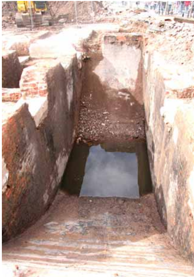
Plate 19: The Guibal-fan -style fan housing in the Pumping Station at the eastern limit of Area B
