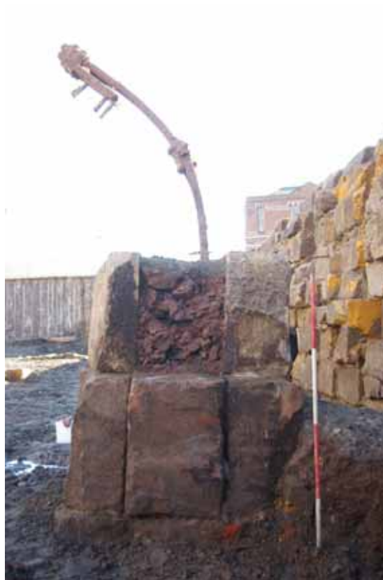
Plate 15: Crane base at the rear of Manchester Dock
