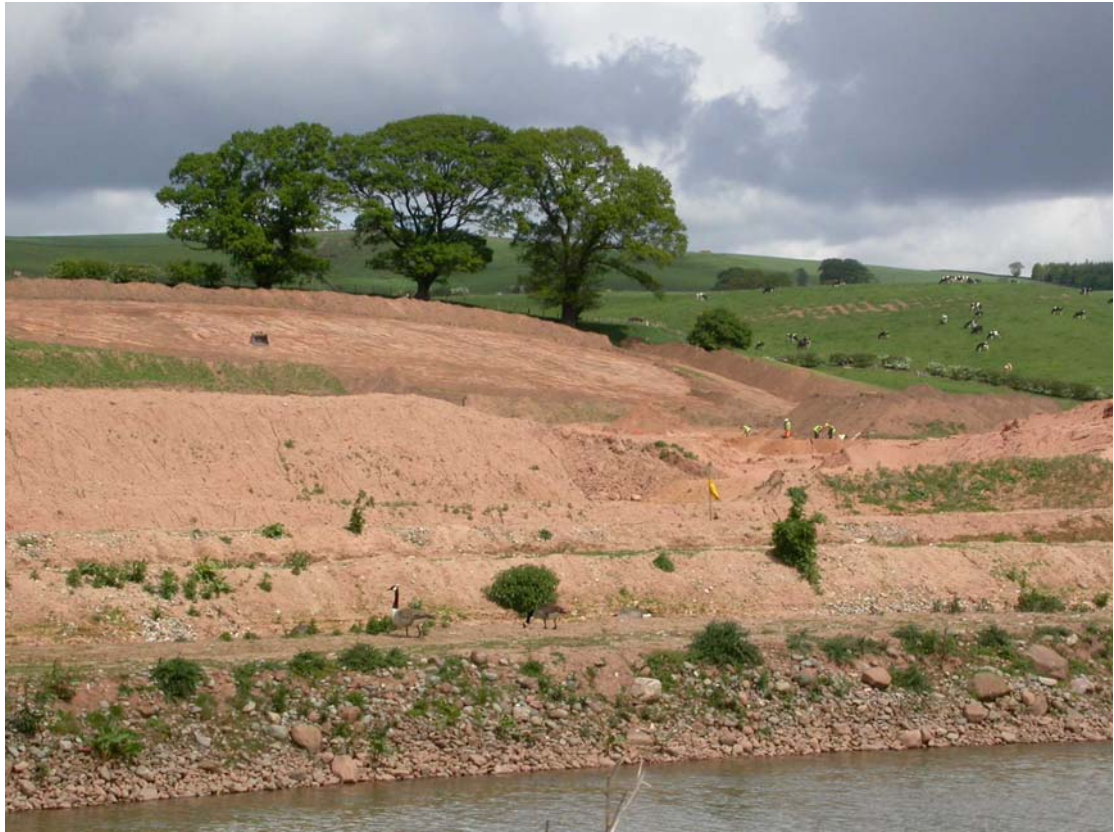
Plate 1: General view of site
