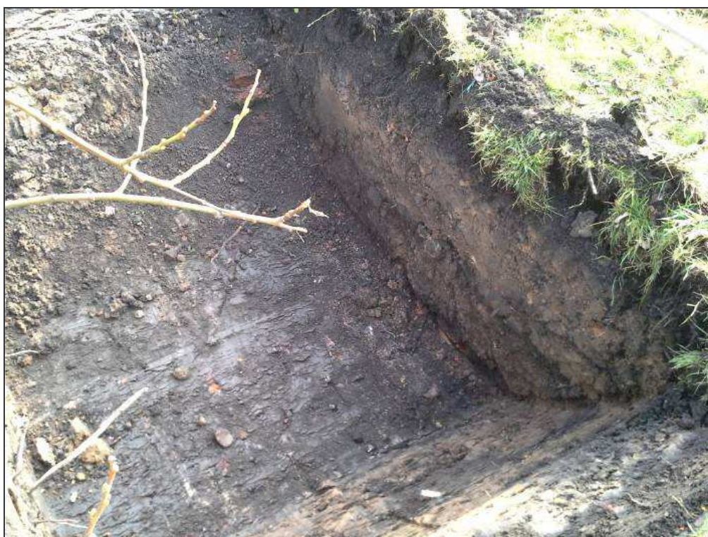
Plate 15: Trench 5 South-western part of Trench 5, with sewer infill, looking west
