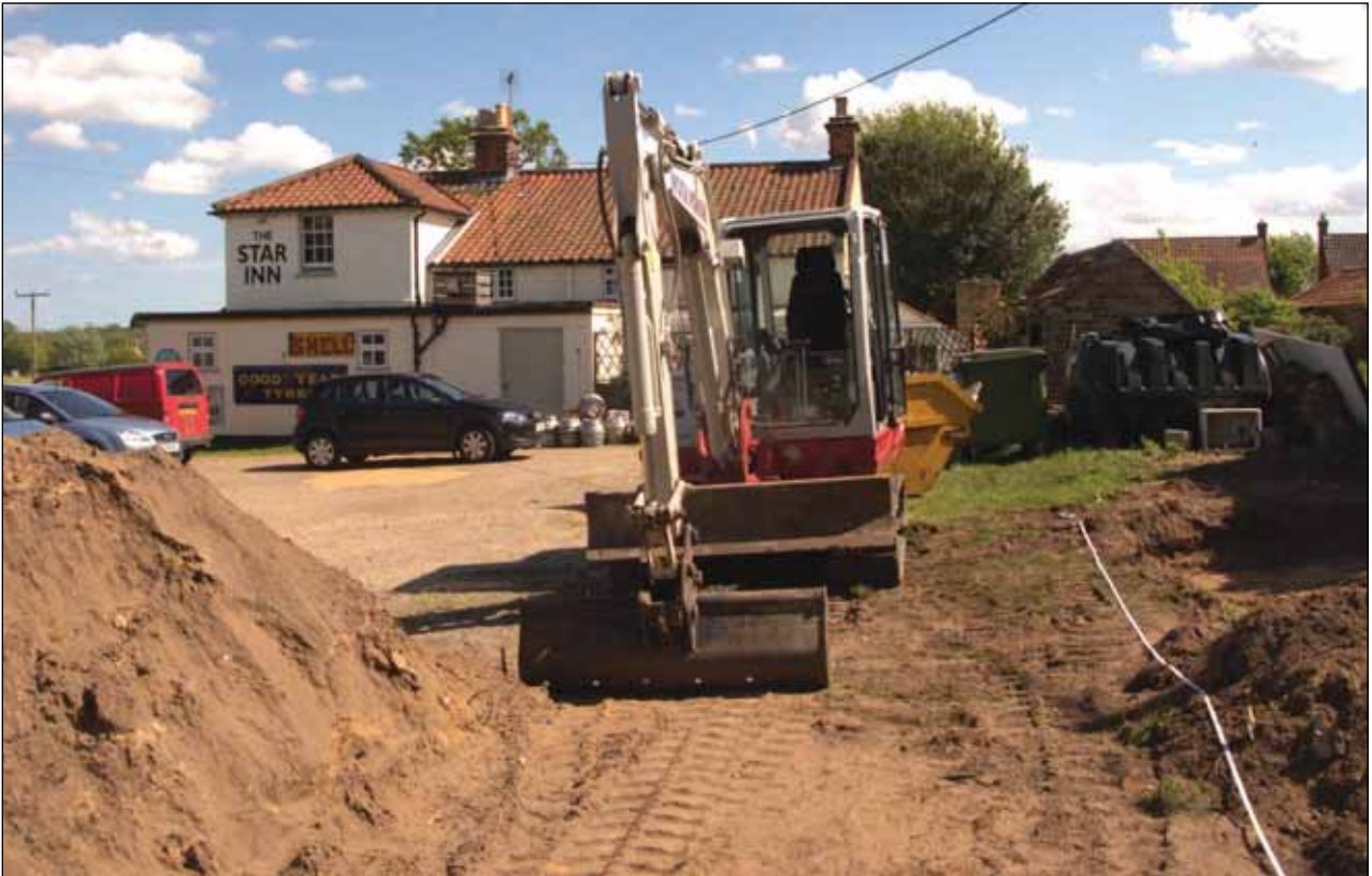
Plate 1: Working shot of the site and The Star Inn looking south
