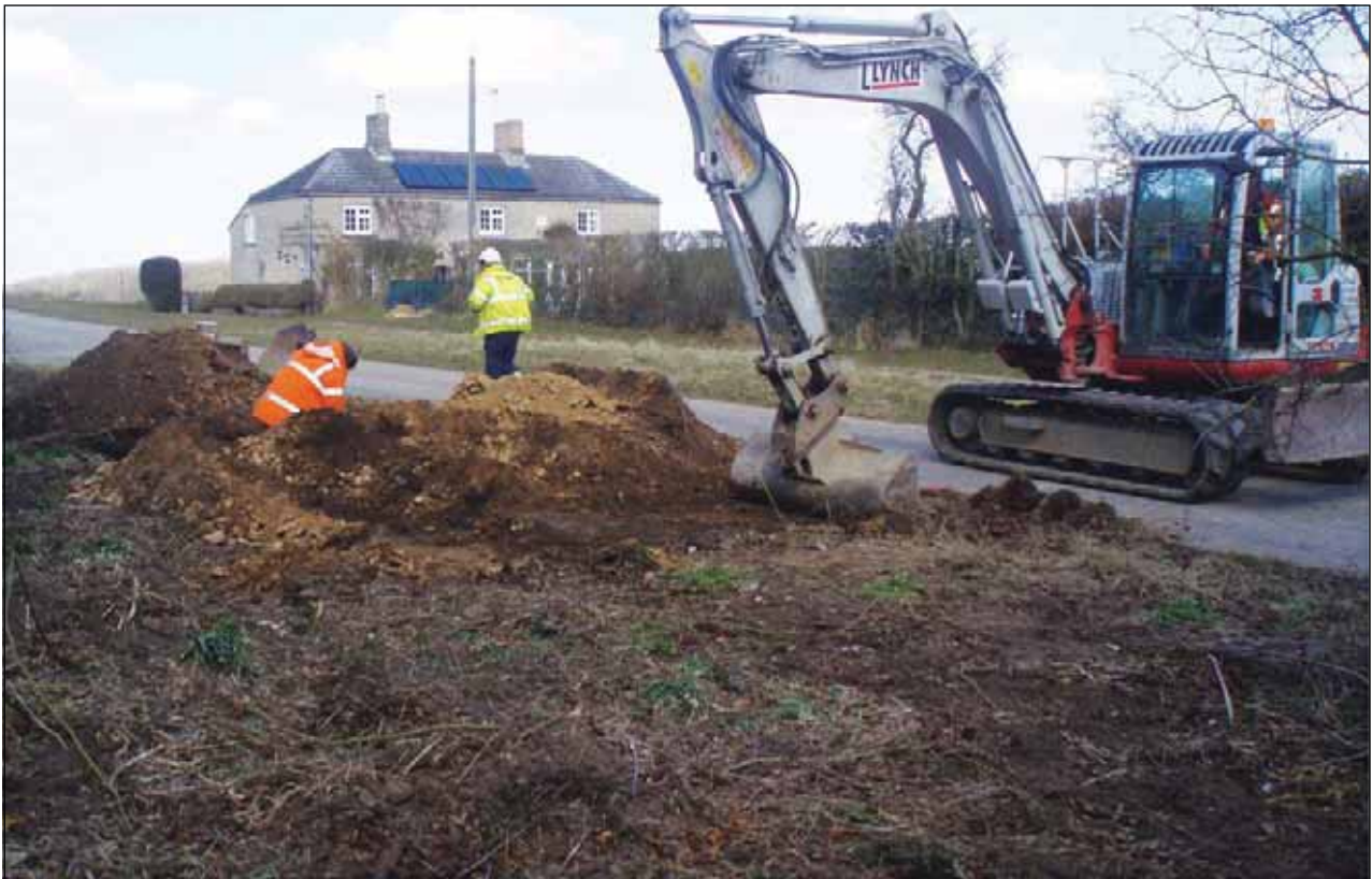
Plate 1: Trench 1 and 2 excavations
