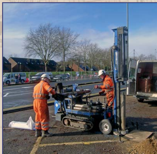
Extracting boreholes in February 2015
