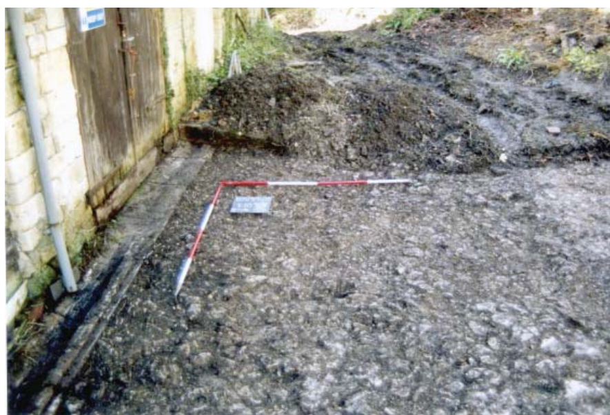
Plate 4: Trench 10 from the east showing wear in gutter in front of wagon store and quality of cobbling
