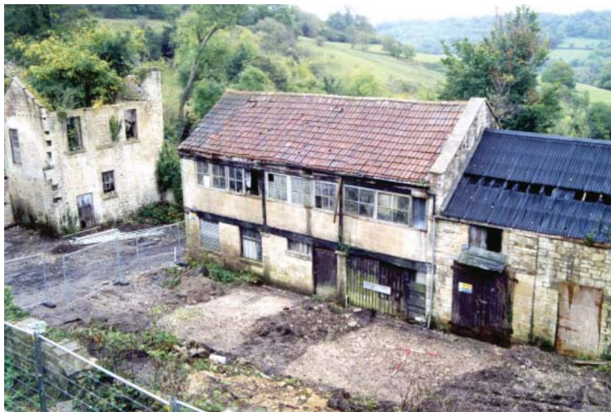
Plate 3: Trenches 9 and 10 from the north west
