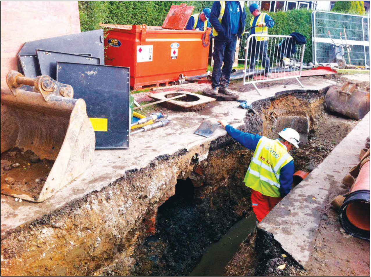
Plate 3: Pipe trench down Willow Lane showing 19th Century Culvert in section
