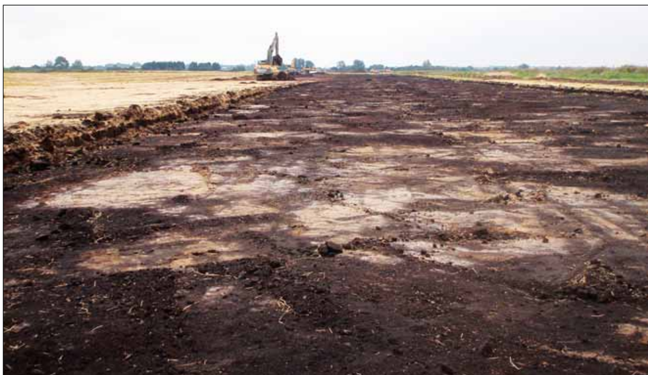
Plate 1: Topsoil strip across reservoir
