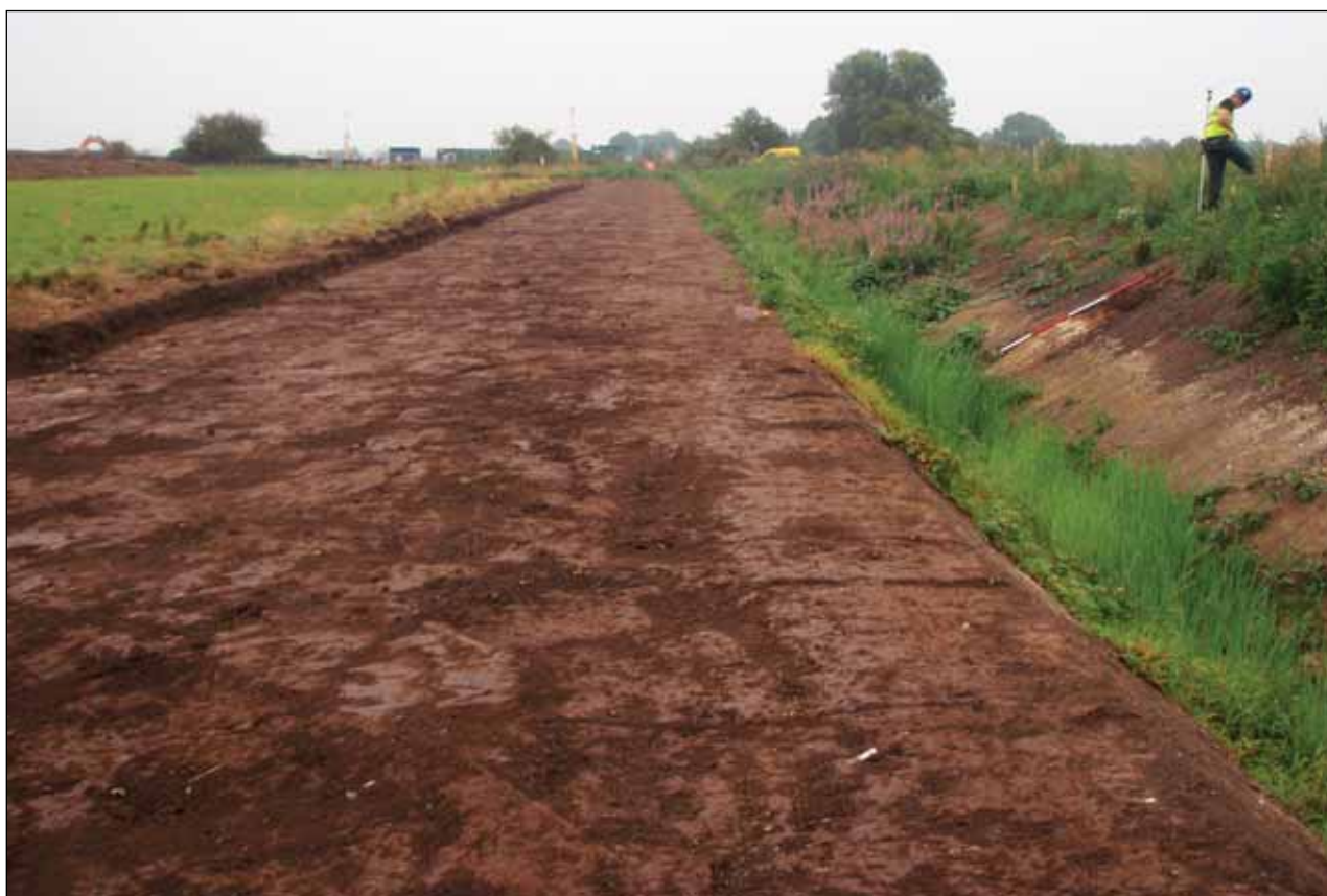
Plate 2: Extant ditch with topsoil strip for new drain
