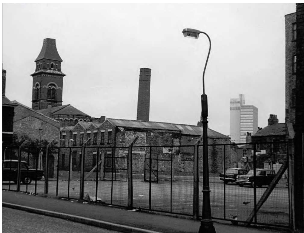
Plate 5: View across the study area from Jersey Street in c 1967, showing the south-eastern part of the site to have been cleared, and Blossom Street Works to the rear
