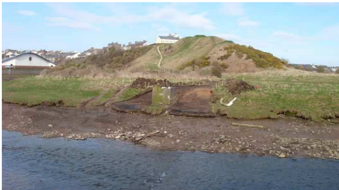
Plate 3: Topsoil stripping adjacent to the River Ellen
