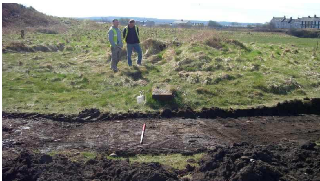
Plate 2: The central section of the proposed cycle path following topsoil stripping
