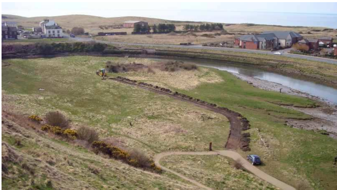
Plate 1: Topsoil stripping in progress
