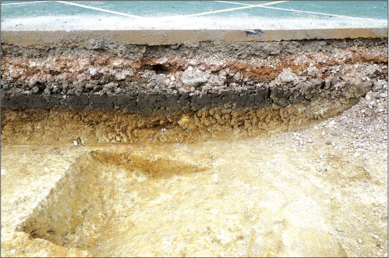
Plate 3: Photograph showing the layers that were used to build up the tennis court over ditch terminus 9 , taken from the south-west
