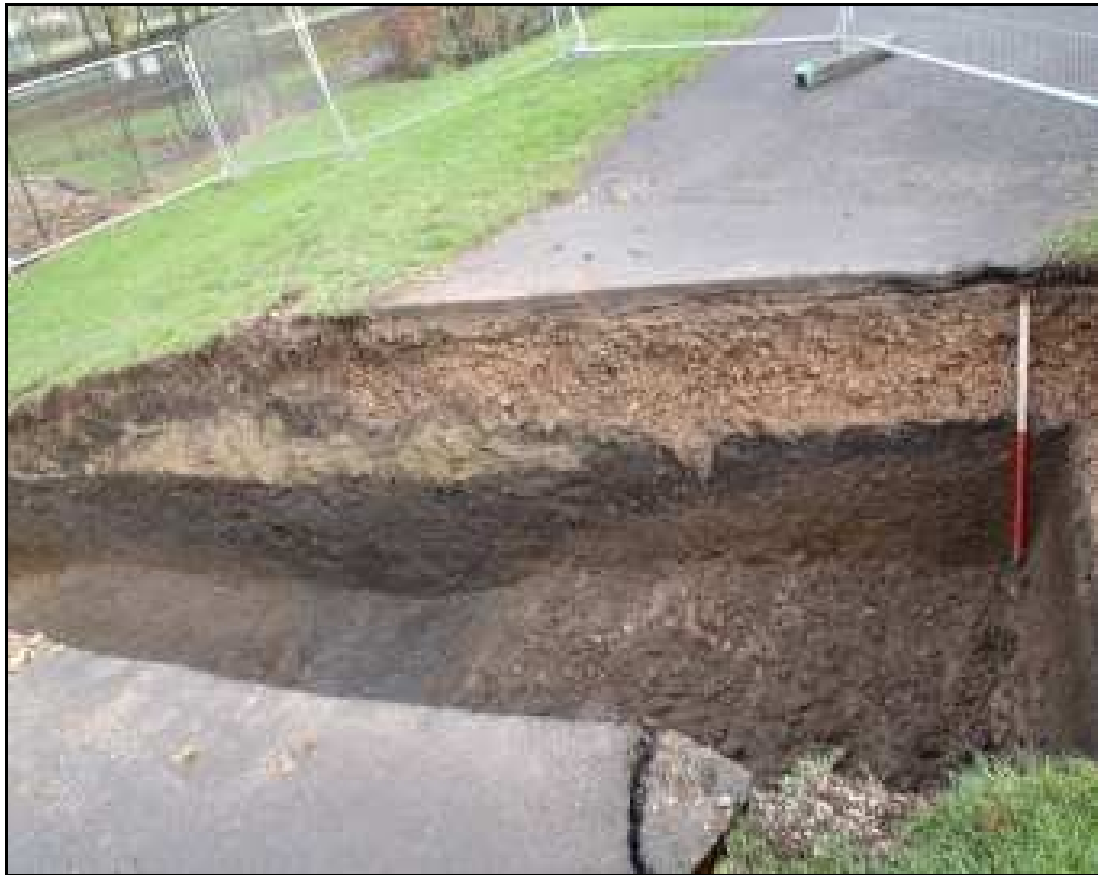
Plate 4: The west-facing section of Trench 20, showing the made ground deposits comprising the bank and cycle path. Viewed facing east.
