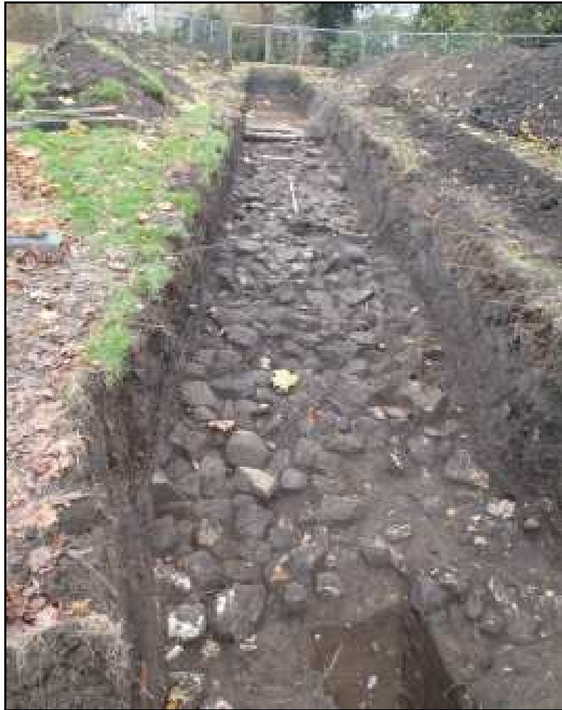
Plate 24: The rubble deposit (2217), probably representing the demolished remains of the fort wall with the start of the machine sondage visible in the foreground. Viewed facing south-west.
