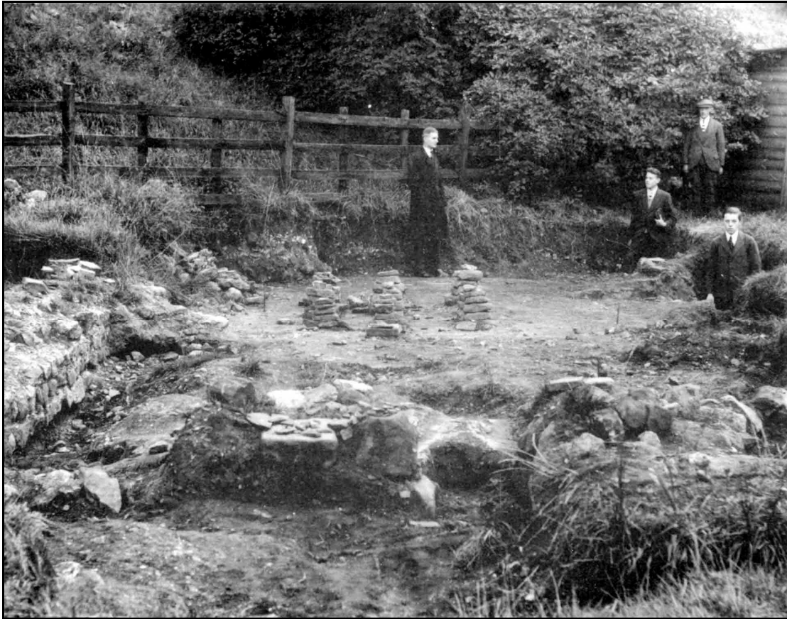
Plate 3. Picture of the hypocaust system associated with the mansio/bath house excavated on Parker's Piece c 1924
