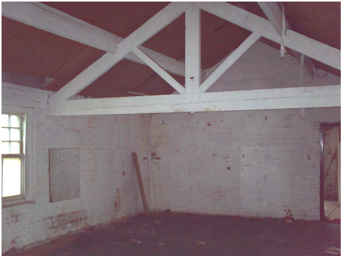
Plate 9: General view of the interior of the stable block
