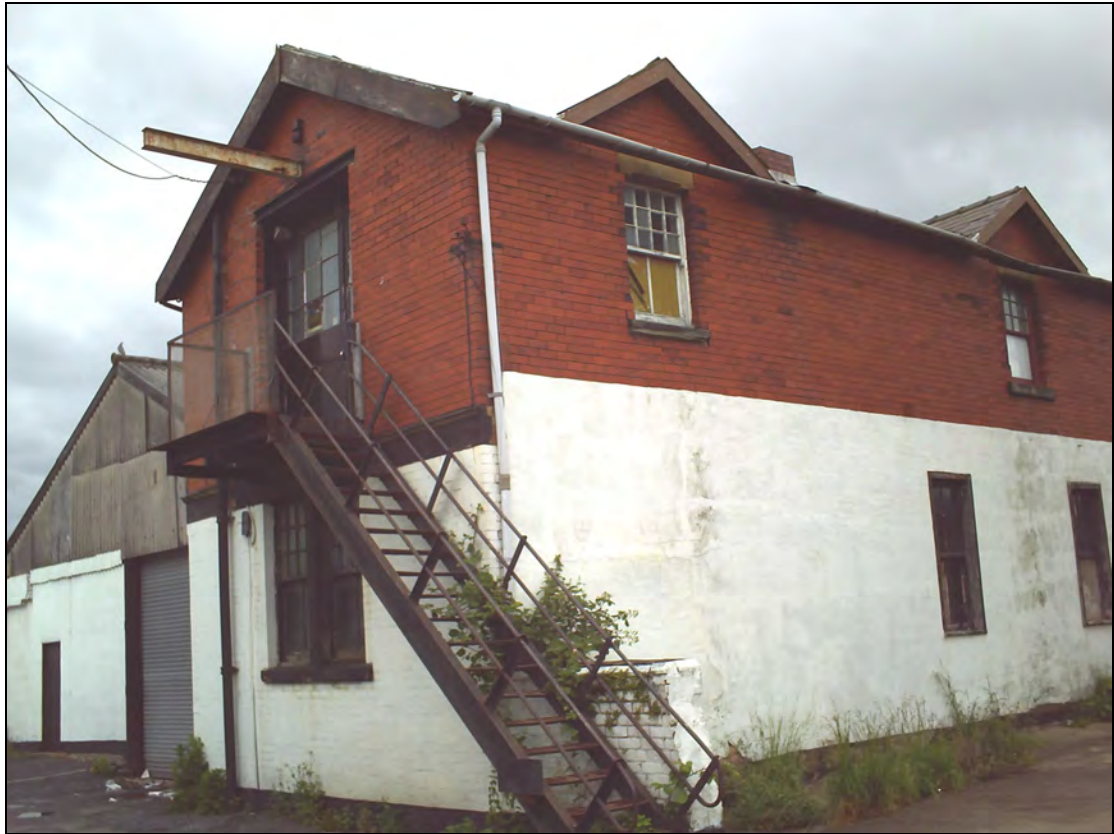
Plate 1: The west elevation of the stable block
