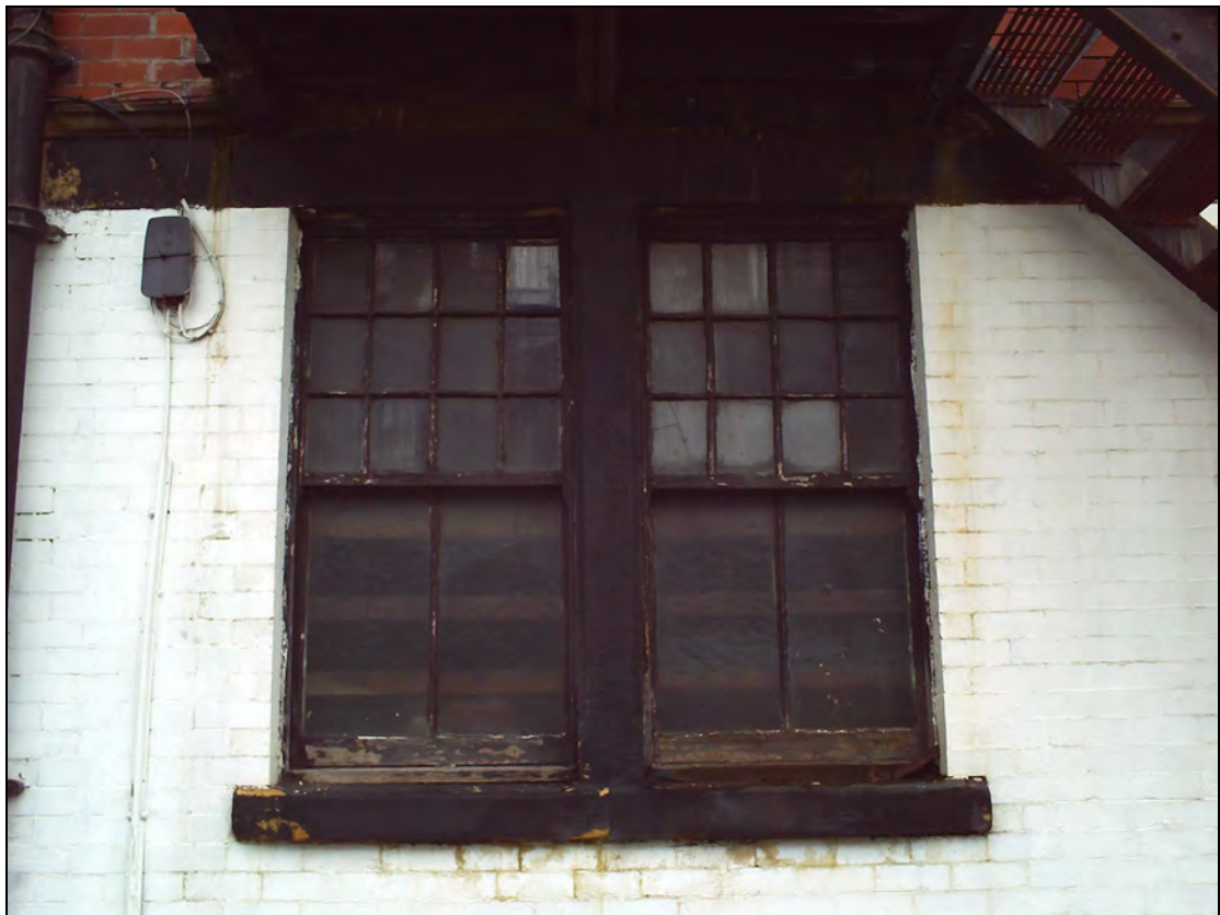
Plate 5: Detail of the sash window on the west elevation
