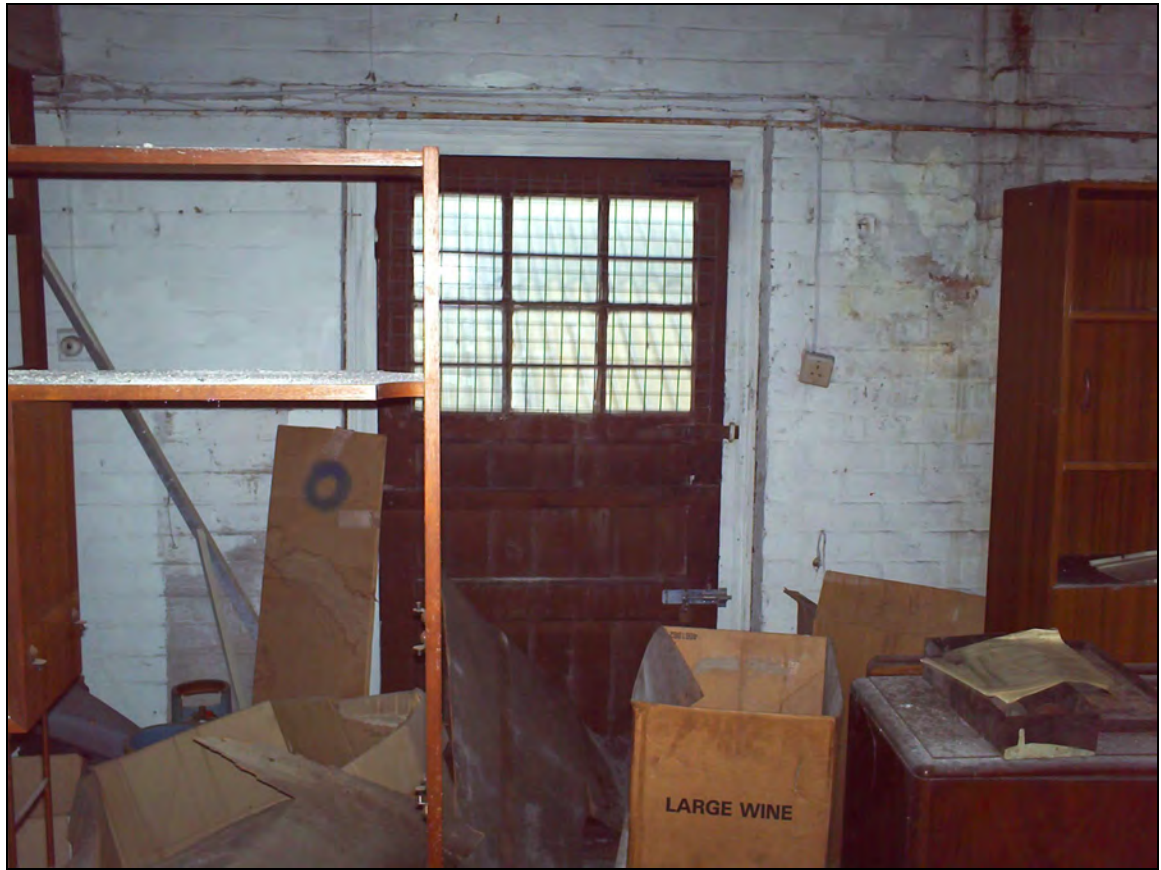
Plate16: Loading door on northern elevation, facing north
