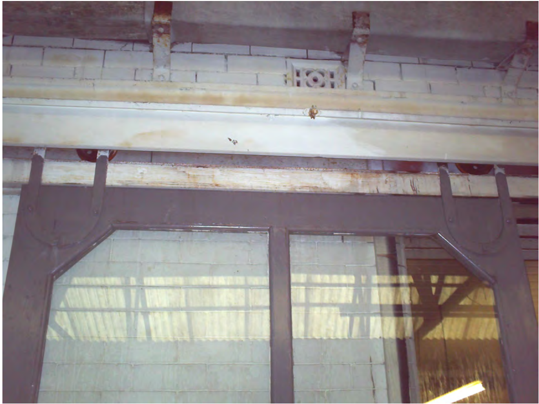
Plate 8: Detail of the sliding door on the north elevation
