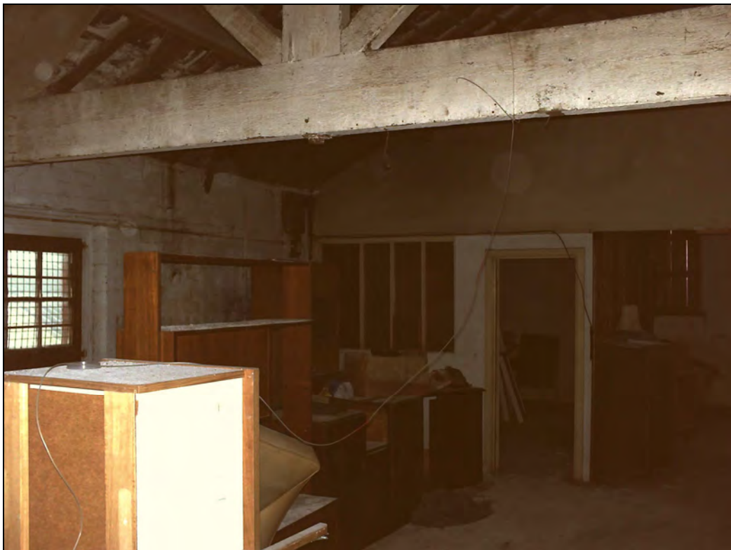
Plate13: Office partition at eastern end of room 6
