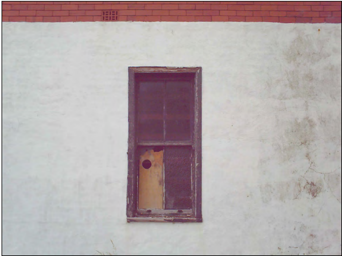
Plate 6: Detail of a ground-floor sash window on the southern elevation
