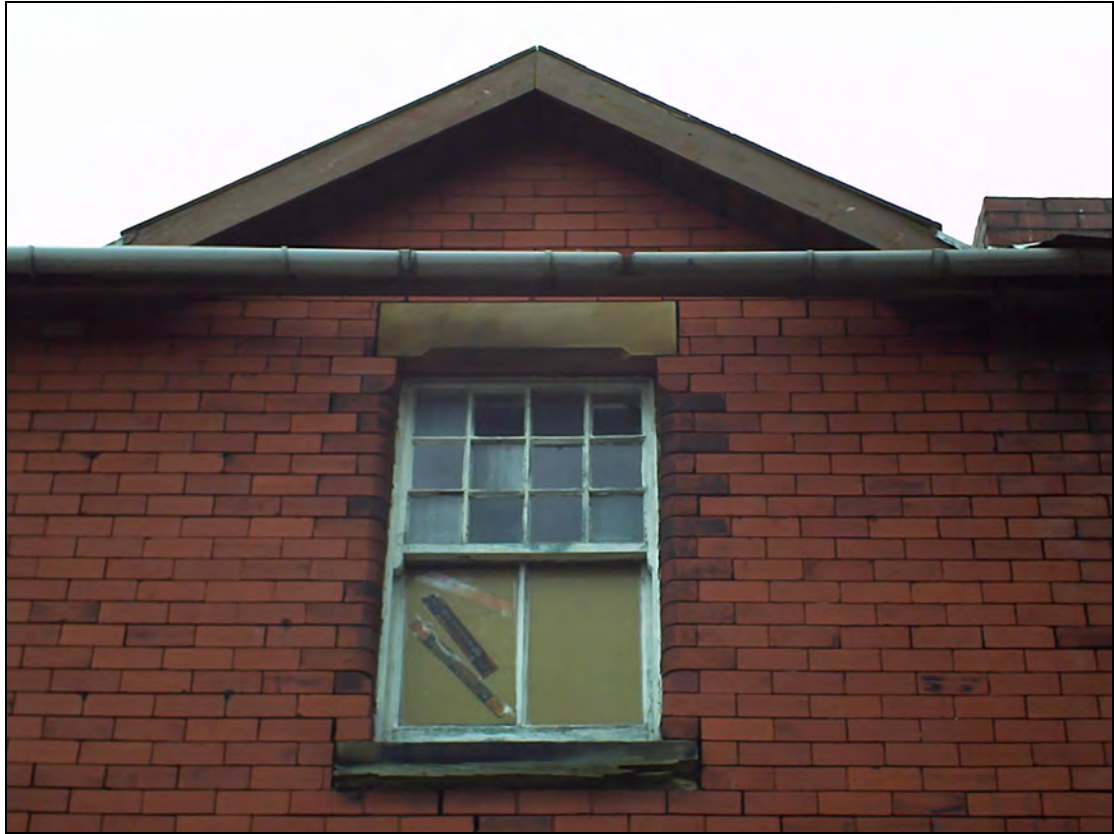
Plate 4: Typical first-floor window
