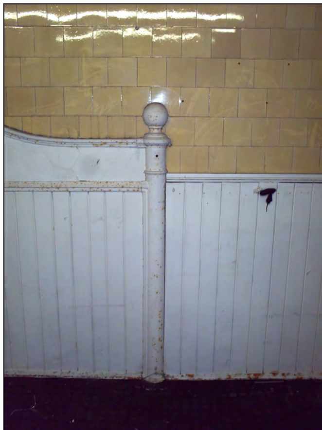
Plate11: Detail of the timber panels and iron posts within room 2
