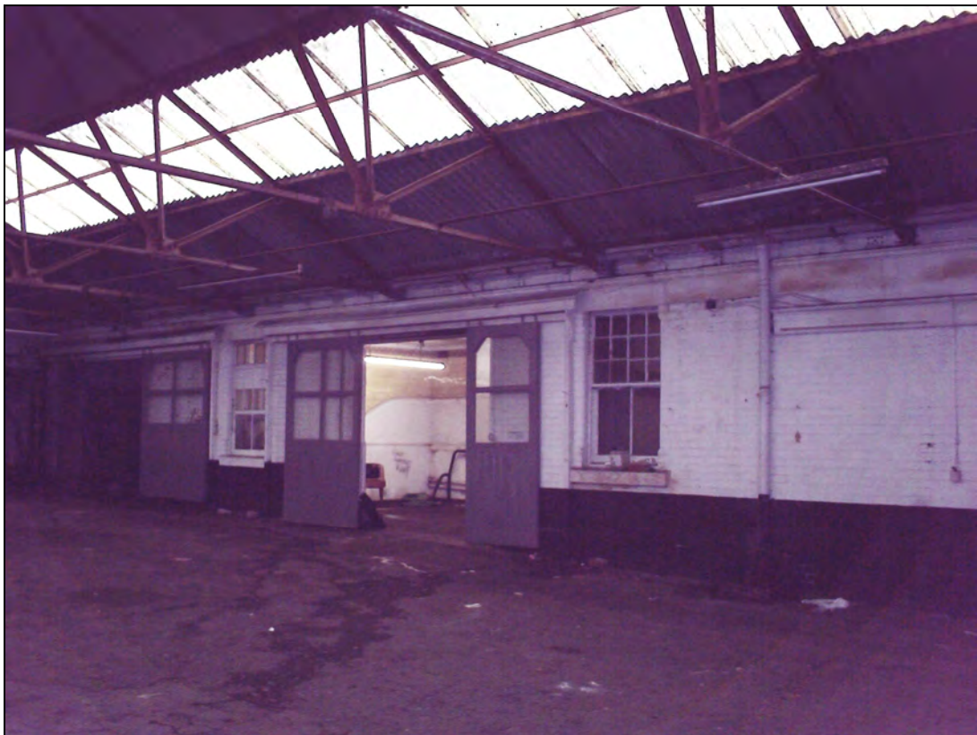
Plate 7: North elevation, with rail-mounted sliding doors
