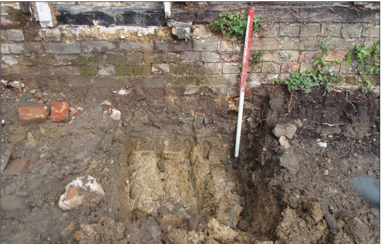
Plate 2: Phase 2 excavation of under-pinning pits
