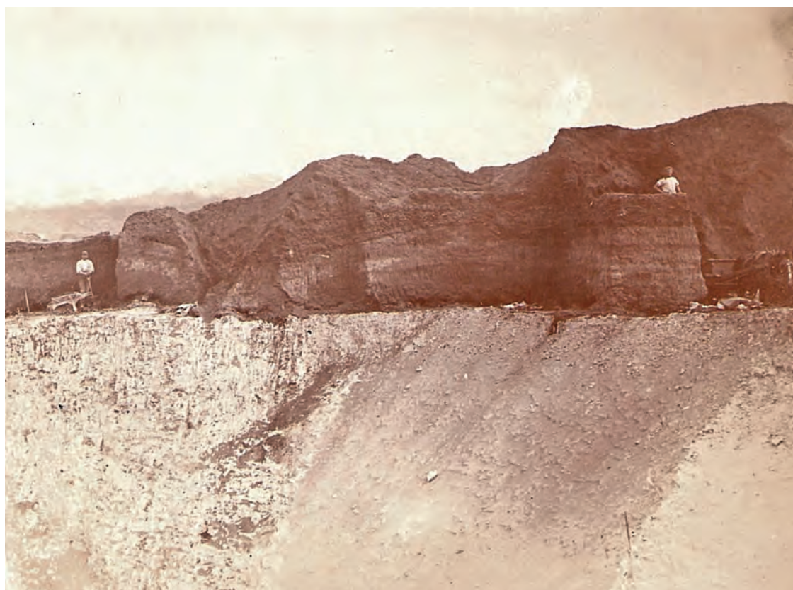
Fig. 2.3 Gravel quarrying in 19th/early 20th century; Galley Hill Pit. Note worker on left with shovel and barrow for aggregate removal.
