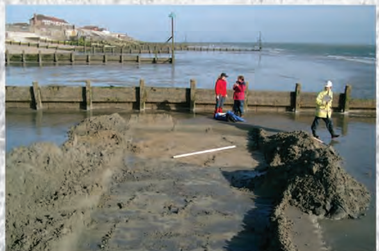
2.4.5 Excavated edge of West Street, Selsey Channel as predicted from the EM31 conductivity survey
