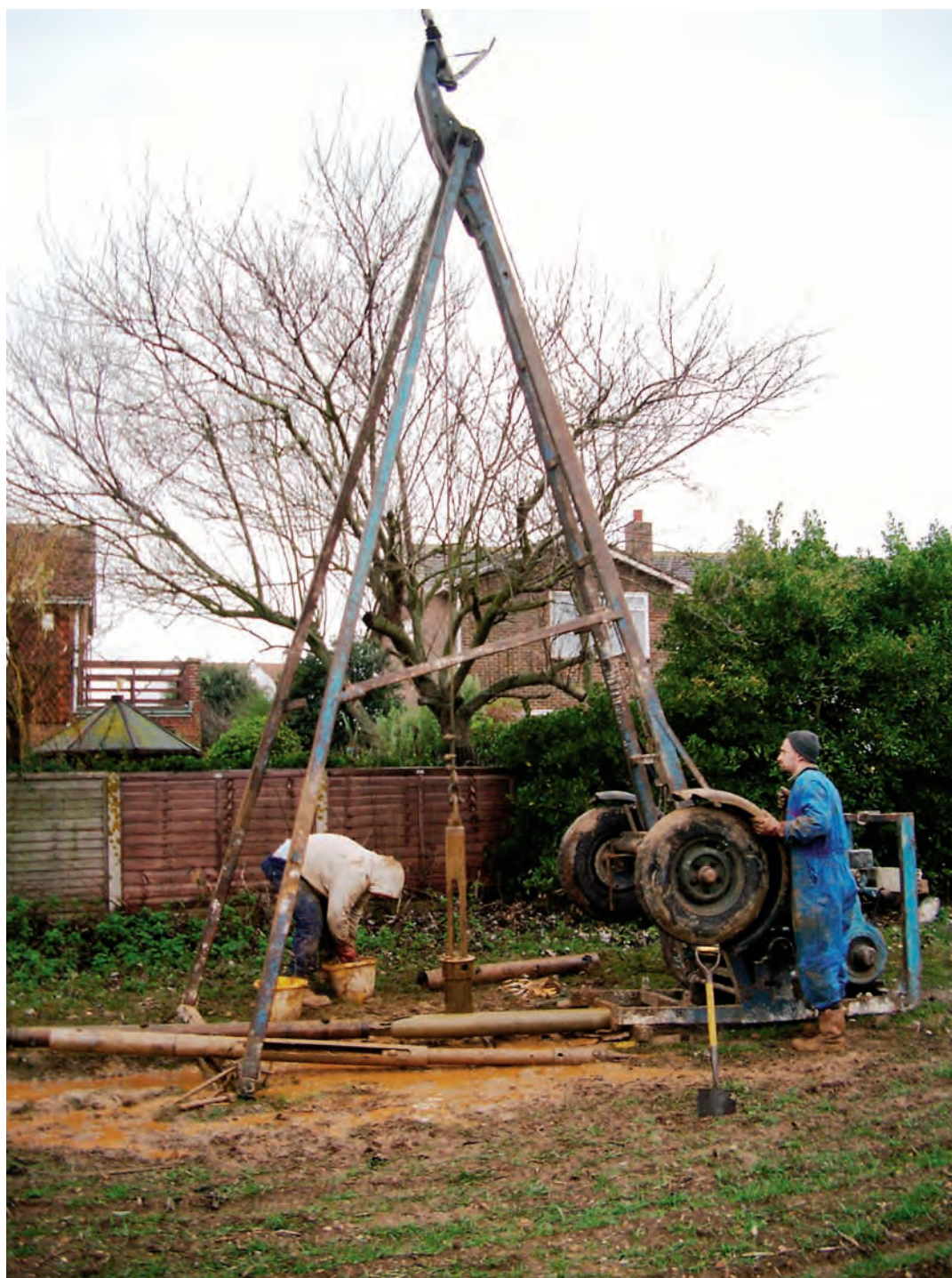
Fig. 2.4 Shell and auger drill rig at West Wittering, West Sussex
