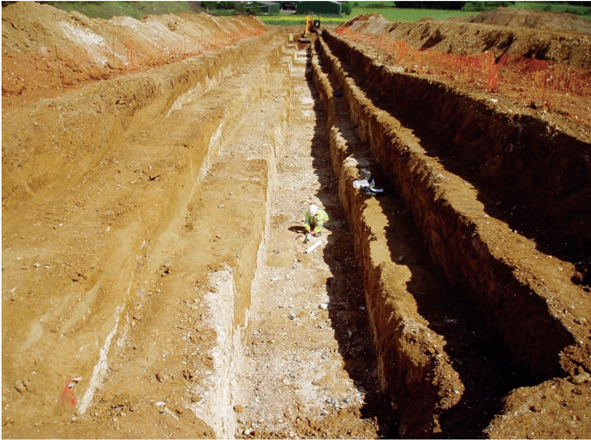
Fig. 2.11 Long trench excavated in a stepped fashion through Devensian slope deposits at Dartford A2/A282 crossing
