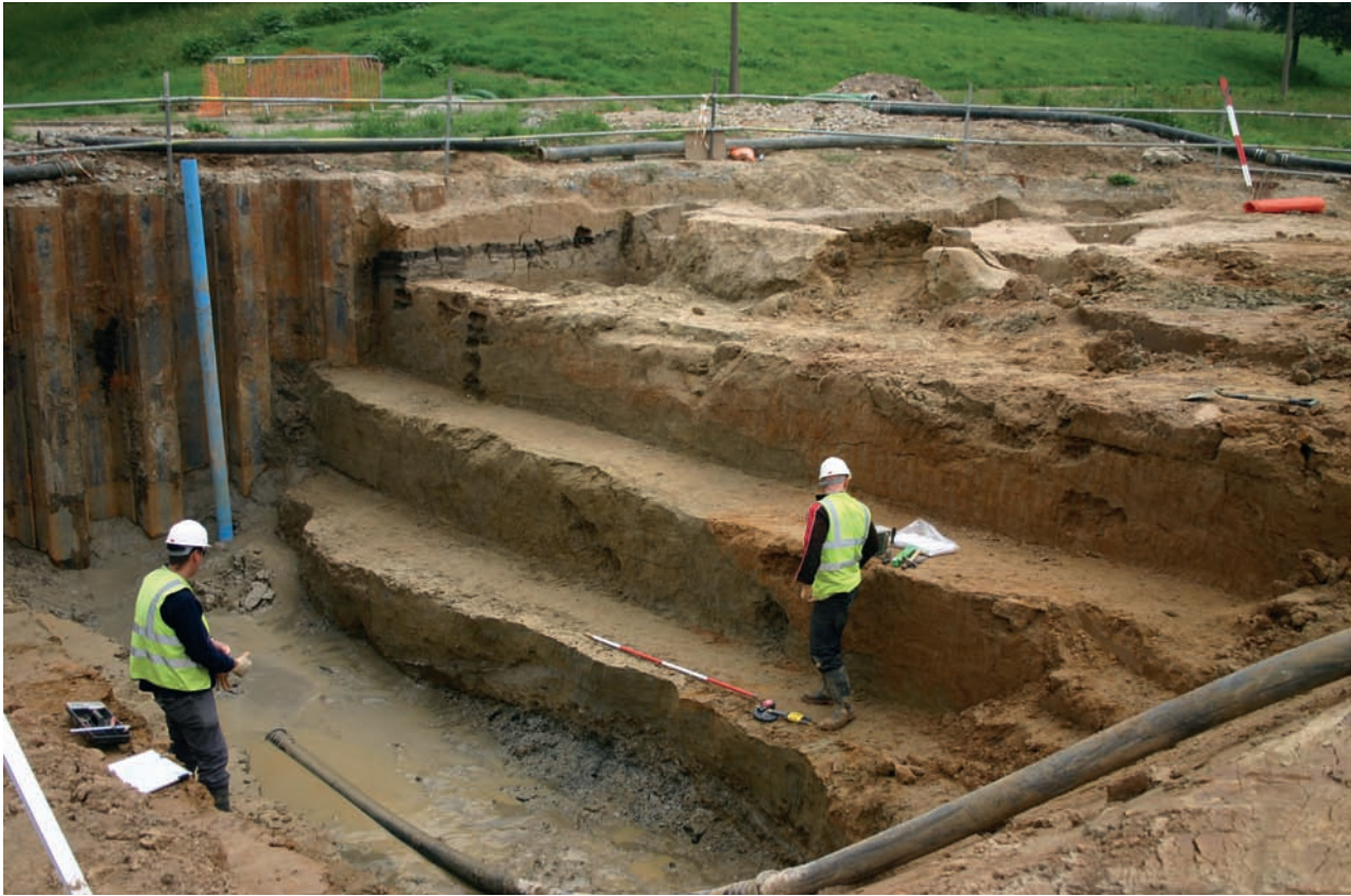
Fig. 2.9 Stepped trench at Northfleet Sewage Works during investigation of Devensian colluvial sediments
