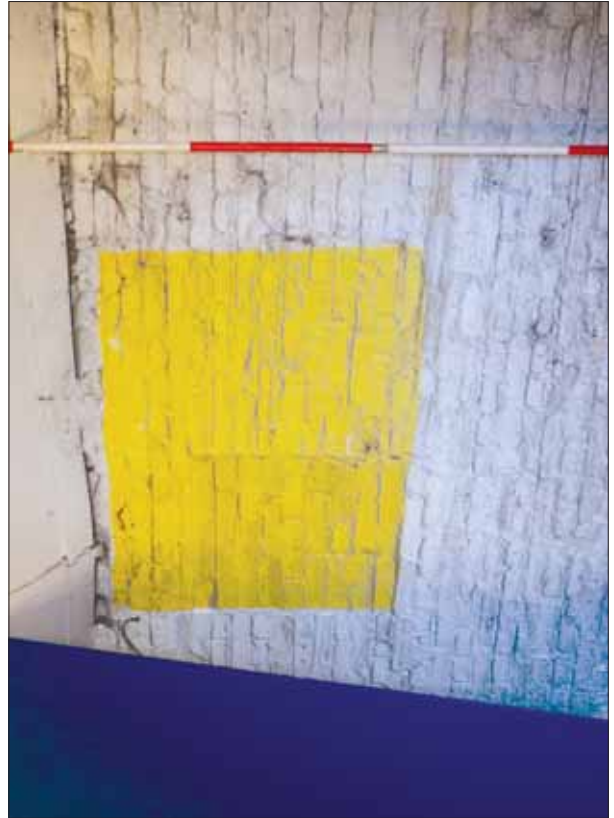
Plate 11: Blocked window east wall of Room 1, from south-west
