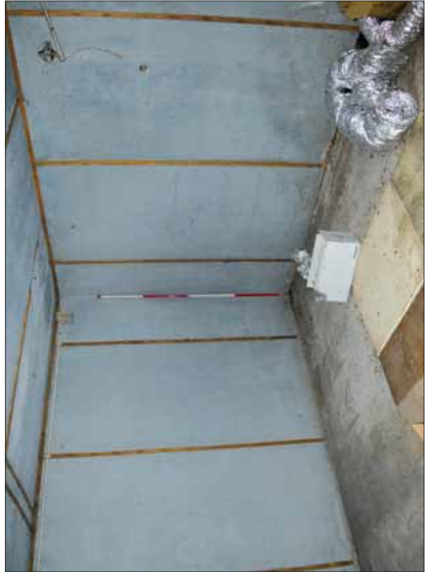
Plate 31: Detail of north-east corner of Room 5, from south-west
