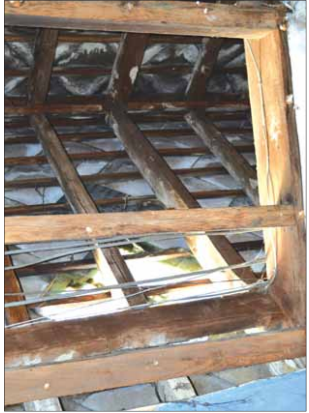
Plate 16: Detail of exposed roof space in Room 1, from east
