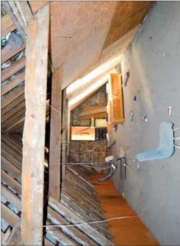
Plate 38: Detail of Room 8, from east
