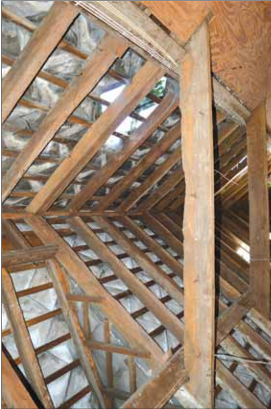
Plate 41: Detail of Timber roof Construction above Room 8, from east
