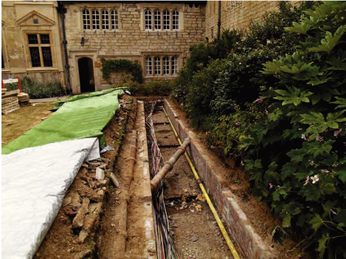
Plate 3: Area on the south side of the Quad, showing the brick lined cable duct
