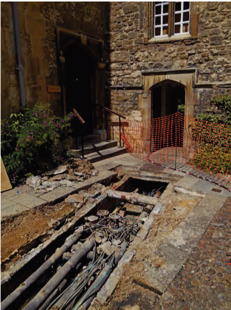
Plate 4: Area on the west side of the Quad, showing the brick lined cable duct
