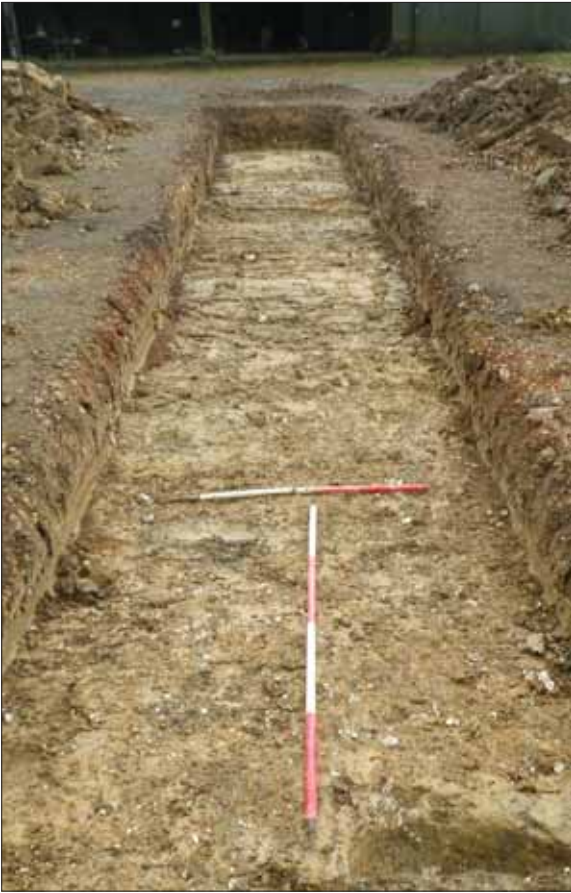
Plate 1 Trench 1 from the North with pits 28 and 32 in foreground
