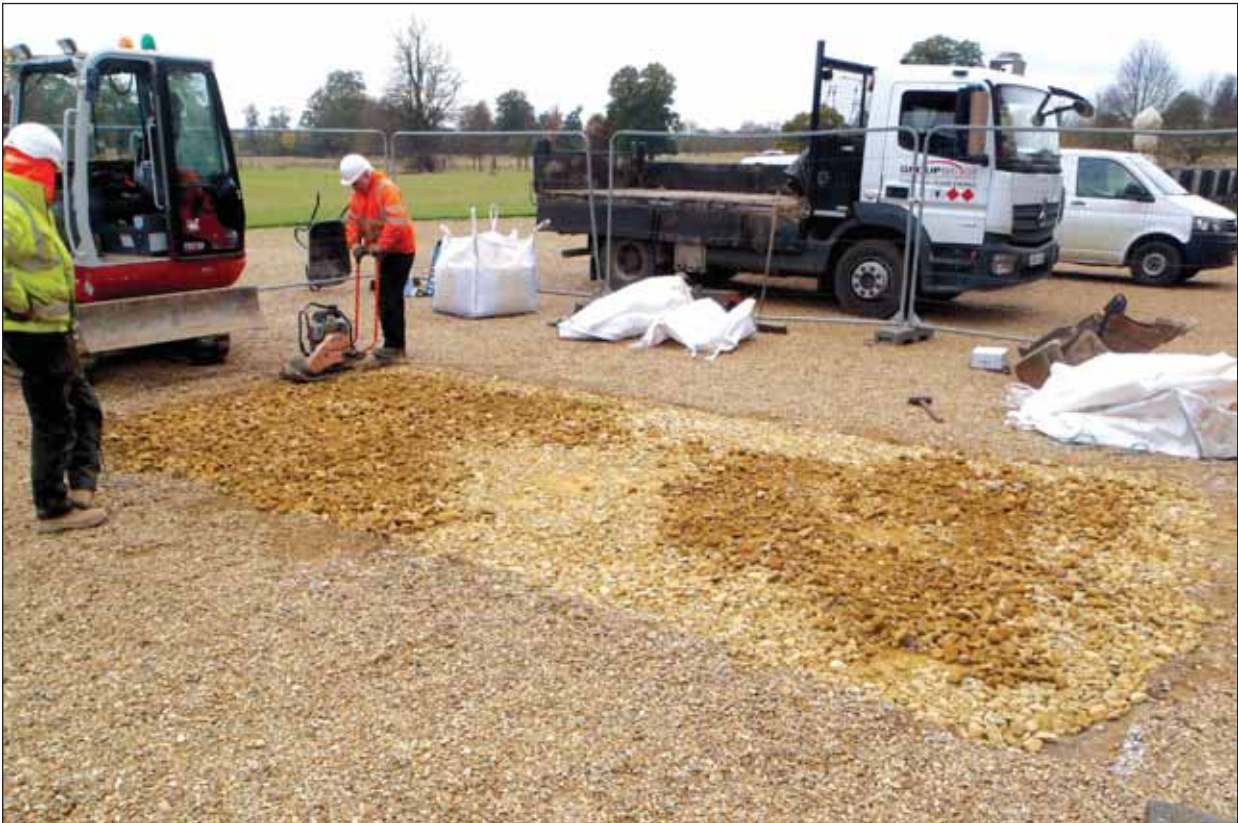
Plate 5: Reinstatement in progress, from east
