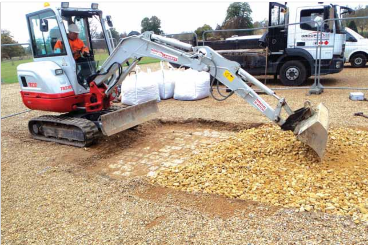
Plate 4: Reinstatement in progress, from east
