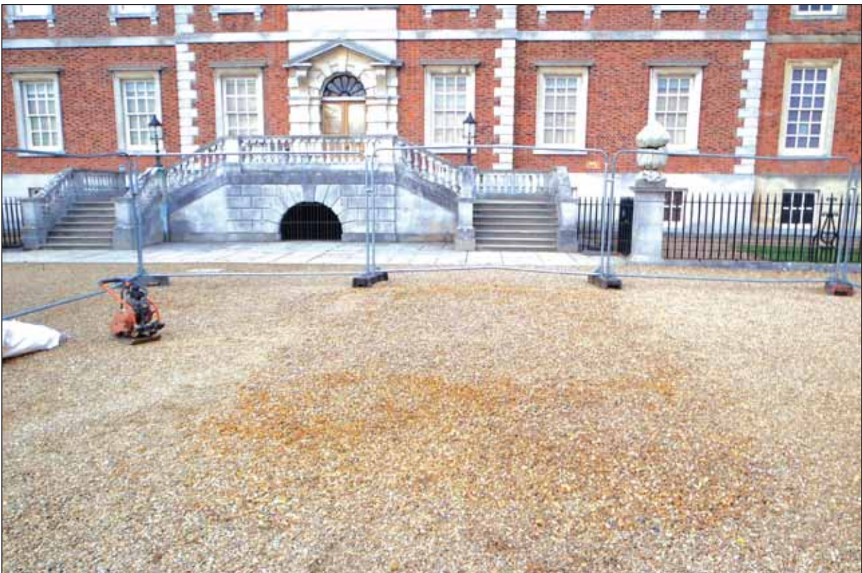
Plate 6: Reinstatement complete, from south
