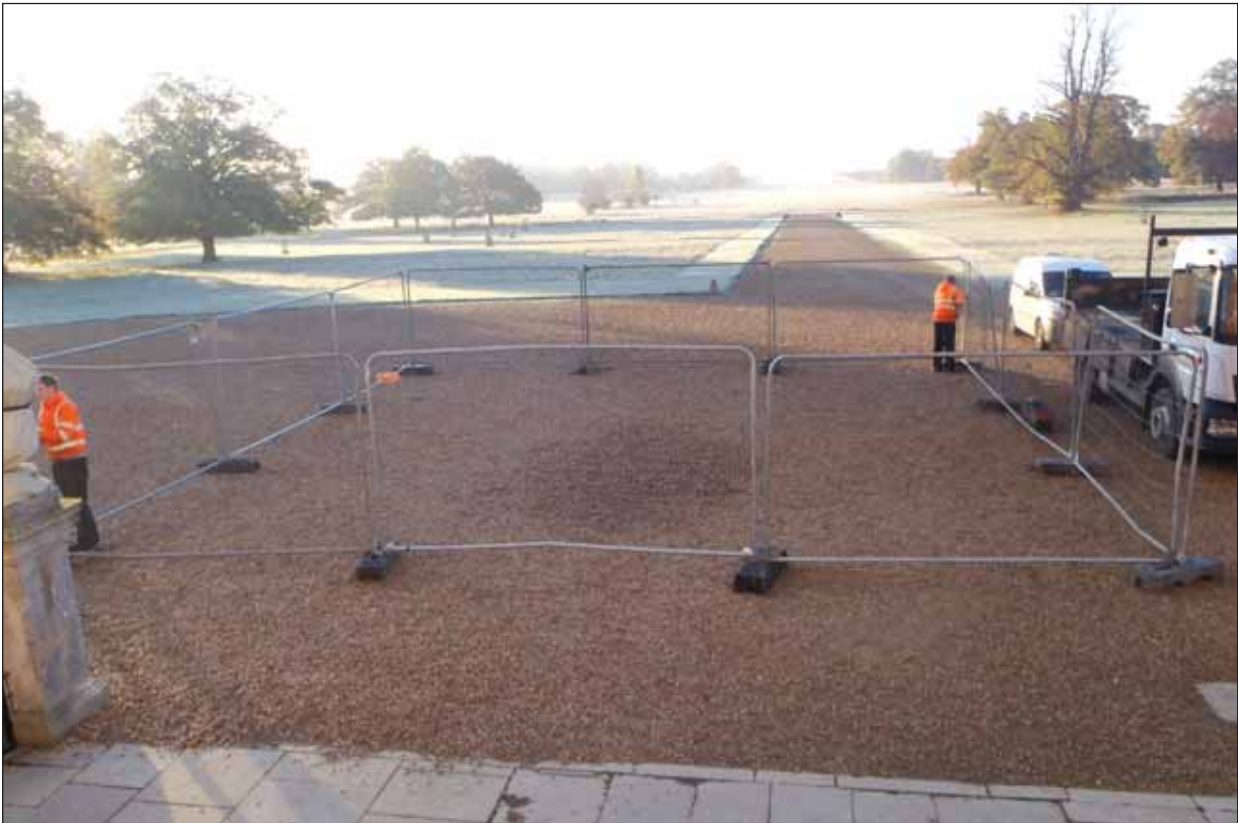
Plate 1: Pre-excavation showing oil spill, from north
