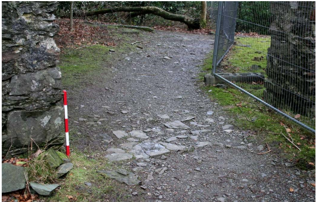
Plate 36: The stone threshold between jambs of the Station flanking wall arch
