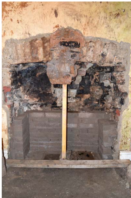
Plate 45: Brick arched fireplace after the removal of the 1950's surround
