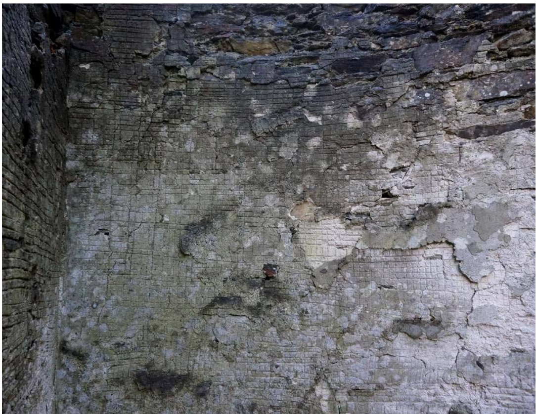
Plate 32: The criss-cross key pattern of the lime plaster scratch coat in the stairwell
