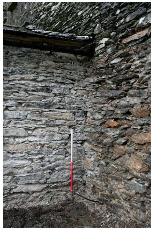
Plate 43: Well bonded junction between cottage and flanking wall
