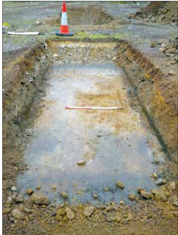
Plate 8: Trench 7, looking north-east
