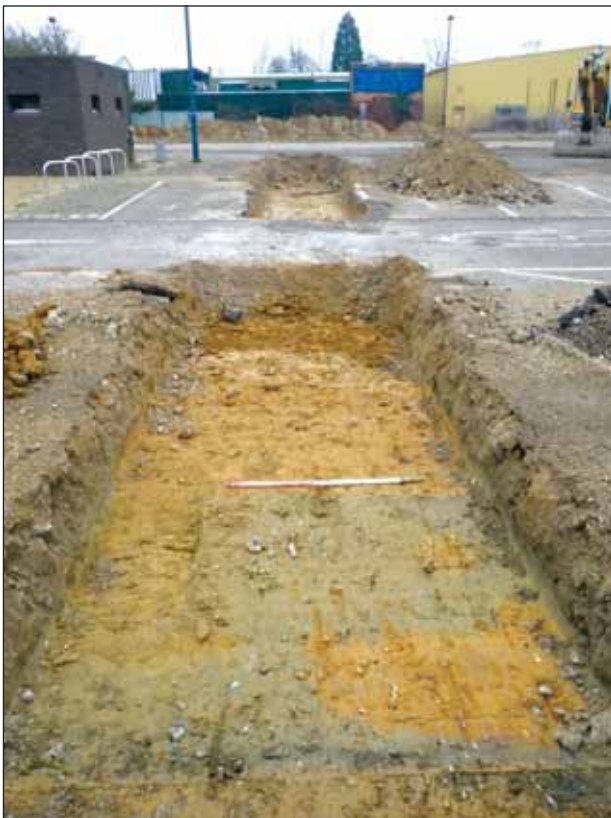
Plate 3: Trench 2, looking north-east
