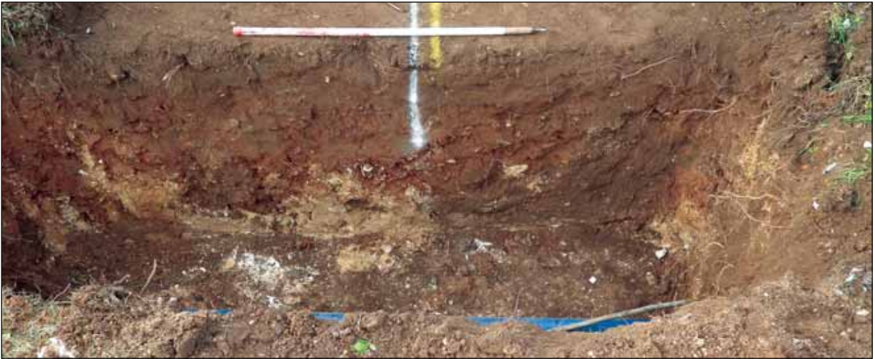
Plate 1: Excavation for Booster station looking west
