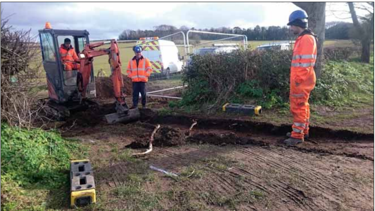
Plate 2: Excavation of parking area
