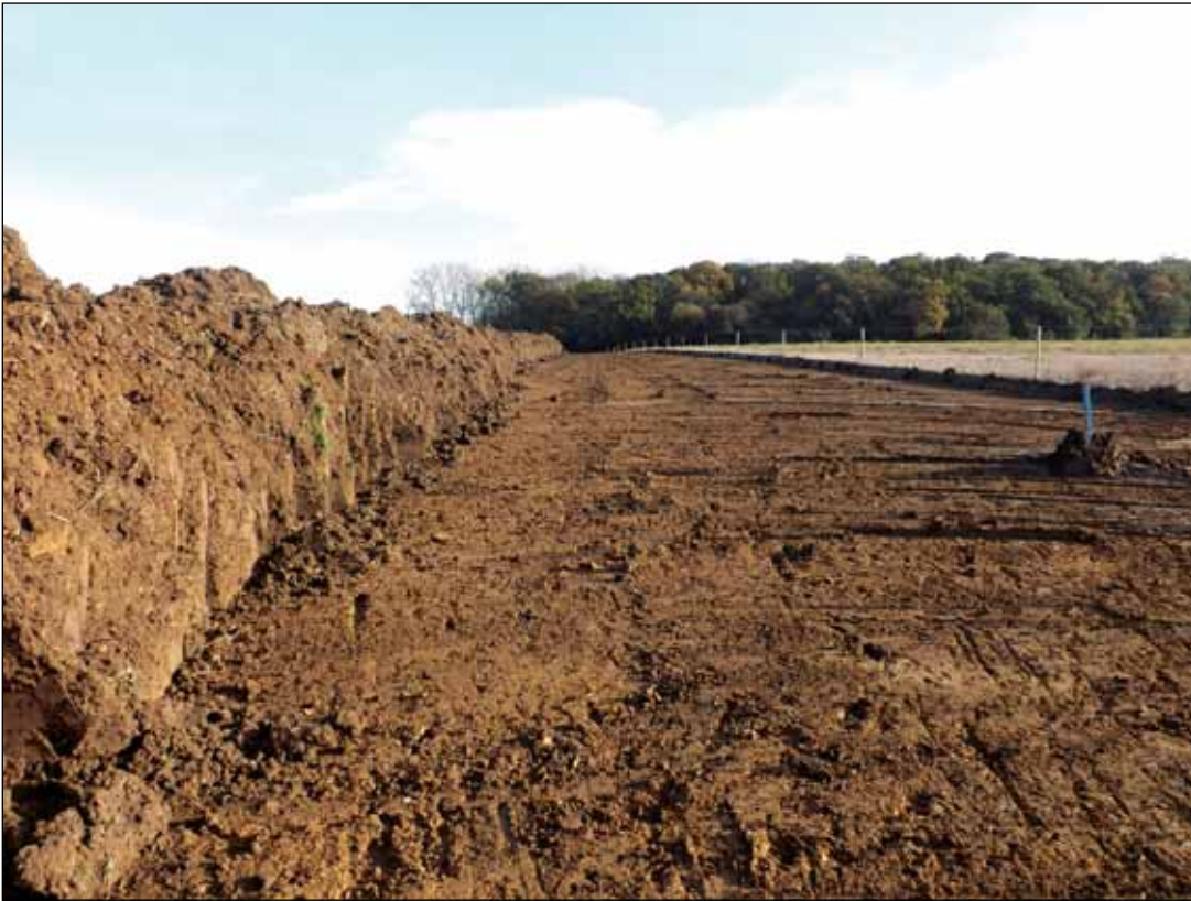
Plate 1: Chainage 900m after topsoil strip, facing east
