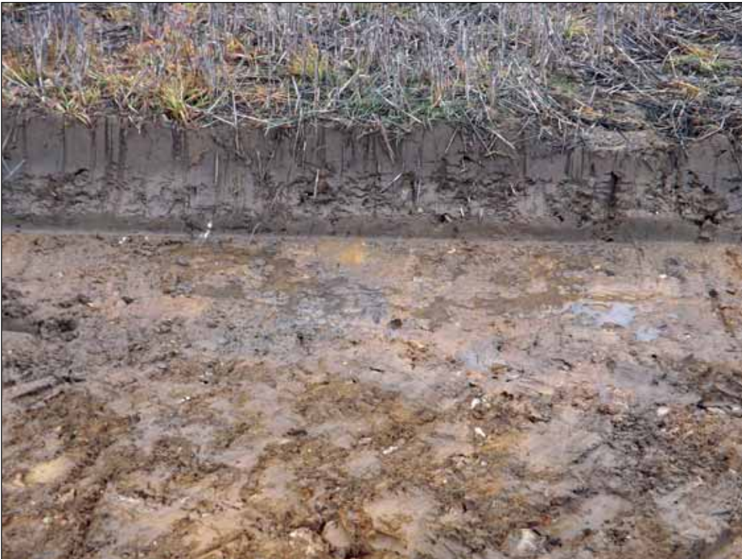
Plate 2: Depth of topsoil strip at Chainage 600m showing under lying clayey subsoil
