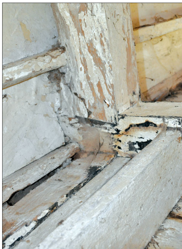
Plate 75: Detail of wall plate and cross beam of Room 1 in Building D
