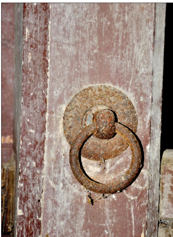
Plate 21: Tie ring to stable door post in Room 1 of Building A
