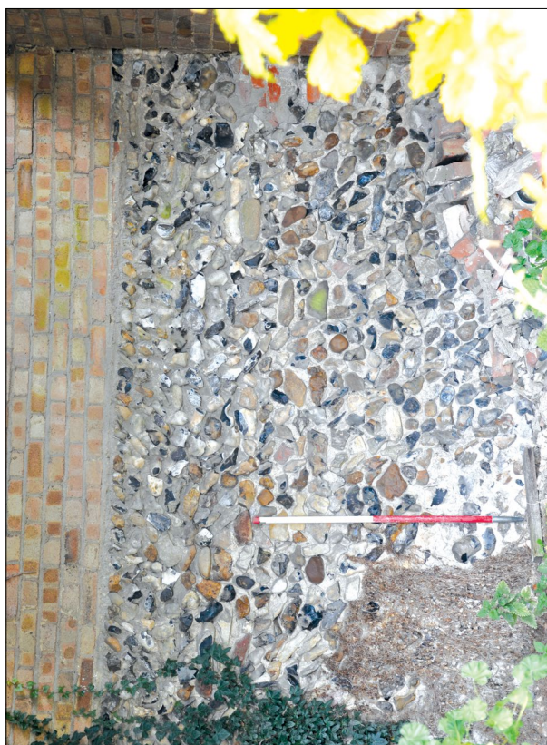
Plate 49: Detail of flint wall to the north-east elevation of Building C
