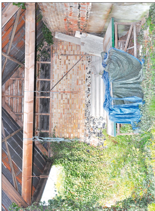
Plate 41: Northern wall of Building B showing additional building to top of existing wall
