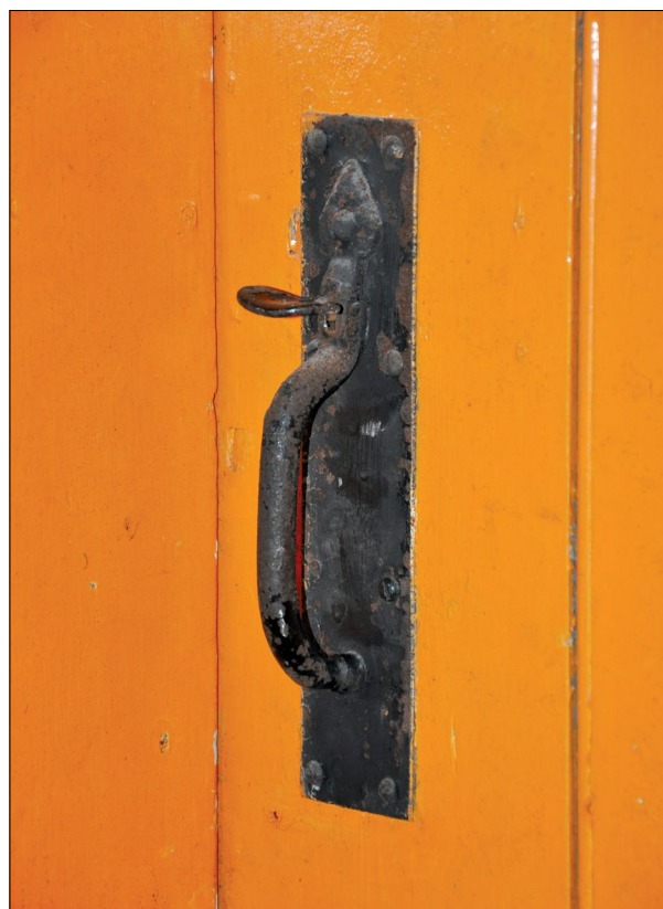
Plate 28: Detail of upright latch of tack room door in Building A
