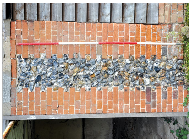
Plate 63: Detail of flint dressing to the eastern elevation of Building D
