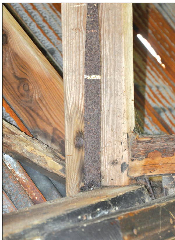
Plate 52: Detail of iron tie to the roof plate and cross beam, in Building C
