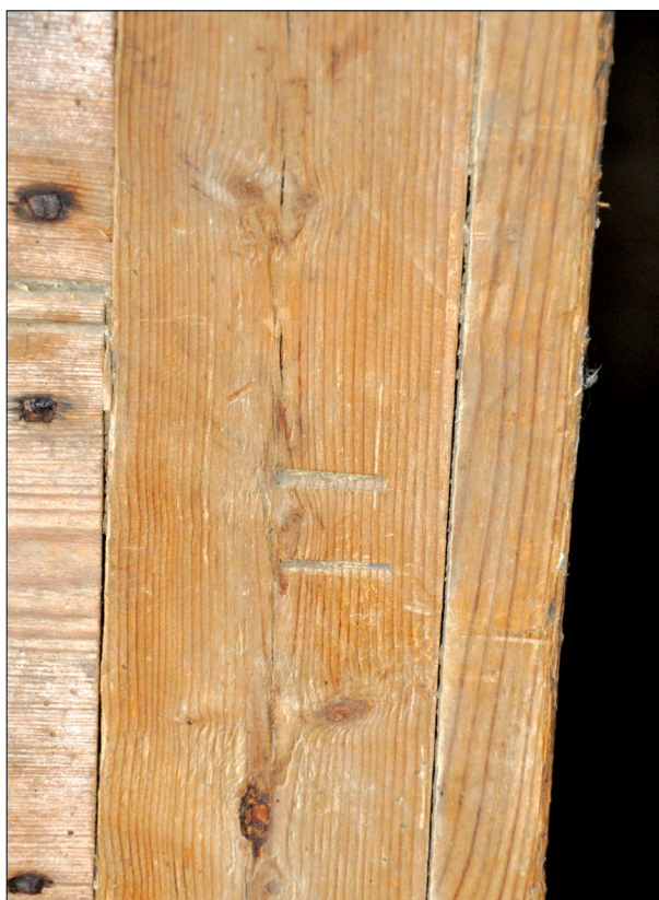
Plate 94: Carpenters marks on internal woodwork to stalls of Building E
