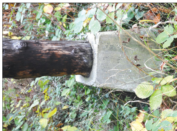
Plate 47: Detail of concrete base and post to Building C
