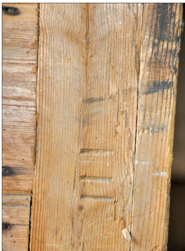
Plate 93: Carpenters marks on internal woodwork to stalls of Building E
