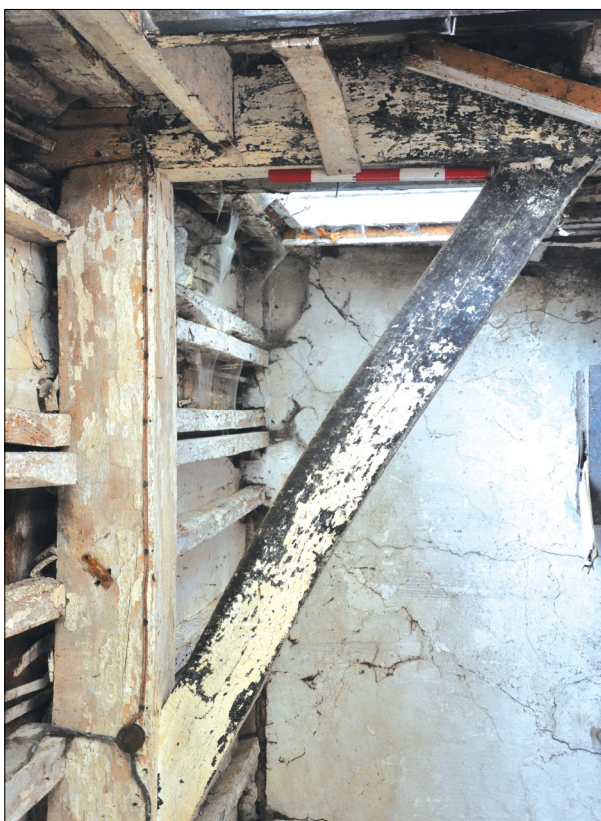
Plate 73: Detail of brace in roof structure of Room 1 in Building D
