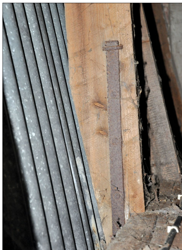
Plate 96: Detail of cross beam and iron brace to roof structure of Building E
