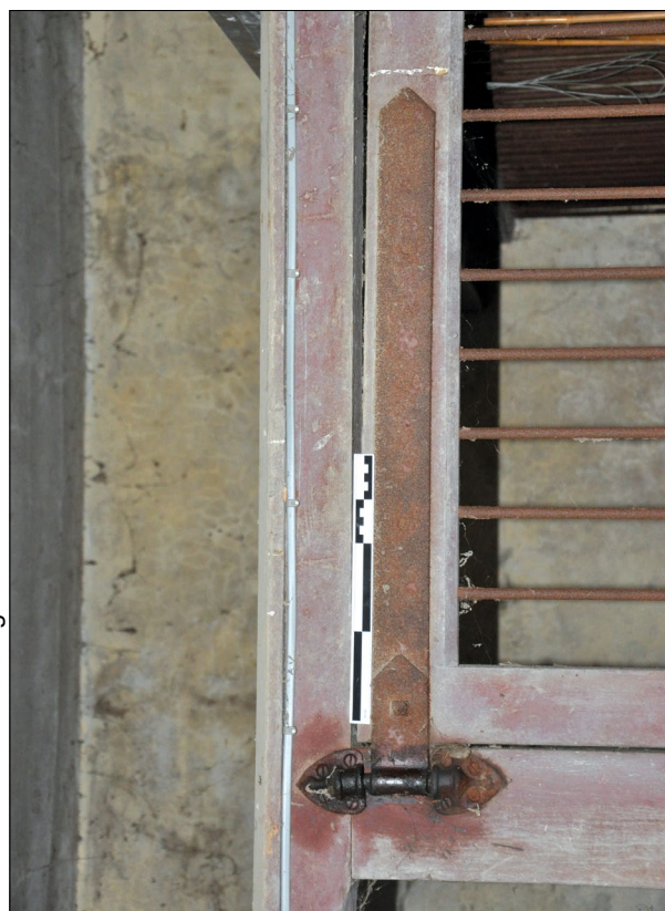
Plate 20: Detail of strap hinge to stable door in Room 1 of Building A
