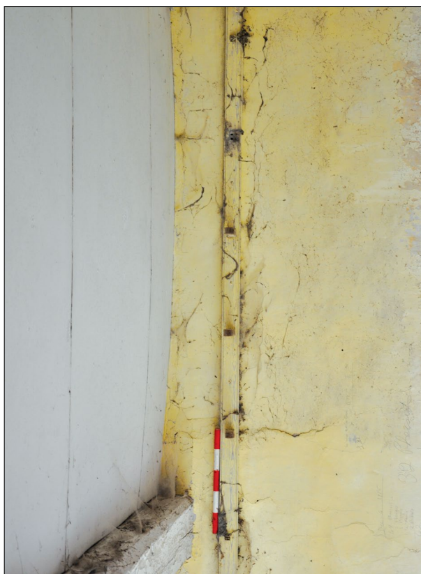
Plate 82: Tack rail at roof level on the northern wall of Room 2 in Building D
