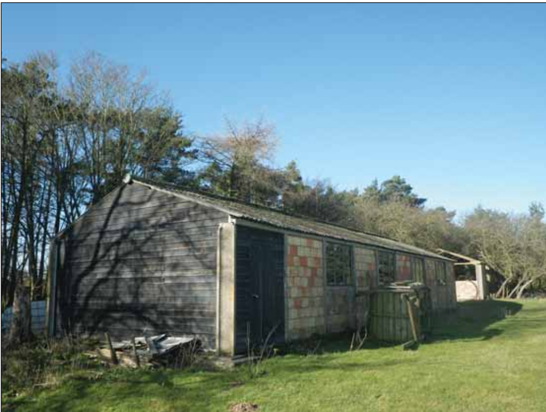
Plate 8: Standing remains of houses from POW camp, looking north-west.
