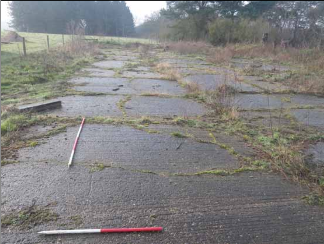
Plate 9: Concrete surface, looking south.
