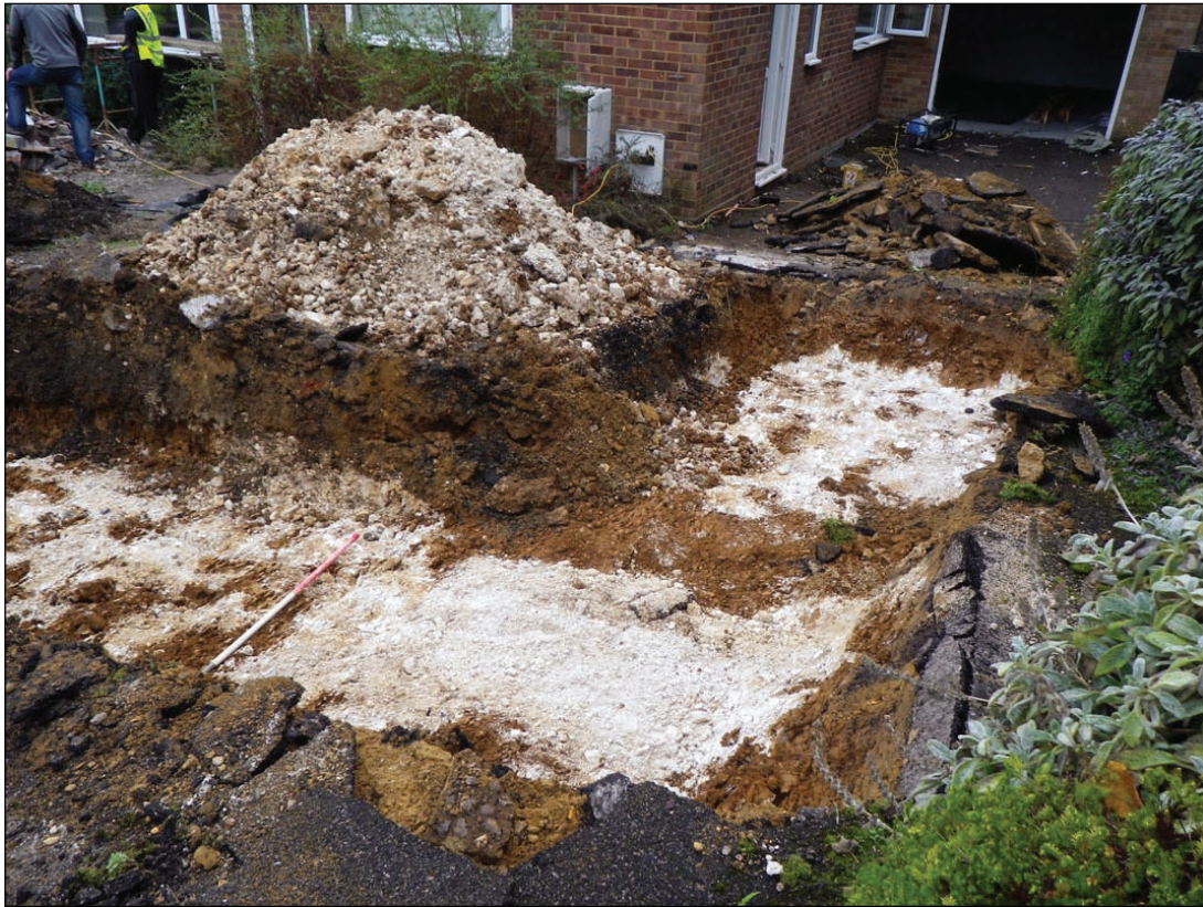
Plate 2: Trench 1, looking north-north-east
