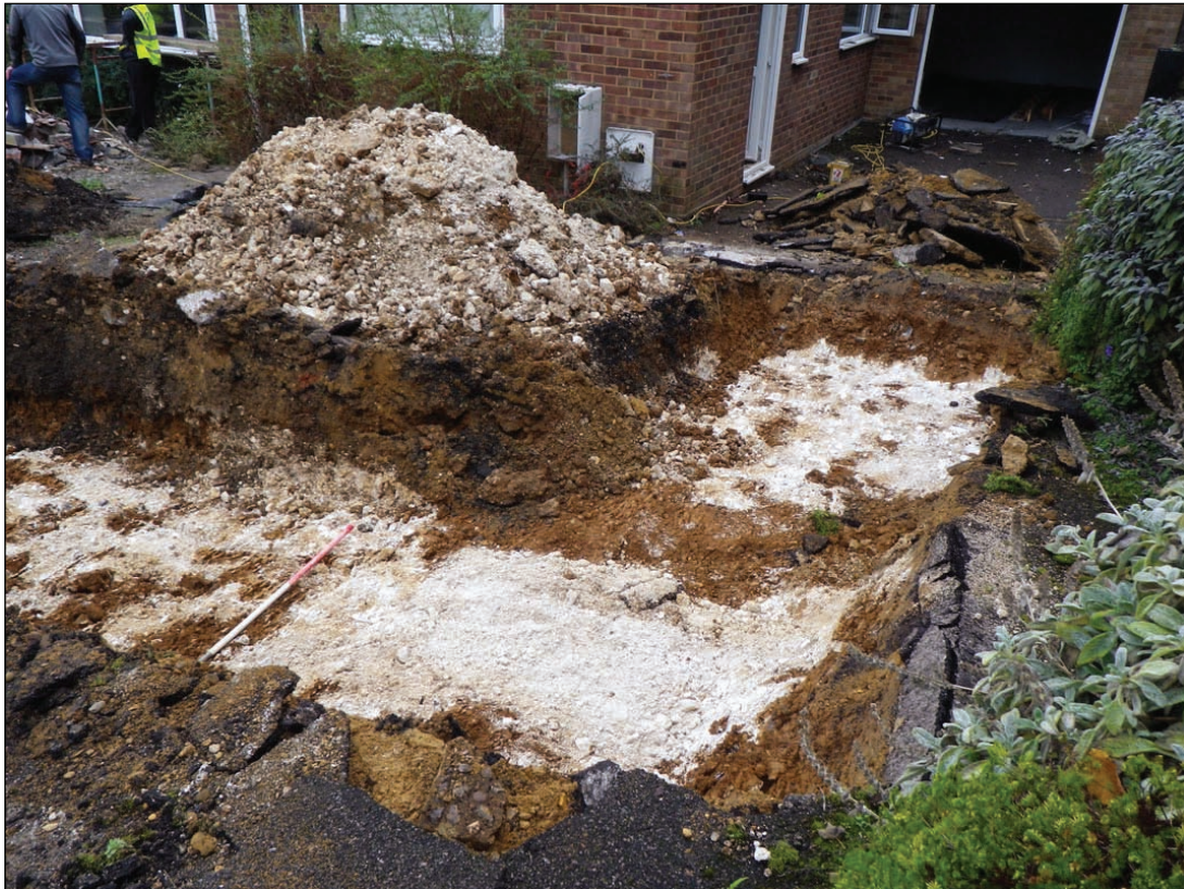
Plate 2: Trench 1, looking north-north-east
