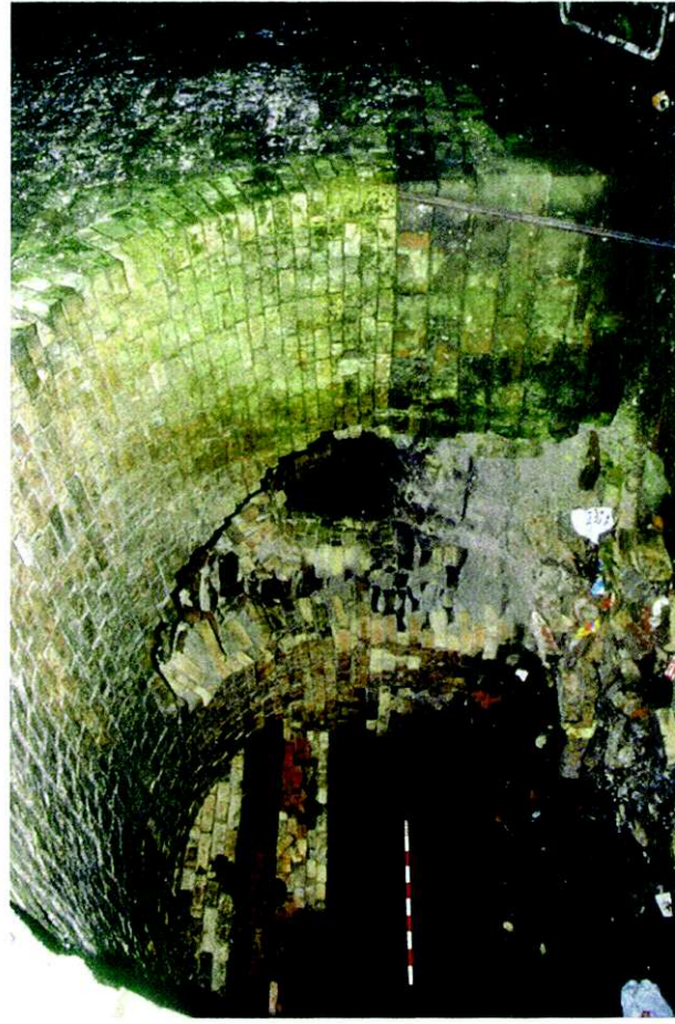
Plate 19: No.2 Furnace - N.W. blowing vault, showing vaulted 'drying passage'.
