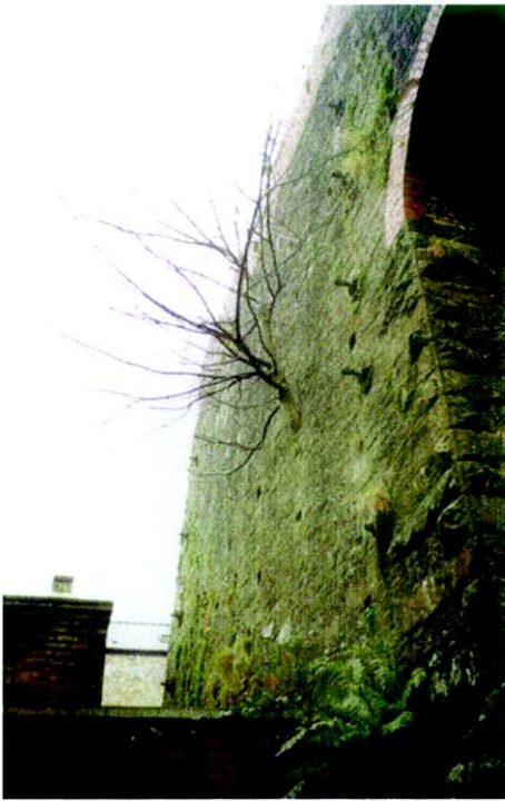
Plate 25: No.4 Furnace - sycamore growing in N.E. elevation.
