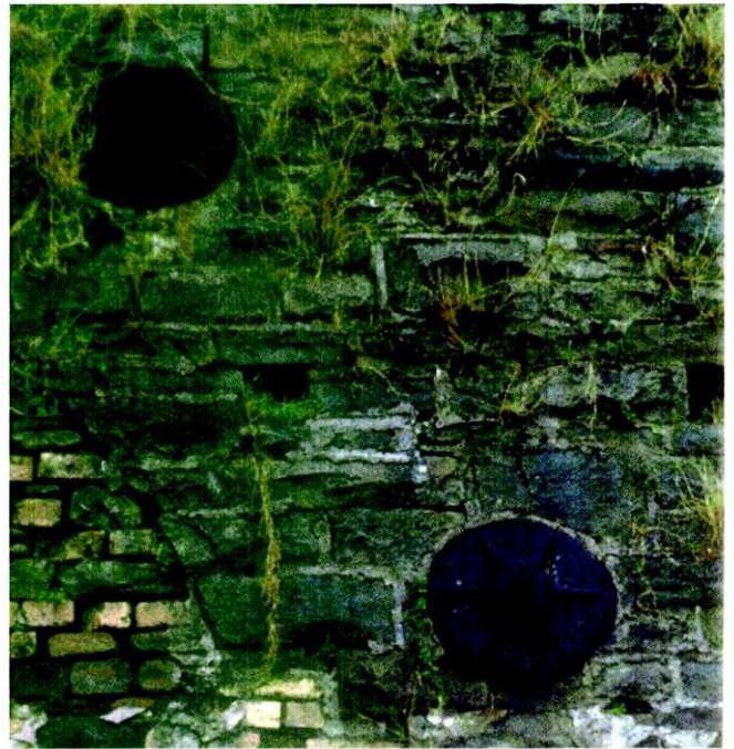
Plate 10: No.1 Furnace - later circular tie plate.
