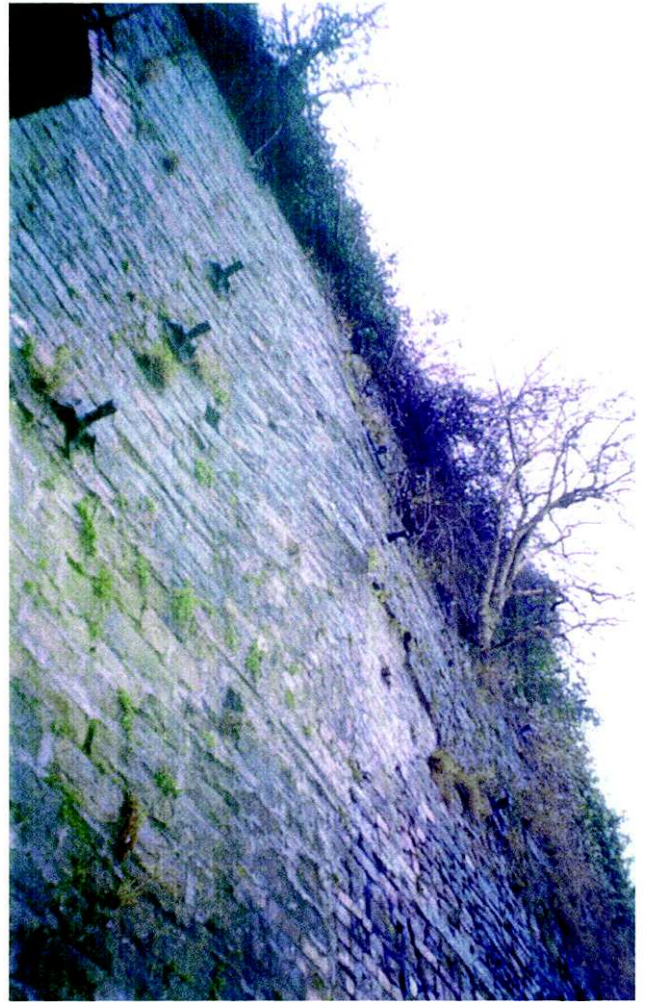
Plate 6: N.E. elevation of No.1 Furnace, showing tree and bulge in stonework.
