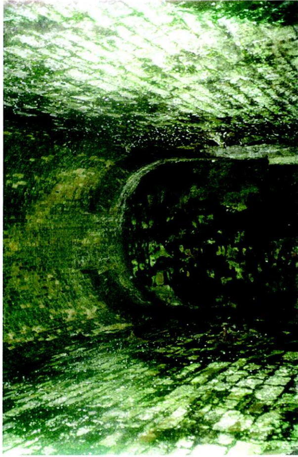
Plate 17: Inserted brick high vault between No.1 and No.2 Furnaces.
