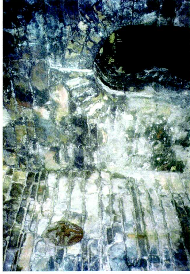
Plate 14: No. 1 Furnace - inserted wall and opening at S.E. end of upper gallery.
