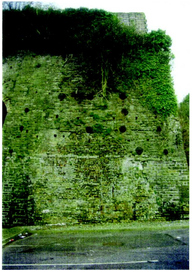
Plate 8: N.E. elevation of No.1 Furnace, showing bricked-up tapping vault.
