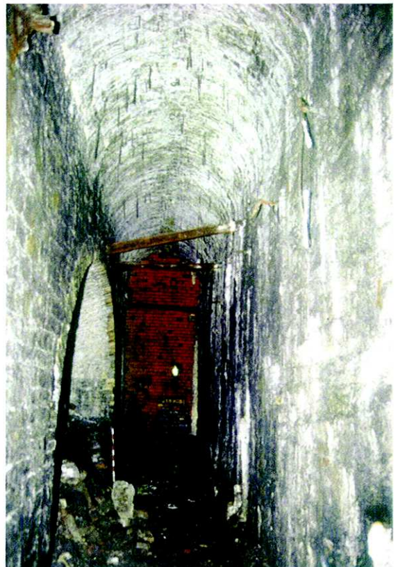
Plate 29: No.4 Furnace - lower gallery, showing rails from which blast main is thought to have been suspended.
