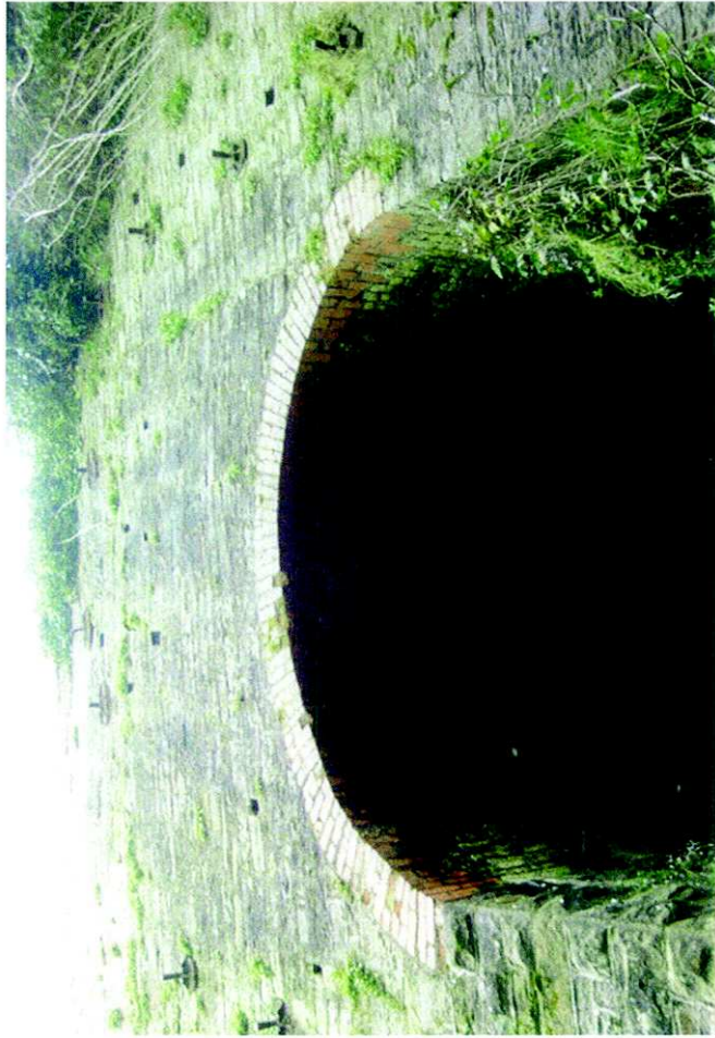
Plate 21: High vault between No.2 Furnace (right) and No.3 Furnace (left). Note structural joint on right side only.
