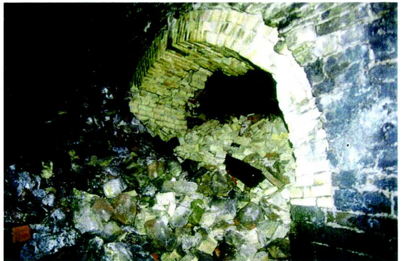
Plate 11: Collapsed S.W. blowing vault of No.1 Furnace.
