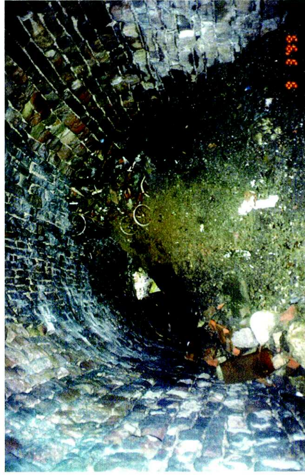
Plate 15: No. 1 Furnace - Collapse in crown of upper gallery.
