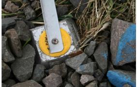
Now look at the bubble above the screen. By adjusting the height of the legs, one at a time, get the bubble roughly in the middle of the spirit level. Have a look at the laser, you may need to twist the wheels again as the laser plummet can move off the nail.
