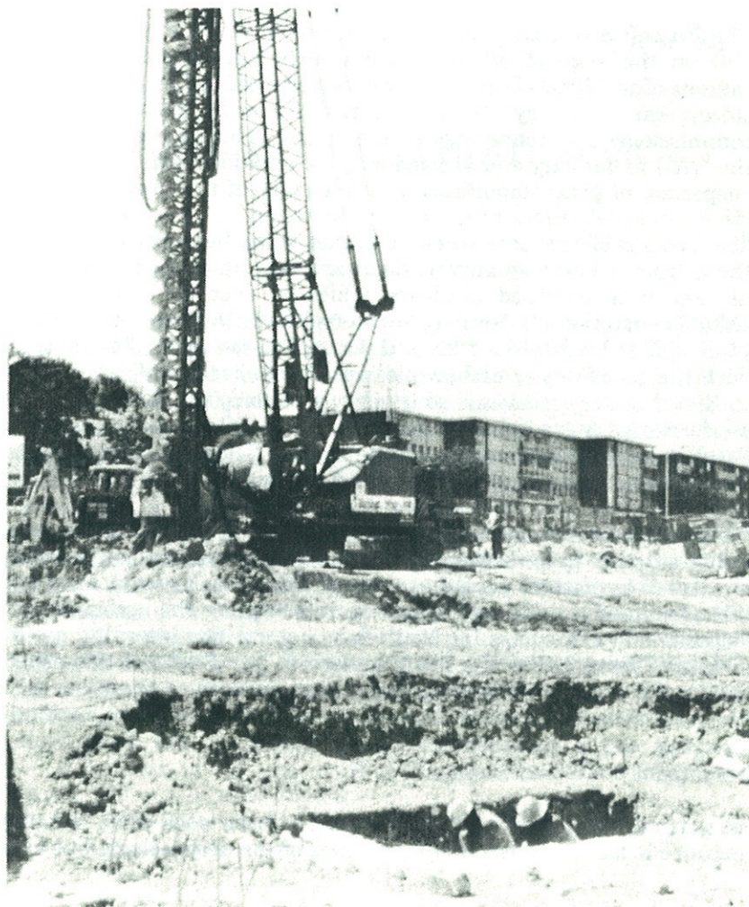
Figure 2: Dover 1989, the Heritage Centre site. Excavation for a lift shaft: the massive piling rig stands in the background (see Newsletter xvii (June 1989), 3-4 for details).
