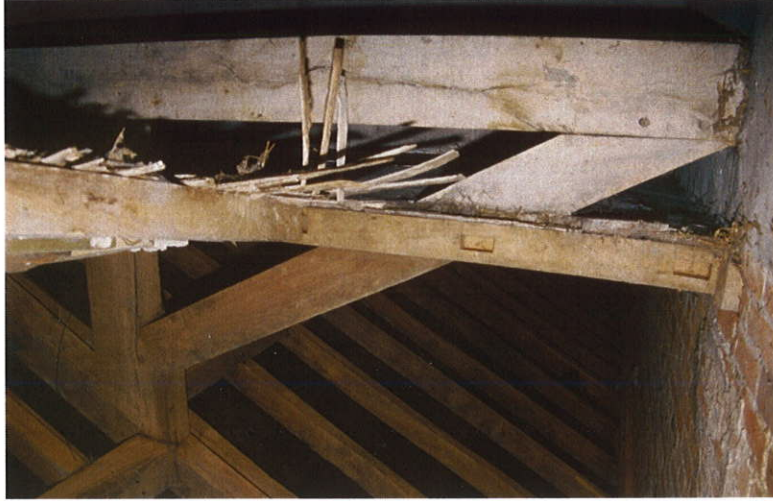
Plate 10: Roof truss above bothy with secondary ceiling abutting
