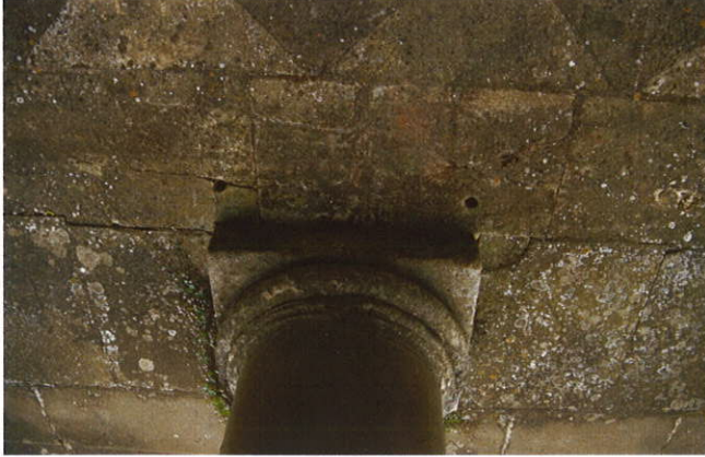
Plate 8: Small holes in floor which formerly held sash posts
