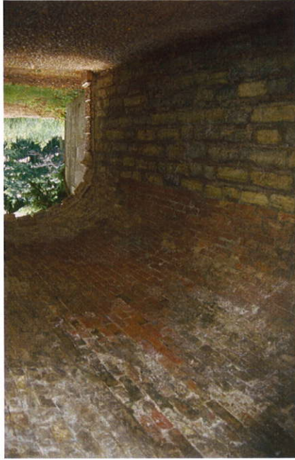
Plate 3: Interior of brick-vaulted tunnel
