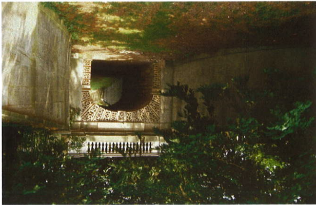
Plate 1 : Southern approach to tunnel showing retaining wing walls and portal
