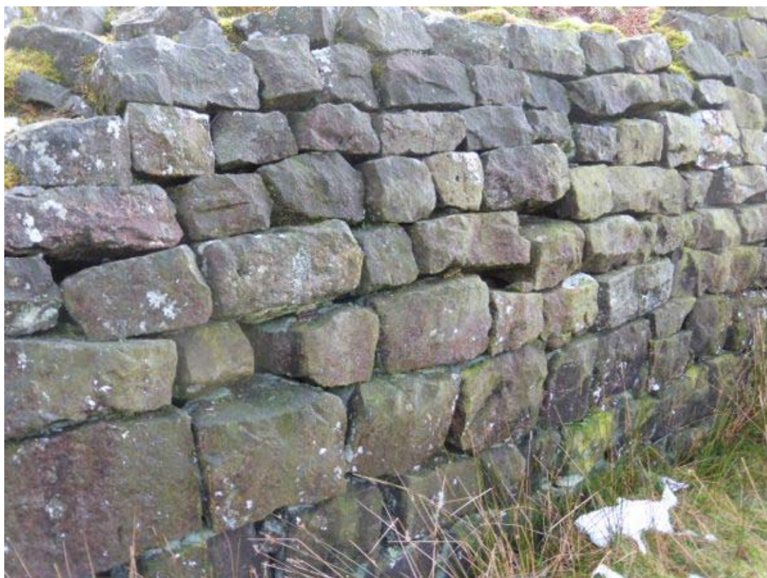
Plate 42: Dressing Floor – Bulging Wall – (East Side)
