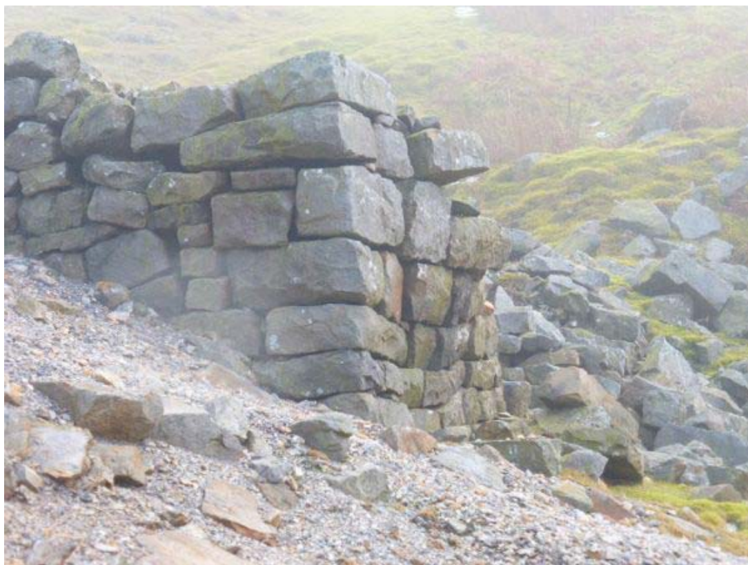
Plate 44: Dressing Floor – Collapsing part of North Wall
