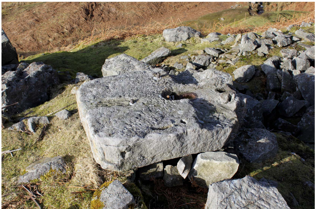
Plate 24: Bearing mount for a drive train leading to the Site 18.2 pit
