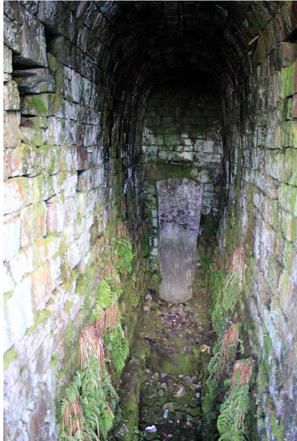
Plate 15: The tall barrel-vaulted interior of the portal with a wheel pit in the base
