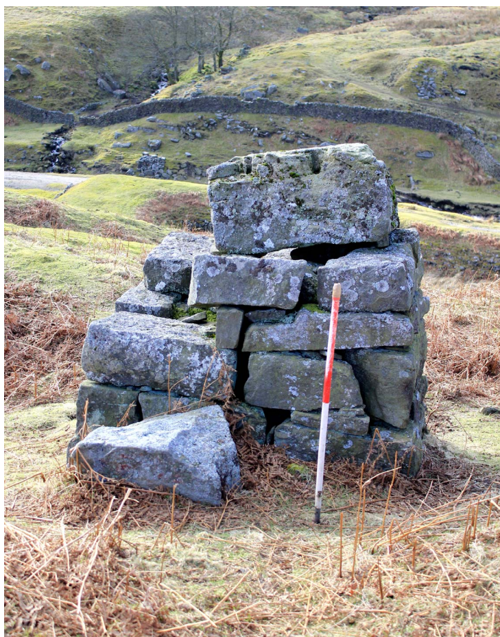
Plate 22: A square, stone plinth supporting the powered ropeway (Site 17.2 )
