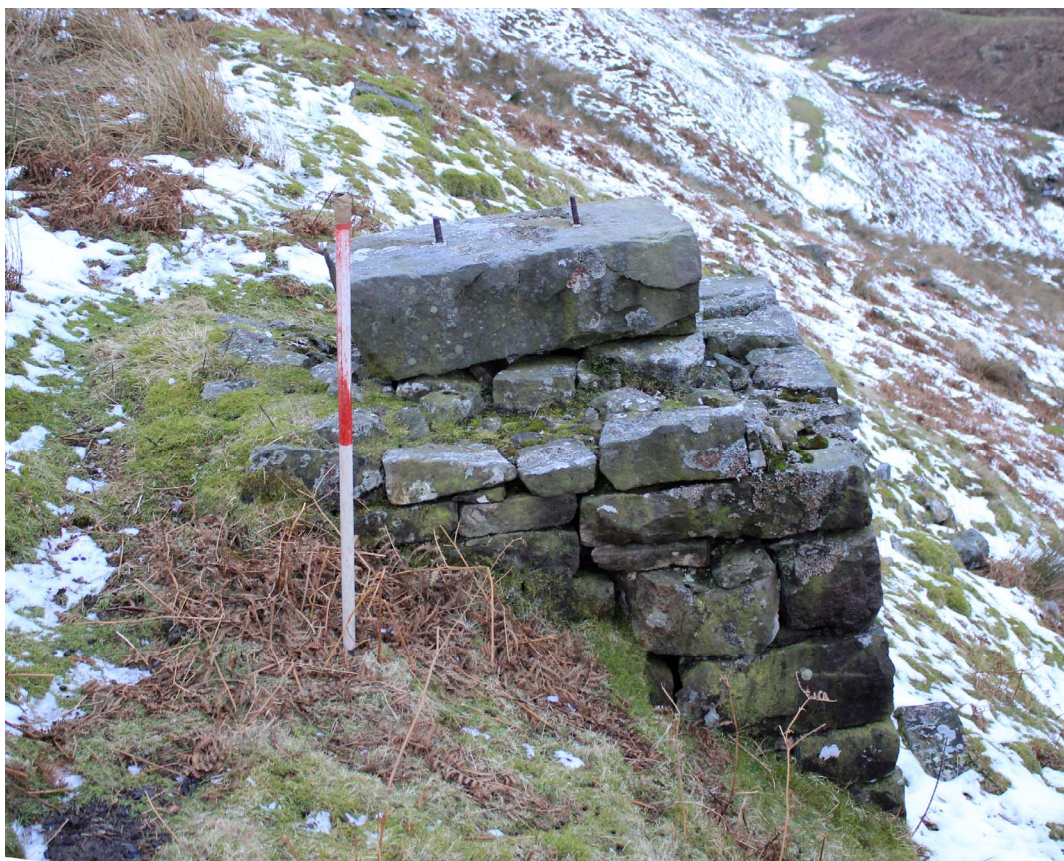
Plate 17: A stone pillar for the pump rods looking west with two bolts extending from a bearing mounting block (Site 7.3c)
