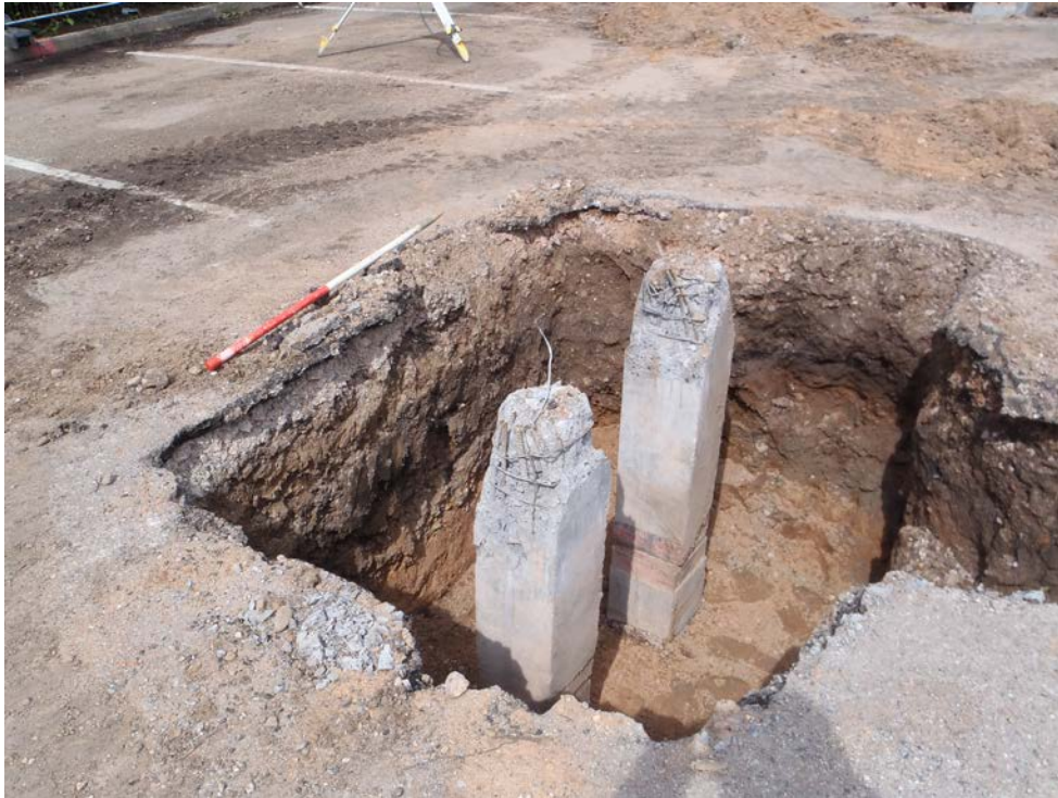
Plate 3: Oblique shot of east-facing section of pile trench A1
