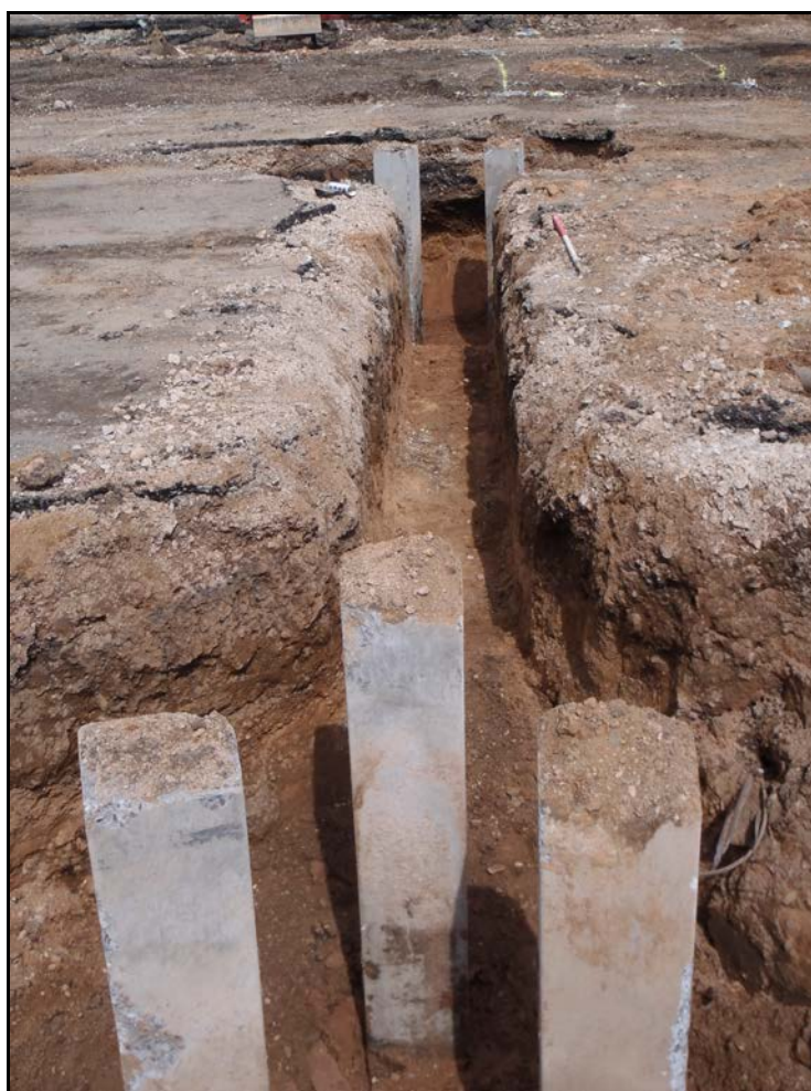
Plate 2: North-facing view of pile trench B3 to A3
