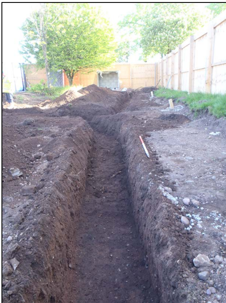
Plate 5: North-facing view of service trench situated to the north-east of site
