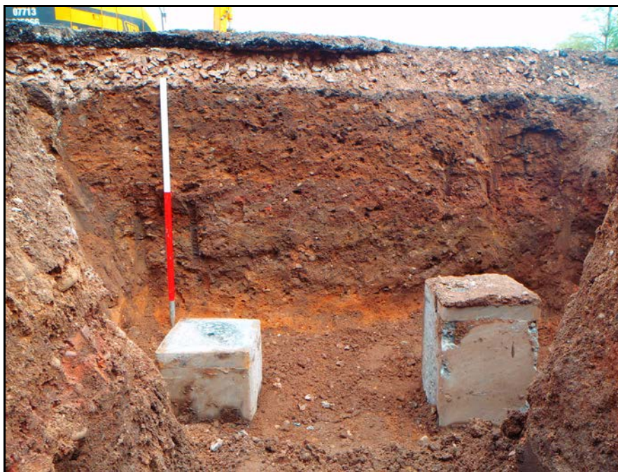
Plate 1: South-west-facing section of pile trench F3
