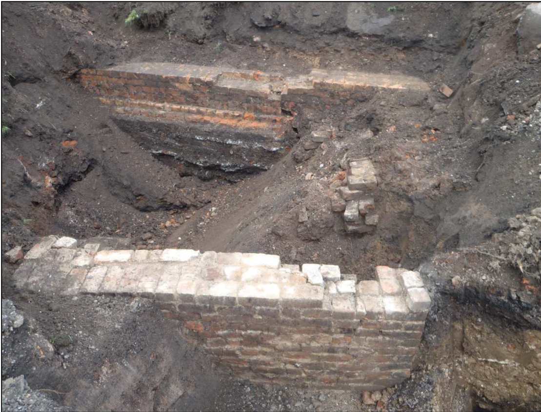
Plate 5: The walls of the possible pump house, looking north, with wall of later structure to the rear
