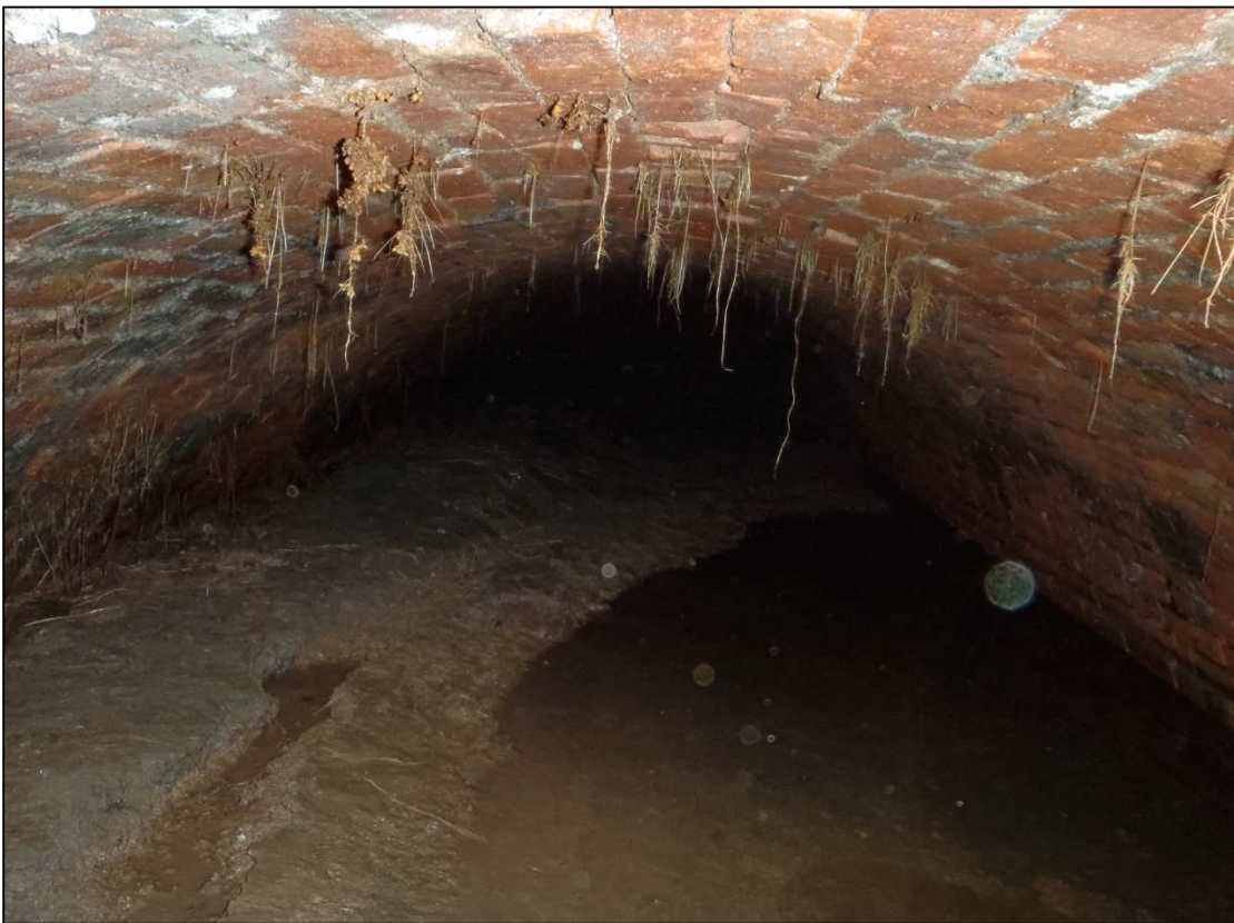
Plate 13: Culvert interior, looking north
