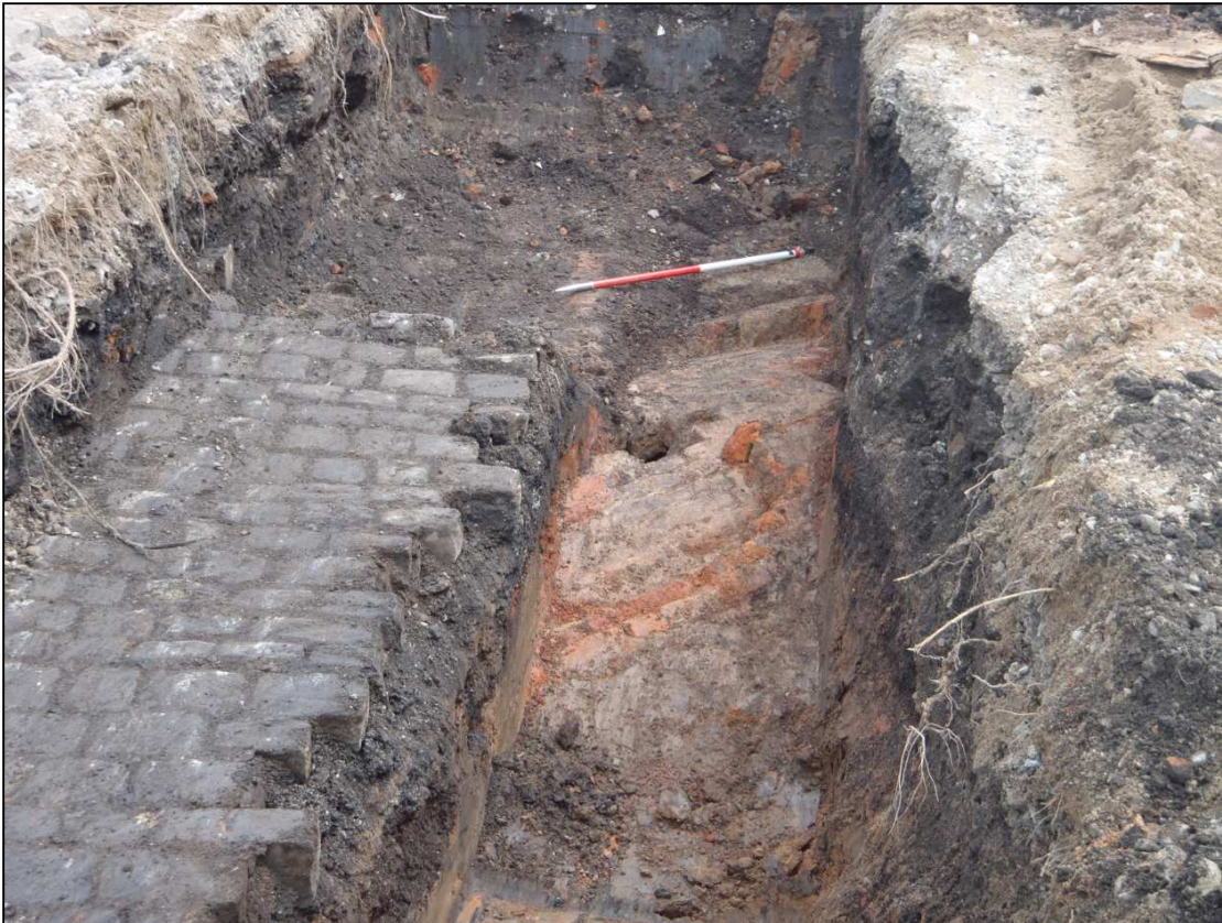
Plate 12: Brick culvert running below road surface, looking south-east
