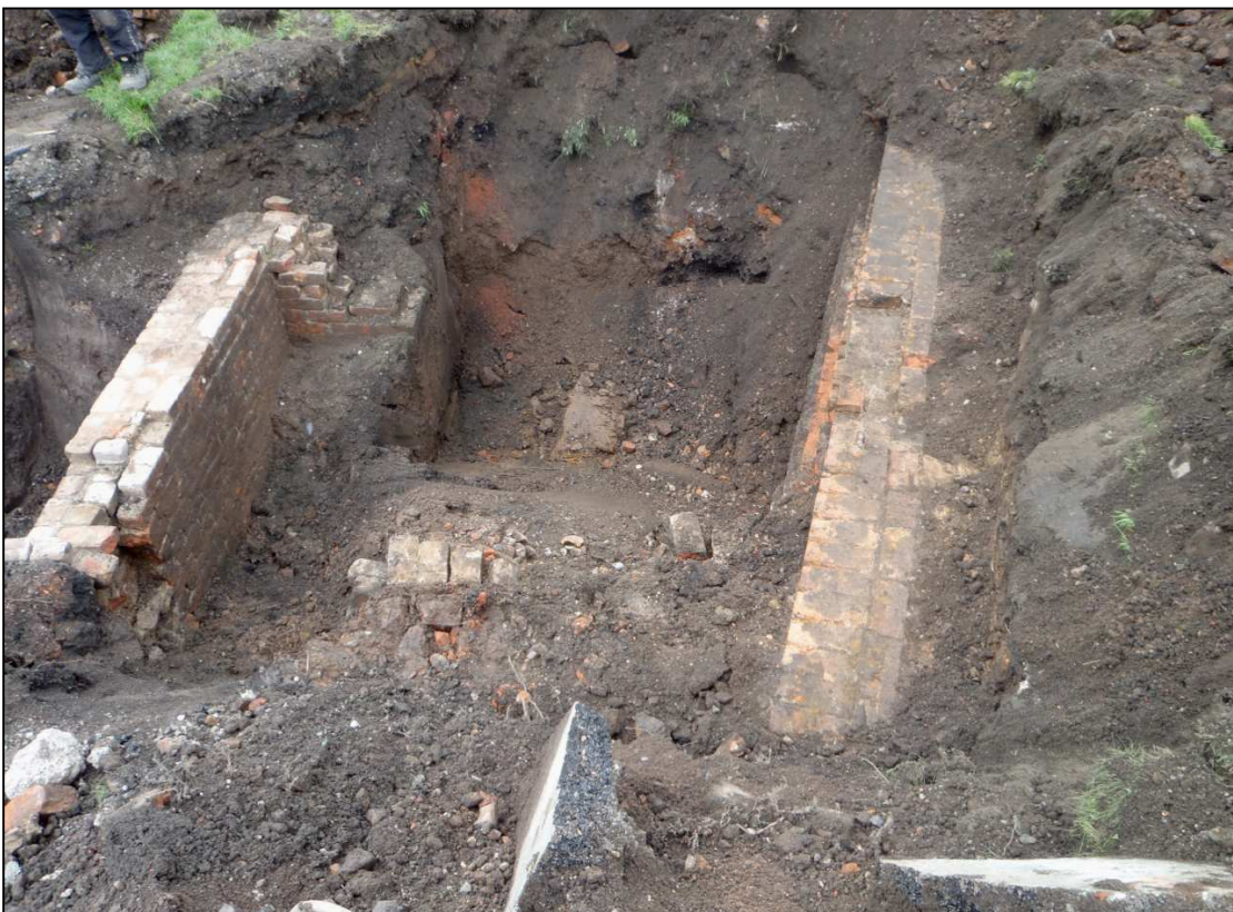
Plate 6: Pump house walling (left) and later wall (right), looking west
