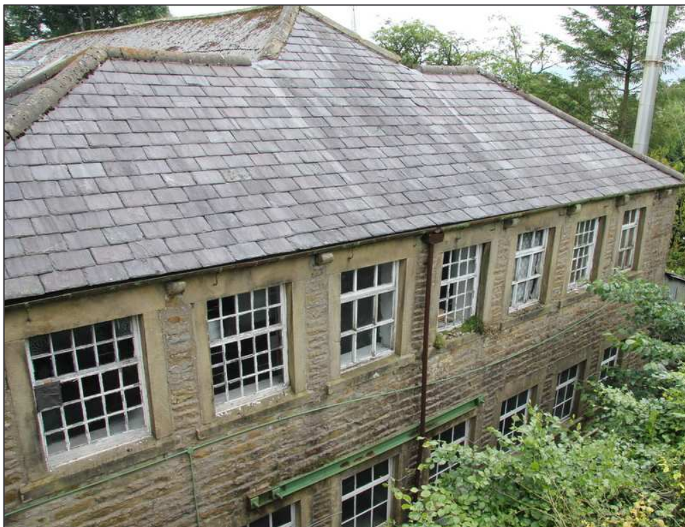
Plate 10: External west elevation of the west wing
