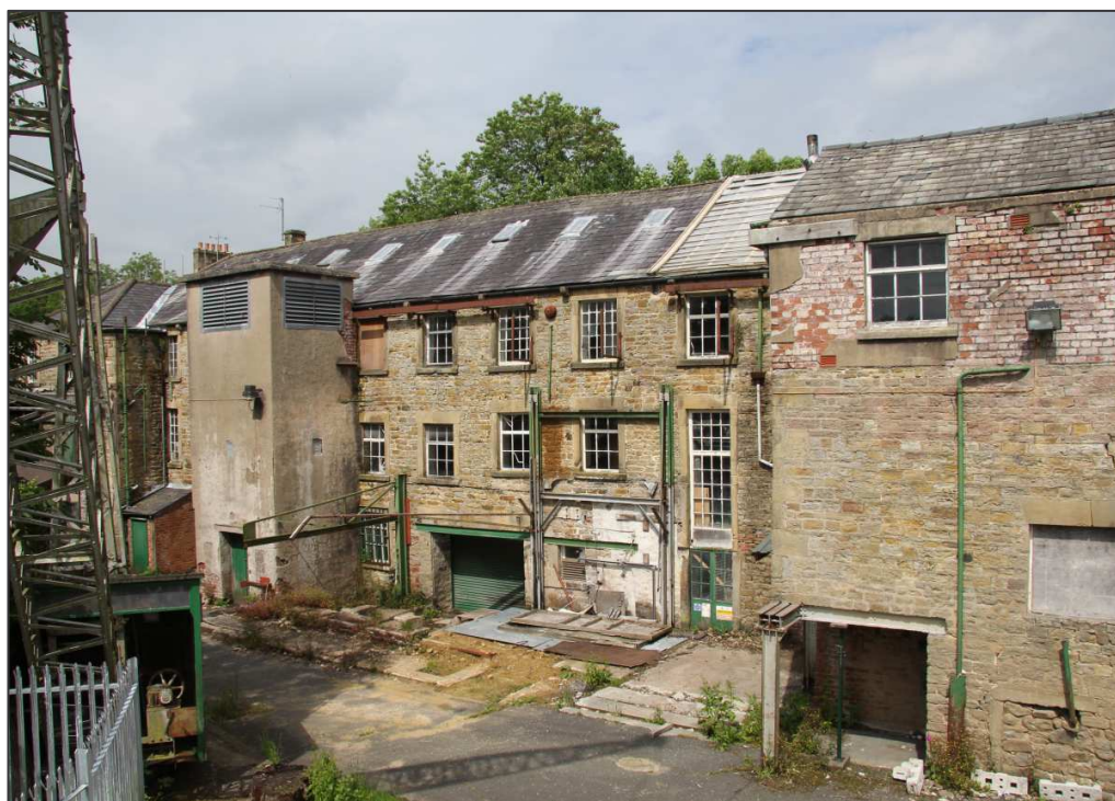
Plate 7: View of the southern elevation of Kirk Mill
