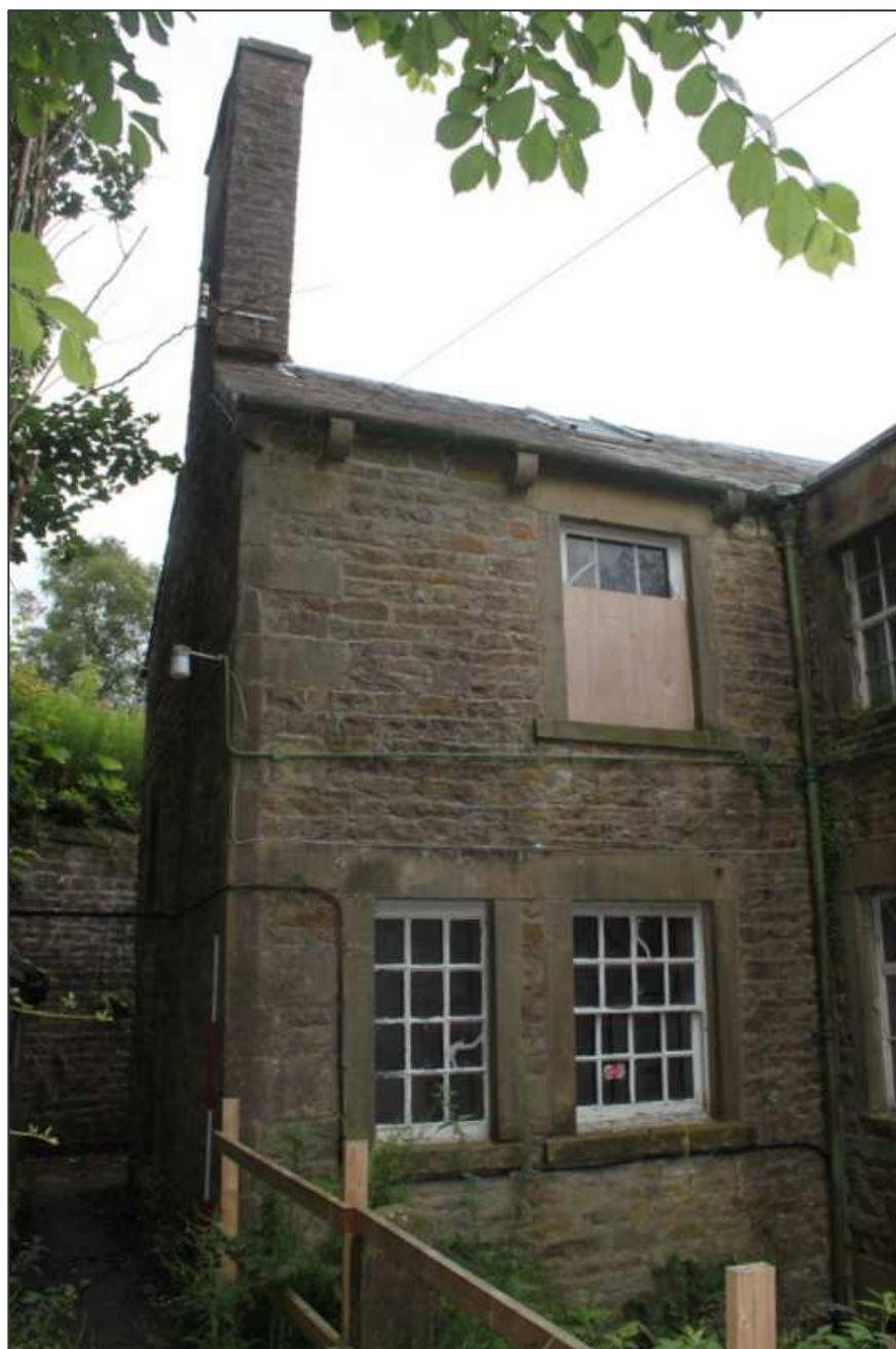
Plate 13: The west elevation of the tower, showing the bell cote
