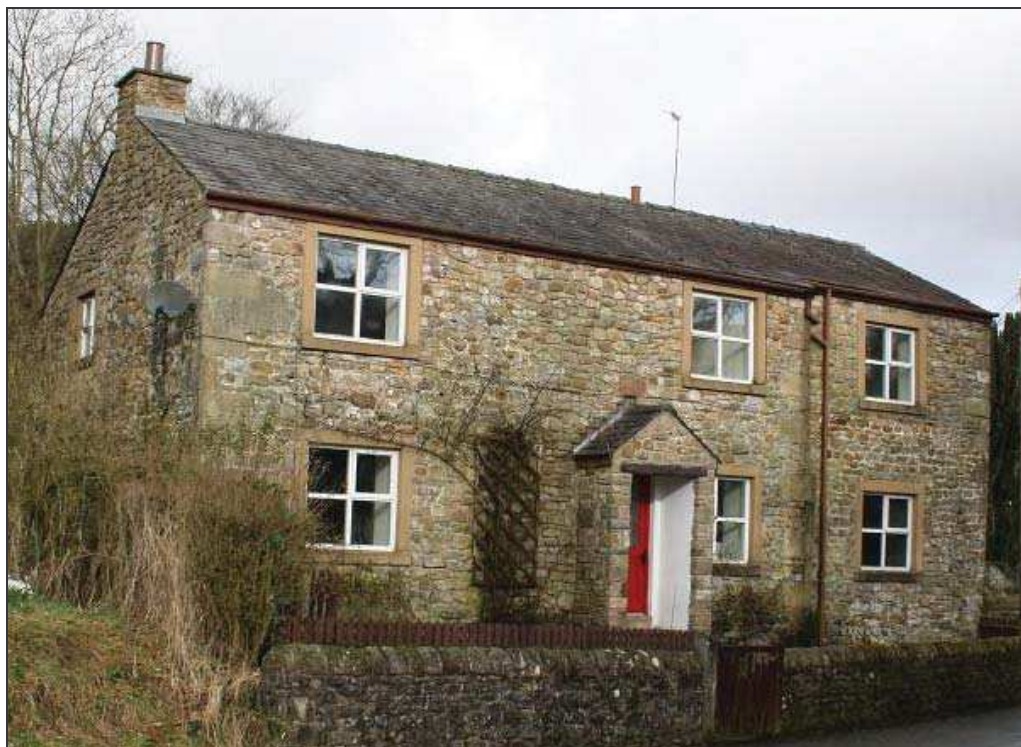
Plate 23: Malt Kiln House
