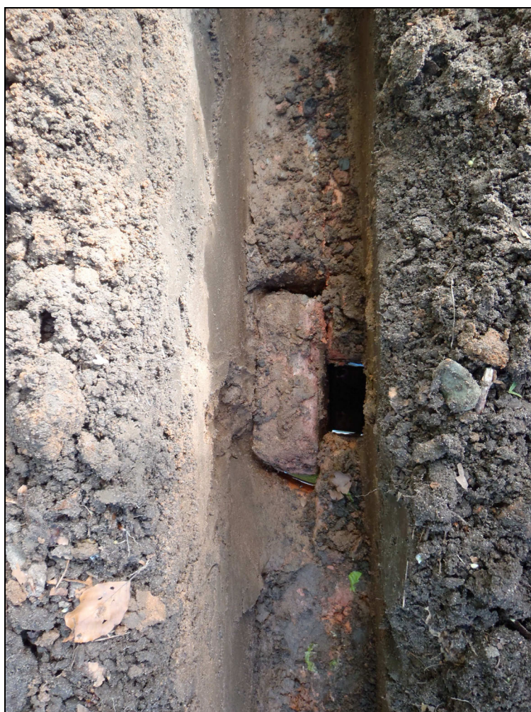
Plate 6: The brick-built drain
