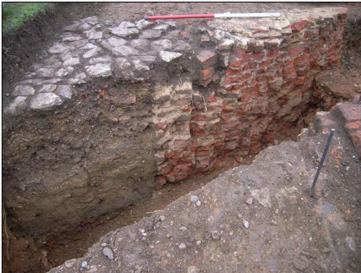
Plate 7: Trench 1, Section through foundations of the Gatehouse, context 115 and later ragstone cobble 120
