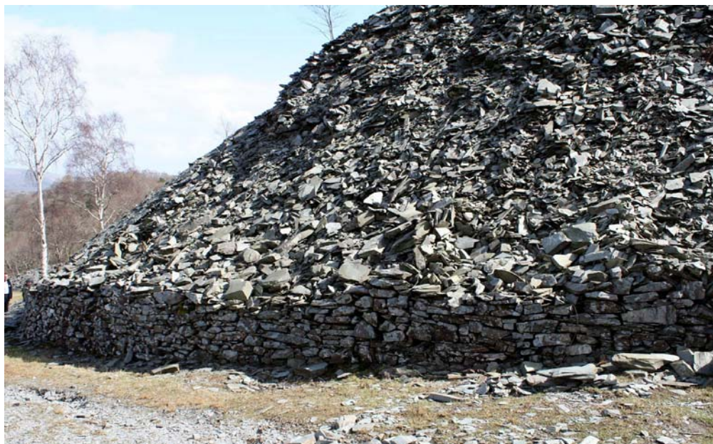
Plate 12: Retaining wall 105 around the base of a large spoil heap
