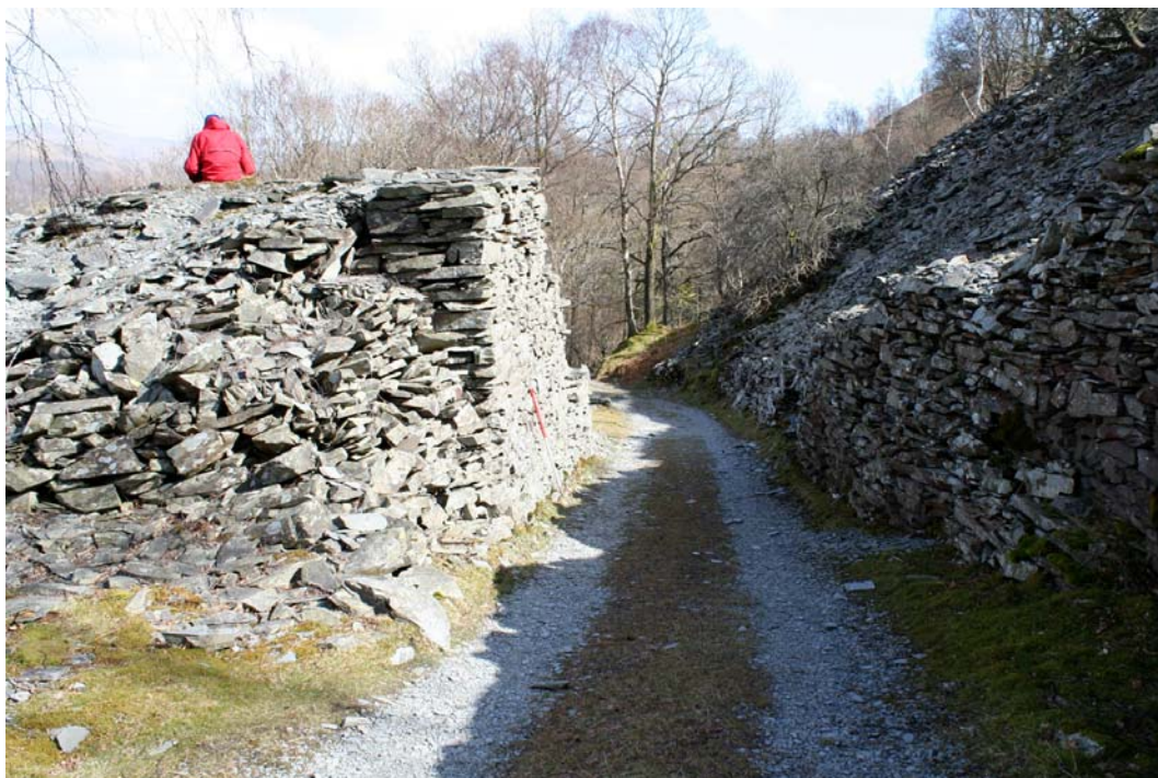
Plate 16: the bridge abutments ( 109 ) allowing the passage of spoil over the miners road
