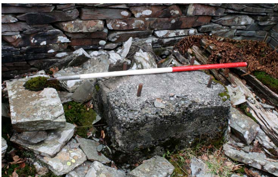
Plate 22: Engine mounting block inside engine shed 103a
