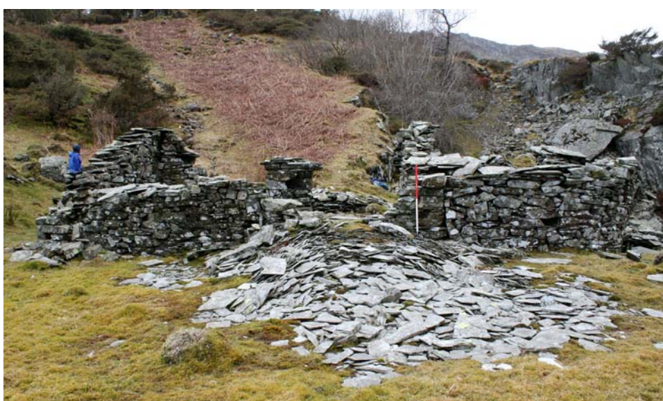
Plate 19: Riving shed 100a with a large pile of riving waste outside the window
