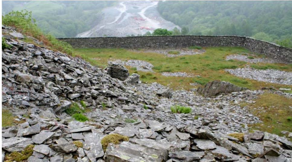
Plate 15: the enclosure wall constructed over the top of a spoil heap, which is now in a good condition without gaps
