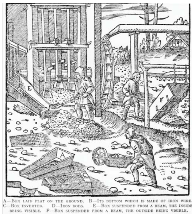
Plate 26: Example of a dry stamp mill (Agricola 1556, 287)
