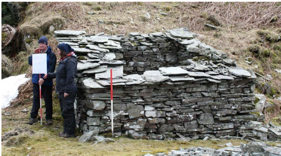
Plate 6: Square store shed (Site 01b ) with remnants of the slate roof surviving
