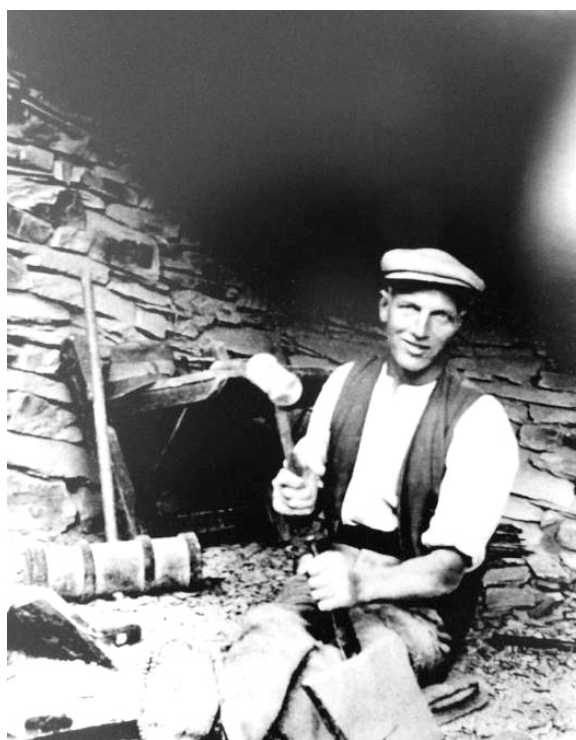
Plate 3: Mr Bowness riving slate in a shed at Banks Quarry probably prior to the First World War
