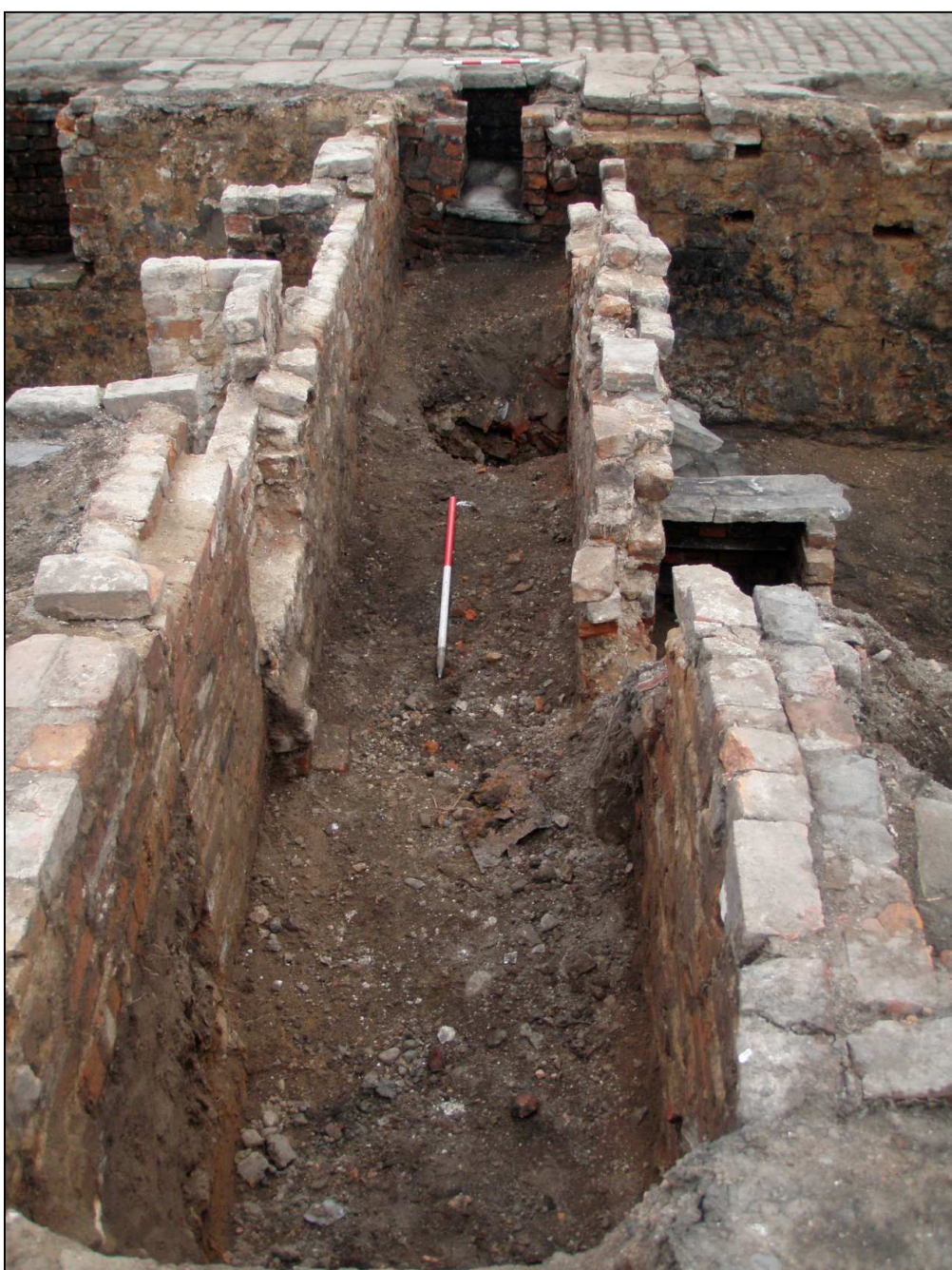
Plate 52: Passage G4, looking south-east
