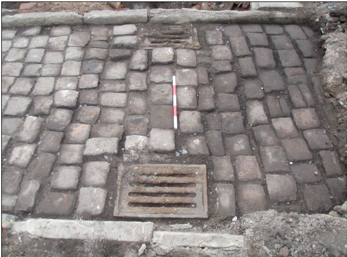
Plate 11: Drain covers set into Lawson Street
