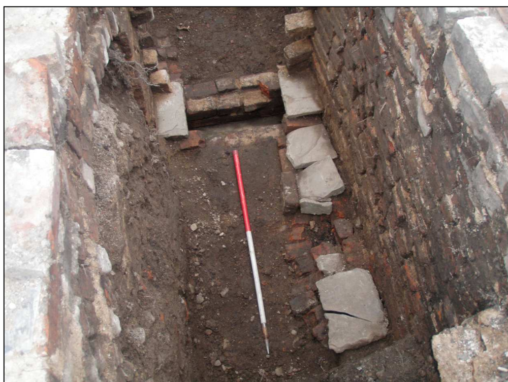
Plate 35: Stone-capped drain in passage G1, looking south-east
