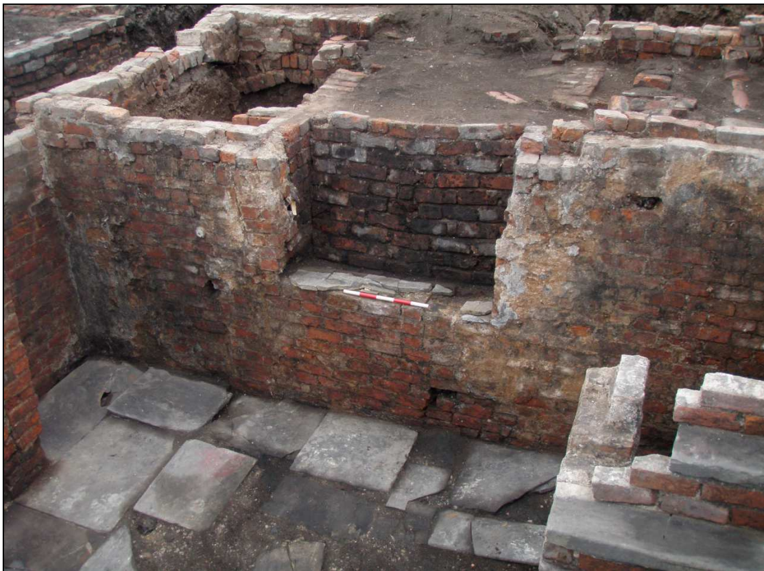
Plate 45: Cellar light window in Cellar H3, looking north-west
