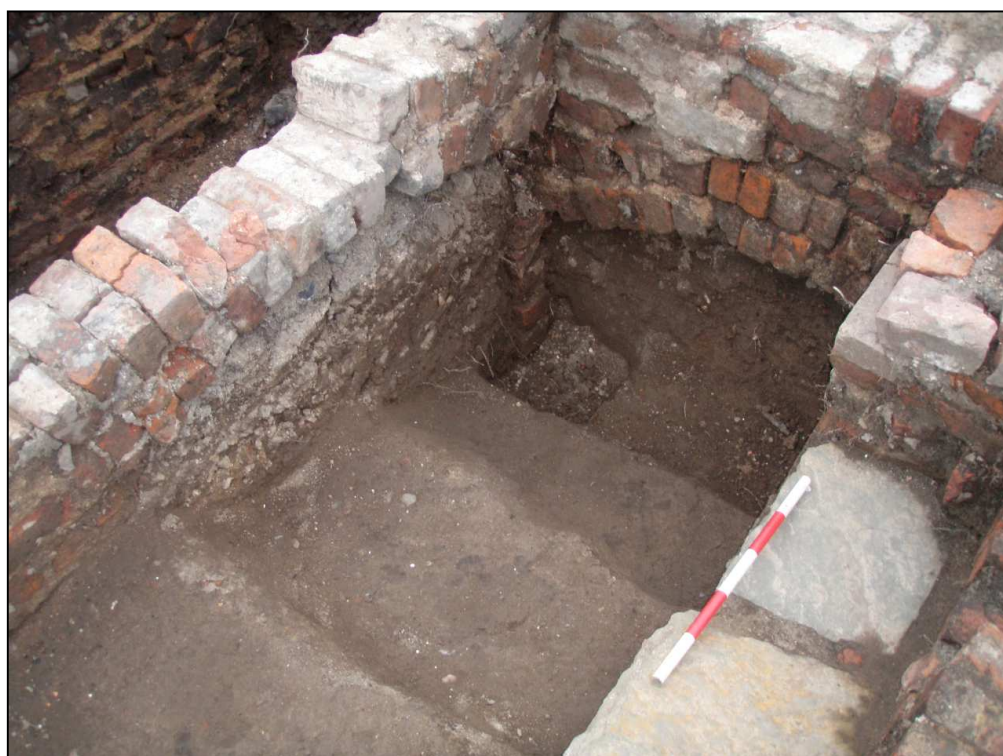
Plate 46: Arches in south-western rear room in Cellar H3, looking west
