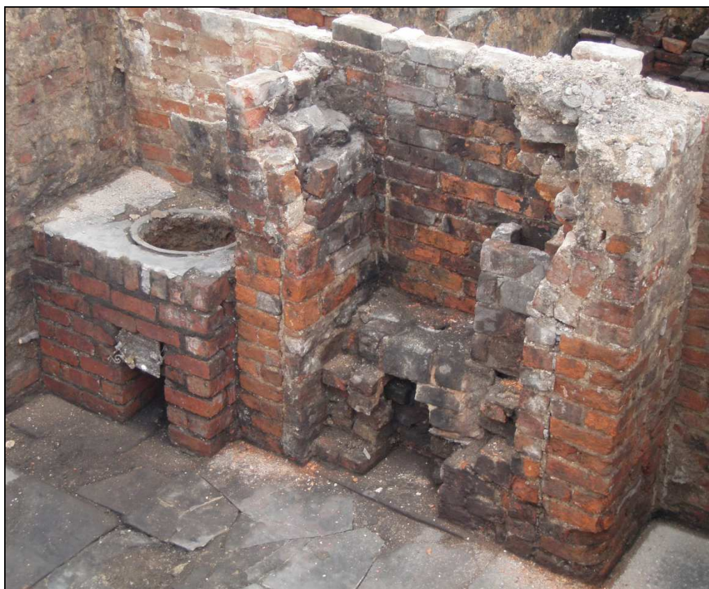
Plate 30: 'Set-pot' boiler in Cellar H3
